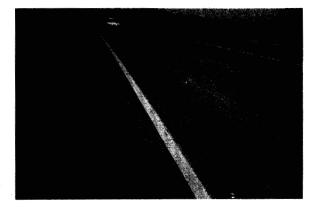
Micro-surfacing has been used to repair OGFCs and raveled surfaces with considerable sucess. This slide shows a 3 years old micro-surfacing project placed on top of a raveled OGFC project in Oklahoma
