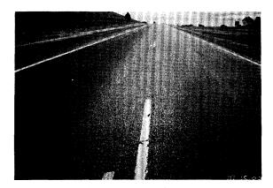
This is a 5-years-old micro-surfacing project on I-40 in Oklahoma. This project involved both rut filling and texturing. With the exception of minor wheel consolidation and cracking, the surface is in good condition.
