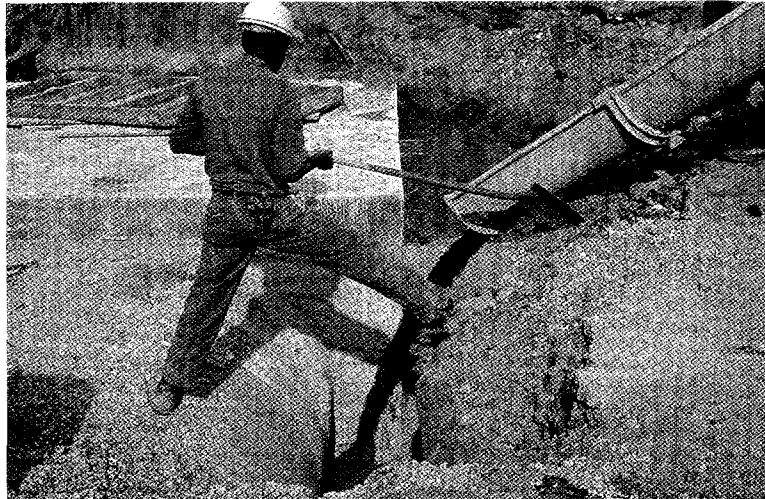
Figure 15. Flowable fill eliminates the need for workers to enter the trench to compact.
