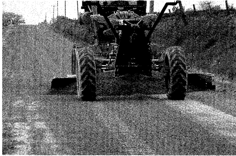
Figure 13. Achieving final grade with a motor grader before final compaction.
