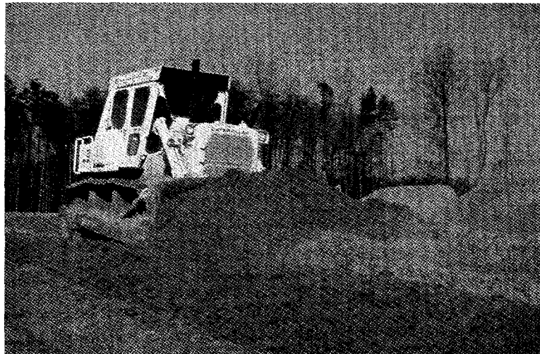
Figure 22. Spreading fly ash structural fill.
