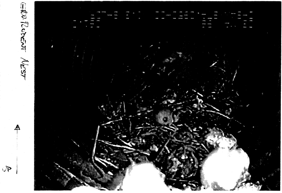
Figure 20. Rodent's Nests Found Blocking the Mainline at 61.0 Feet.
