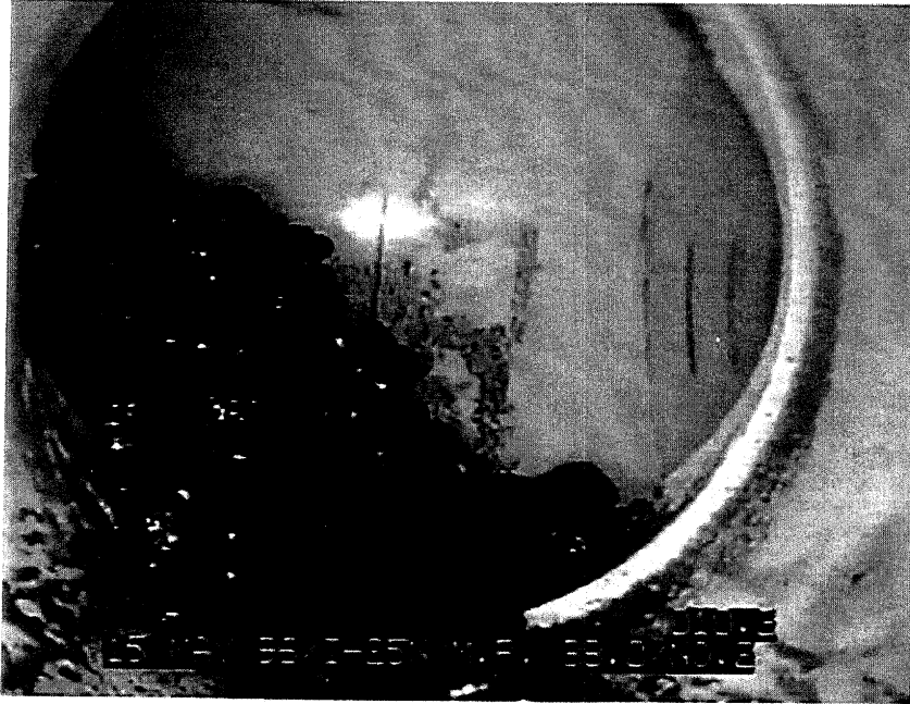
Figure 16. Asphalt-Stabilized Base in Edgedrain.
