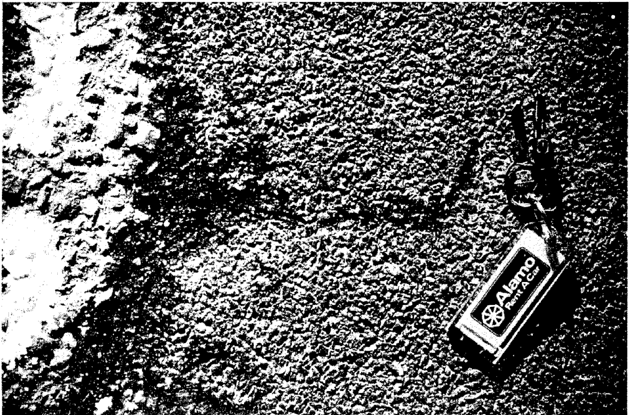
Figure 32. Example of cracking distress.
