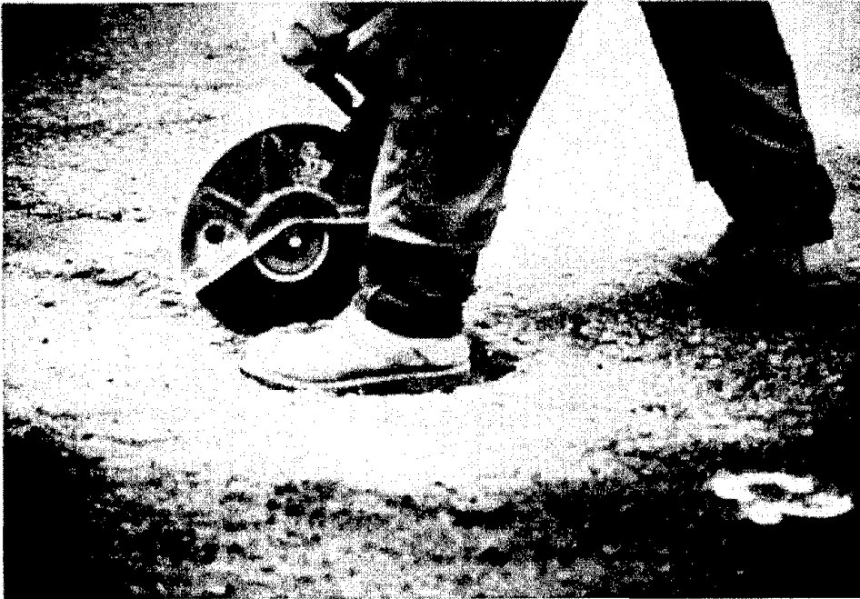
Figure 15. Straightening sides using pavement saw.
