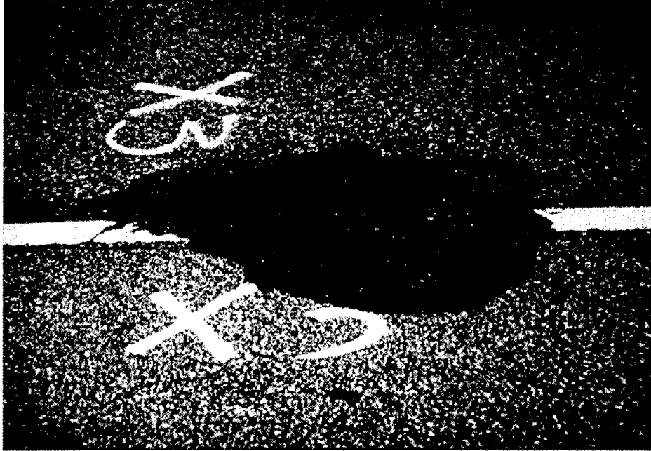
Figure 31. Example of shoving distress.
