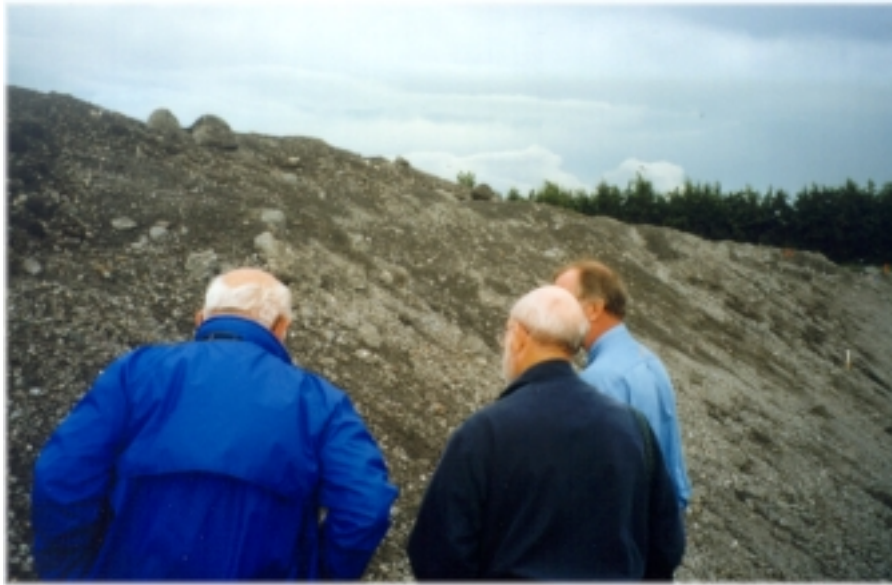
Figure 20. WTE bottom ash use in a road embankment in the Netherlands. The embankment will be about 3 meters high.
