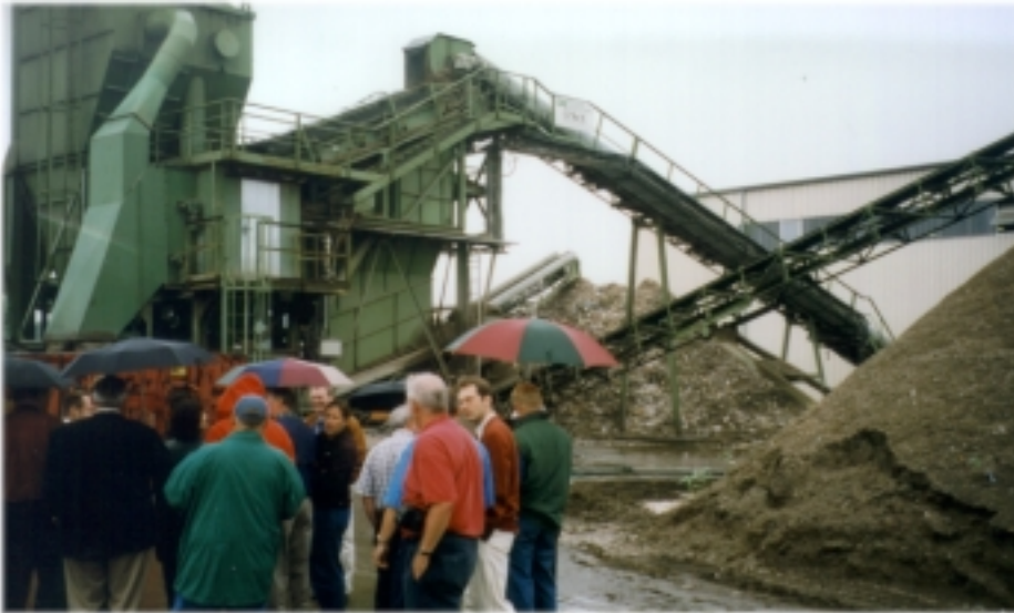
Figure 17. Aggregate crushing and sorting facilities at the Remex C&D processing plant. The pile in the foreground is aggregate made from crushed C&D waste. It will be used in highway base course.
