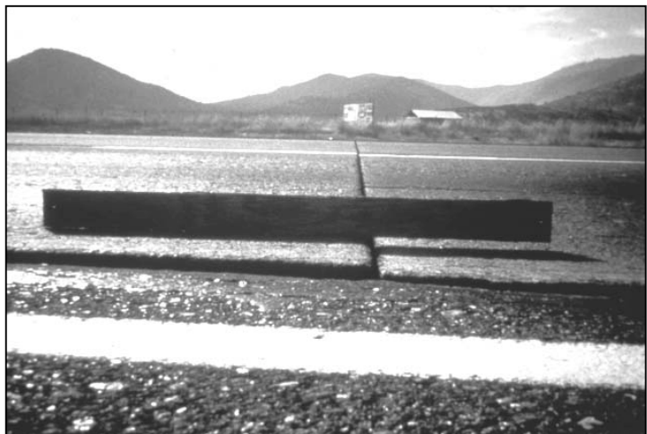
Figure 1. Diamond grinding can be used to correct surface irregularities such as faulting (difference in elevation across a joint or crack).
