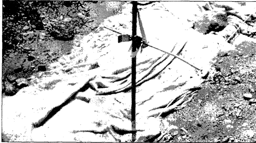
Photo No. 3 String Control for line and Grade
