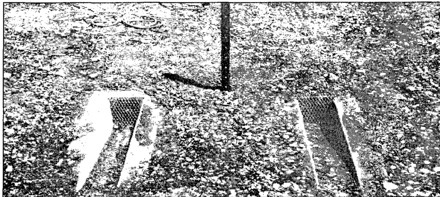
Photo No. 9 Dual Pipe Outlets
