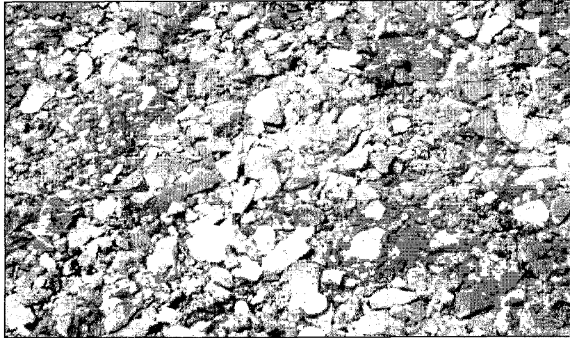
Photo No 4. Completed Unstabilized Permeable Base
