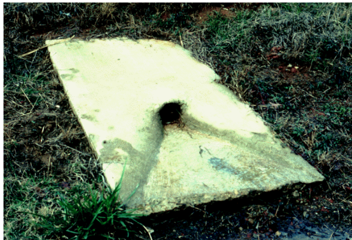
Photo No. 8 Large Outlet Pipe Headwall
