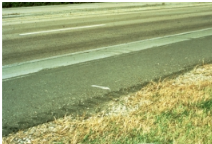
Photo No. 6 Painted Arrow as a Reference Marker
