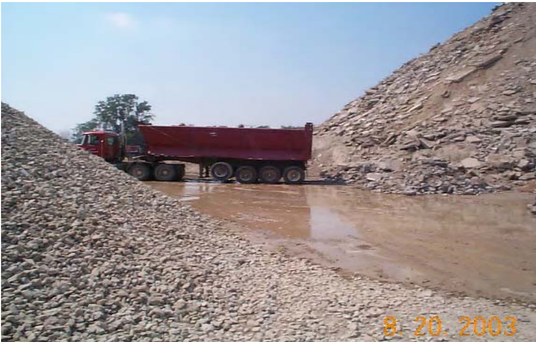
Figure 6. Truck preparing to unload concrete debris Iafate Crushing Plant Visit. Taylor, MI.
