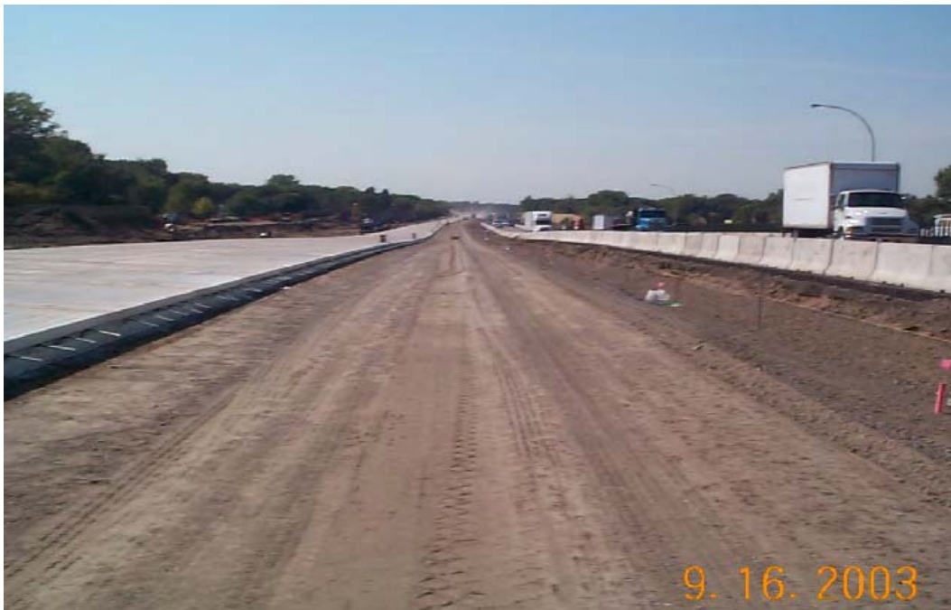
Figure 19. Recycled concrete aggregate. I-694 Reconstruction Project Visit. Brooklyn Center, MN
