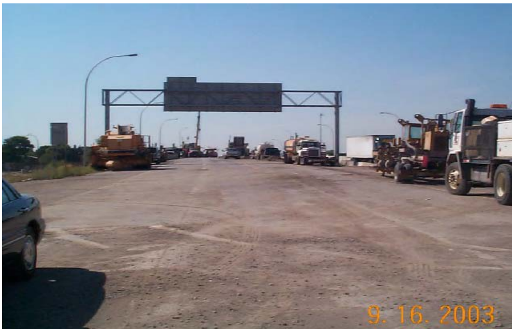
Figure 16 I-694 Reconstruction Project Visit. Brooklyn Center, MN.
