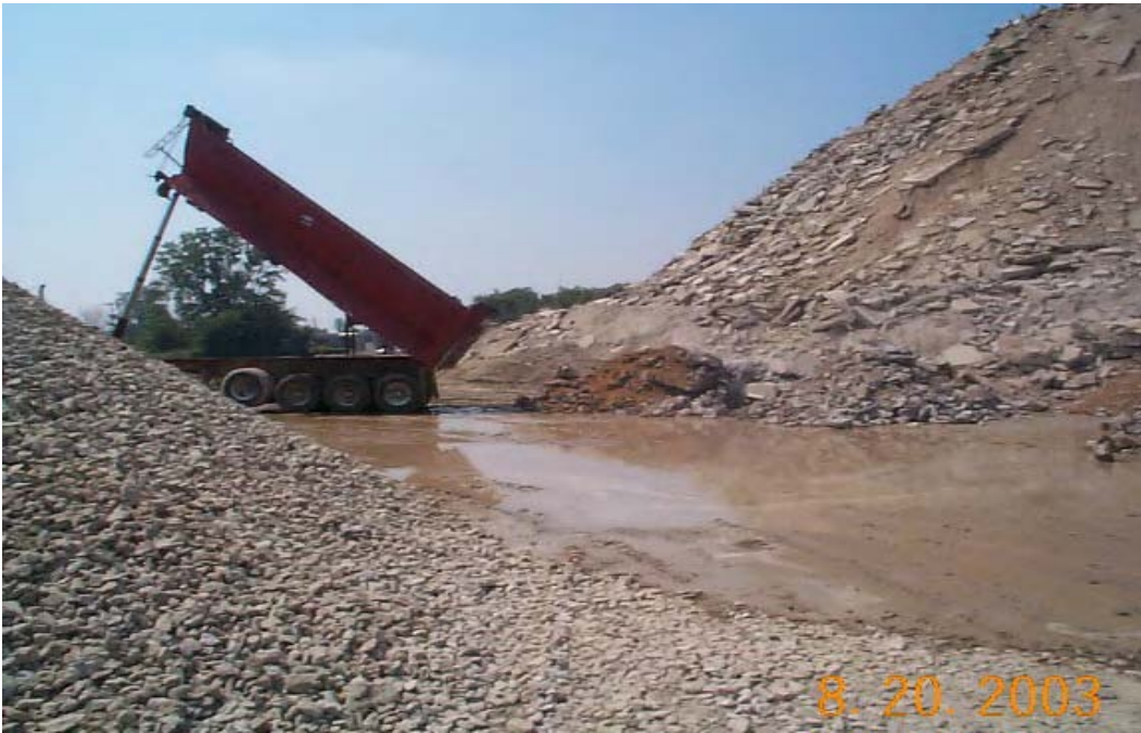
Figure 7. Truck unloading concrete debris. Iafate Crushing Plant Visit. Taylor, MI
