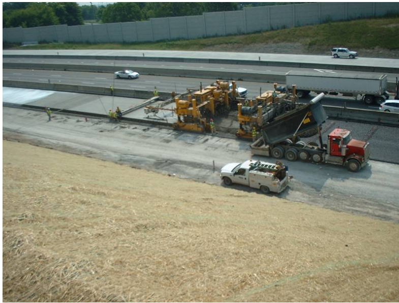
Figure 5. General view of concrete pavement construction on northbound I-65.
