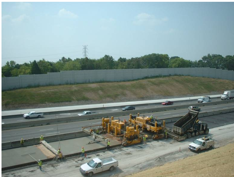
Figure 6. General view of concrete pavement construction on northbound I-65.
