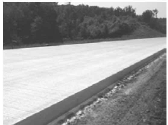
Figure 1. Properly applied curing compound.
