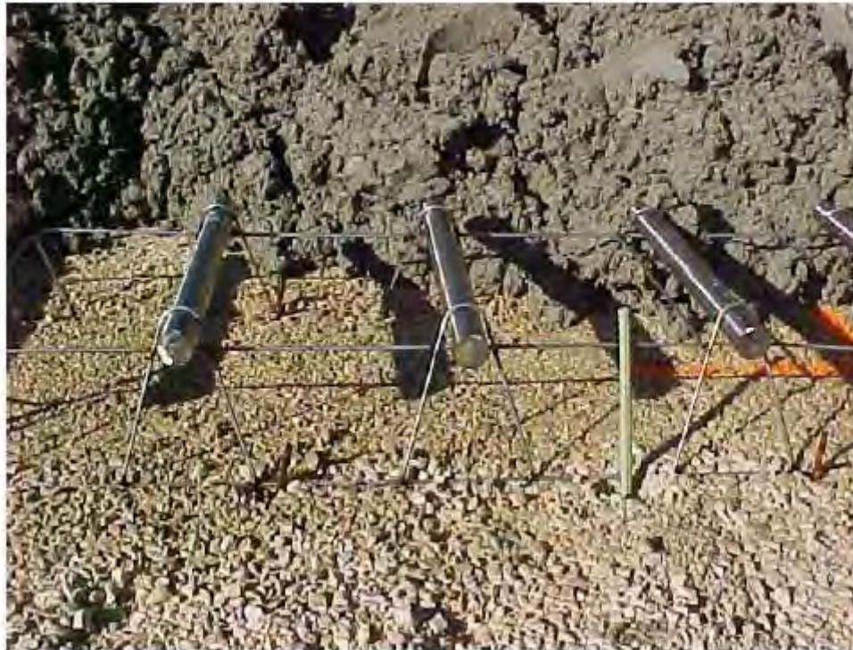
Figure 108. Stainless steel dowels and basket on WI 4 (Kemp 2004).
