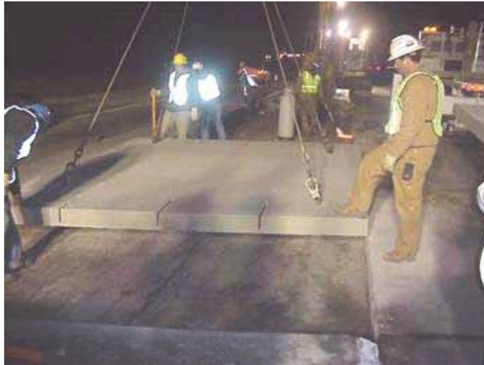
Figure 4. Precast panel installation in Colorado.
