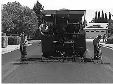
Pavement preservation treatments for asphalt pavements can include slurry seals, which are shown here.
