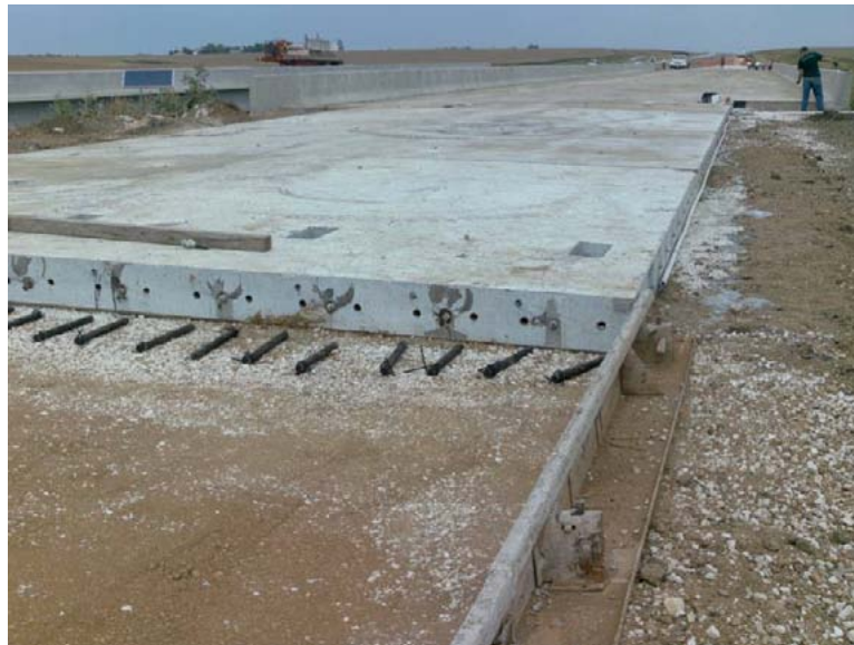
Figure 38. Photo. Dowels for the EF expansion joint prior to its installation in the precast panels (photo by Iowa State University, reprinted by permission).
