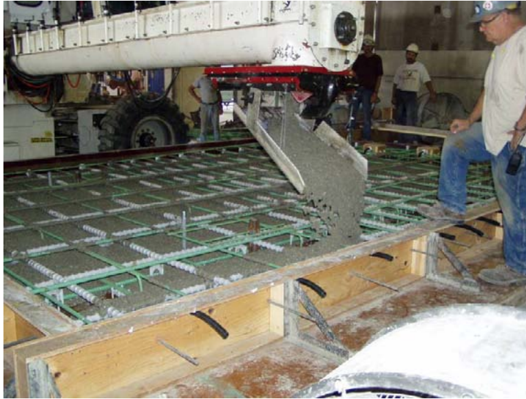
Figure 18. Photo. Placement of concrete for an abutment panel.
