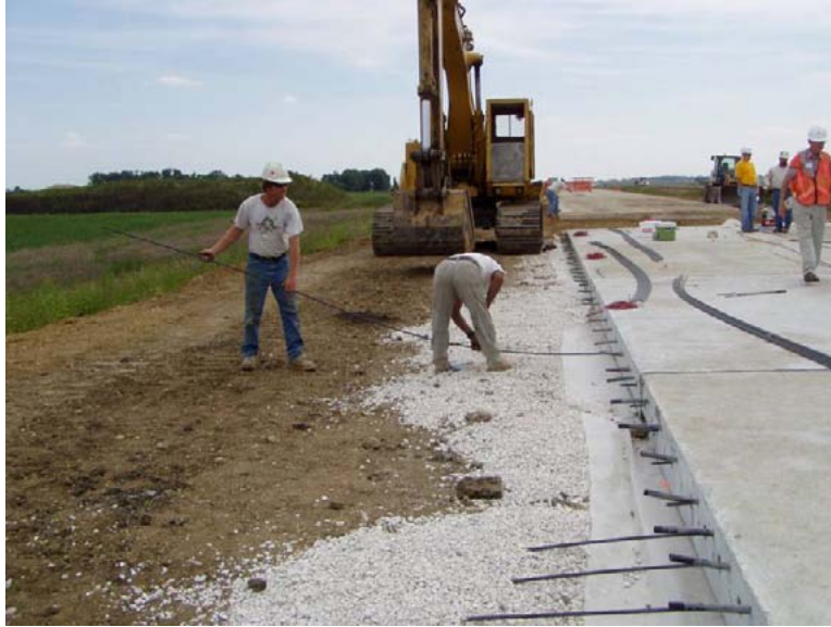
Figure 33. Photo. Inserting the transverse strands into the approach slab.
