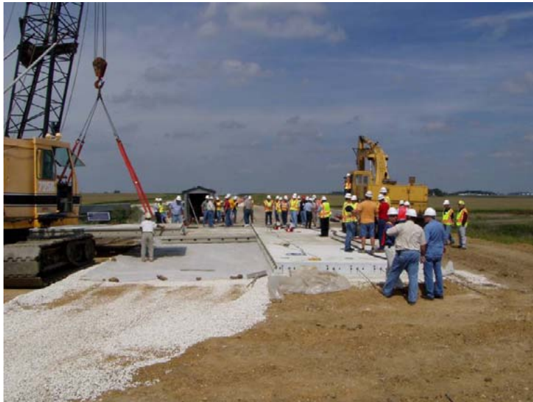
Figure 45. Photo. Site visit during installation of the precast approach slab.
