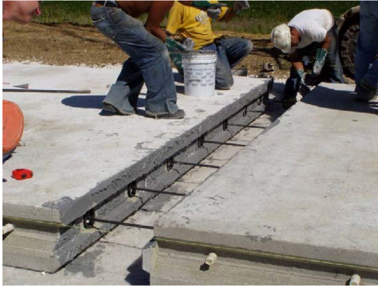
Figure 30. Photo. Application of joint epoxy during panel installation.
