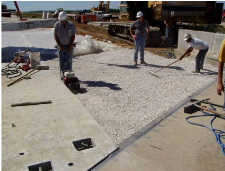
Figure 27. Photo. Grading and compaction of the aggregate base material.
