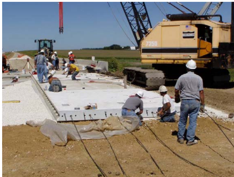
Figure 32. Photo. Inserting the longitudinal strands into the approach slab.
