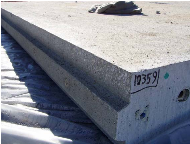
Figure 26. Photo. Keyway after completion of grinding.
