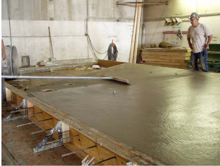
Figure 19. Photo. Application of the light broom texture to the panel surface.
