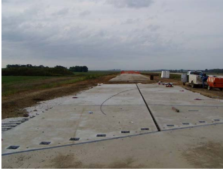
Figure 29. Photo. Finished approach slab prior to final post-tensioning.
