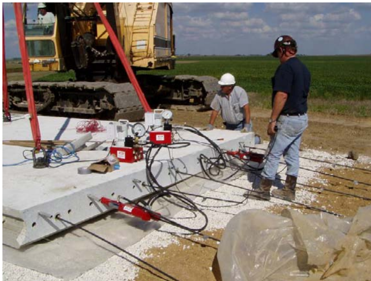
Figure 31. Photo. Temporary post-tensioning used to pull panels together.
