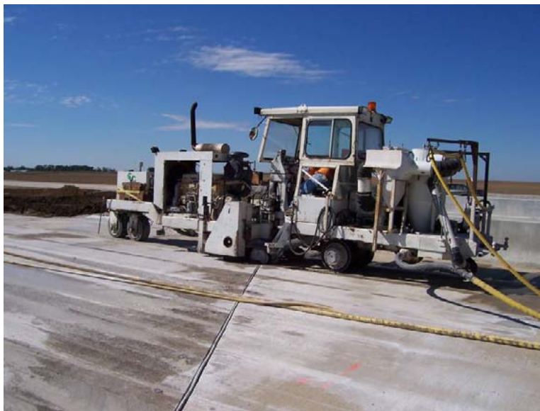
Figure 39. Photo. Diamond grinding the south approach slab.
