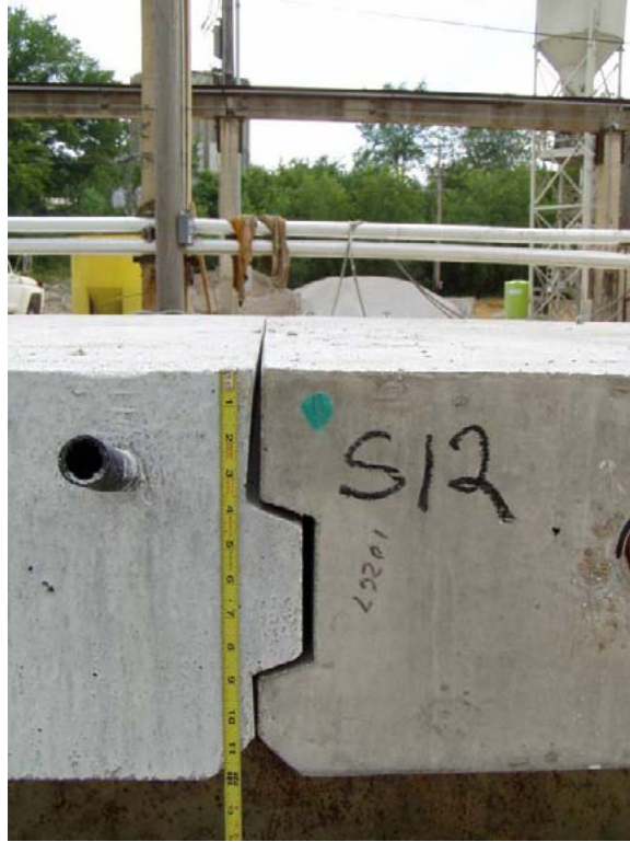
Figure 25. Photo. Battered keyway after removal from forms.
