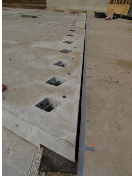
Figure 40. Photo. Joint between south approach slab and bridge abutment.
