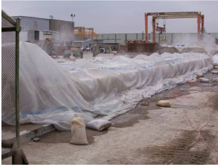
Figure 24. Photo. Casting bed during steam curing operation.
