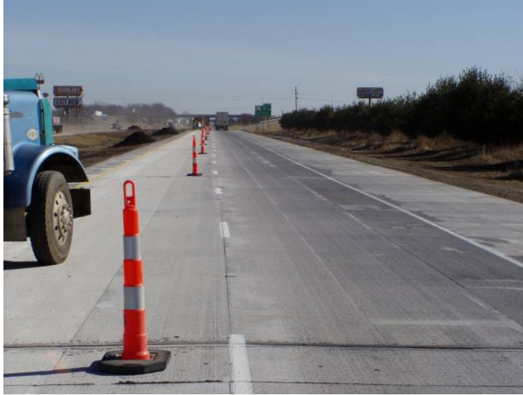
Figure 45. Photo. Final pavement surface after diamond grinding.
