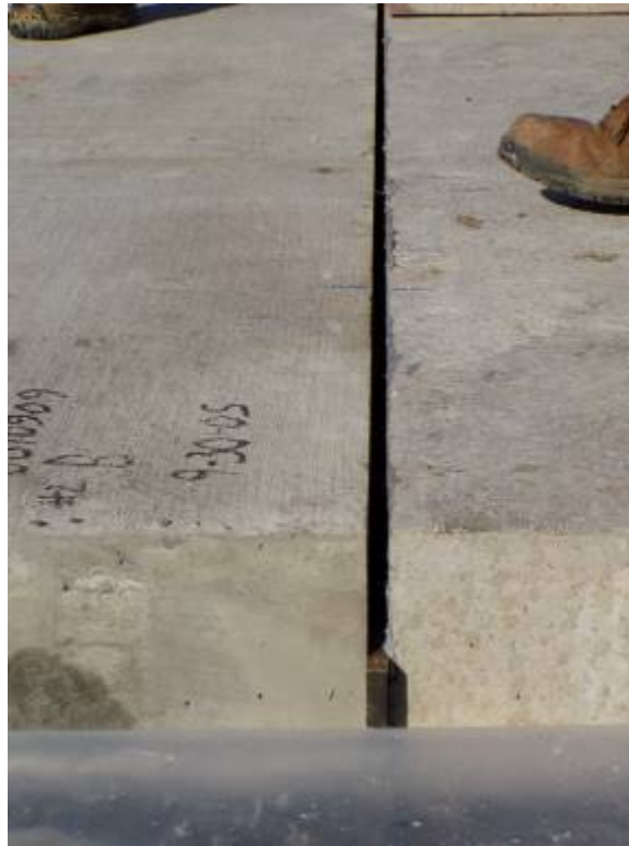
Figure 47. Photo. Shims at the outside edge of the pavement used to correct centerline alignment.
