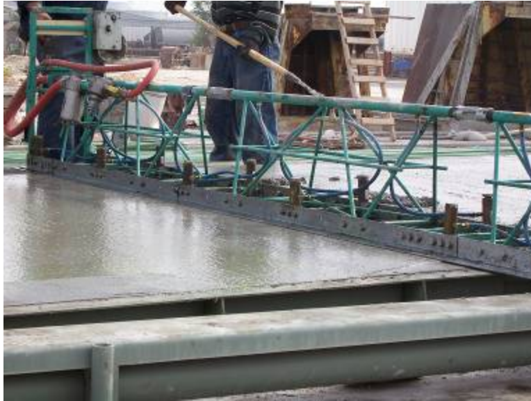
Figure 22. Photo. Vibratory screeding of the panel surface.
