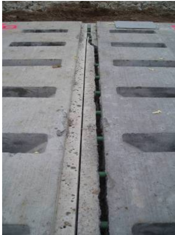
Figure 41. Photo. Expansion joint No. 4 after fracturing during the post-tensioning operation. (photo from MoDOT).
