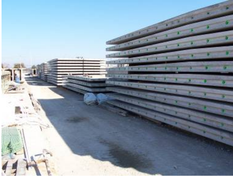
Figure 27. Photo. Panels stacked in the storage area after final curing and inspection.
