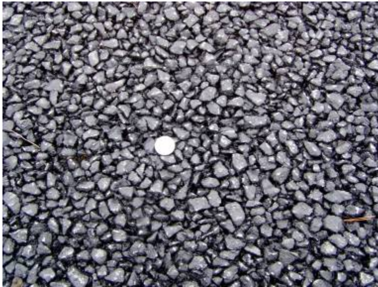
Figure 31. Photo. Finished surface of the permeable asphalt treated base.
