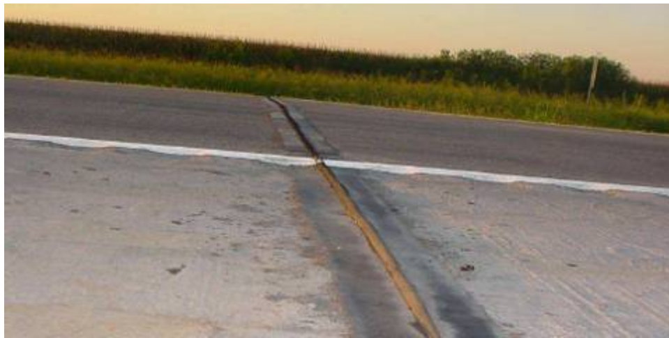
Figure 44. Photo. Joint sealant protruding from the surface of the pavement during under summer climatic conditions. (18)
