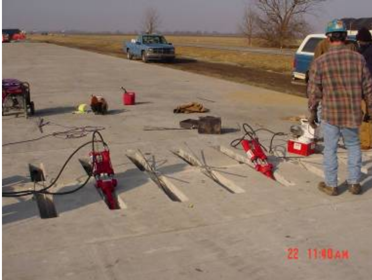
Figure 39. Photo. Final longitudinal post-tensioning completed using two post-tensioning rams (photo from MoDOT).
