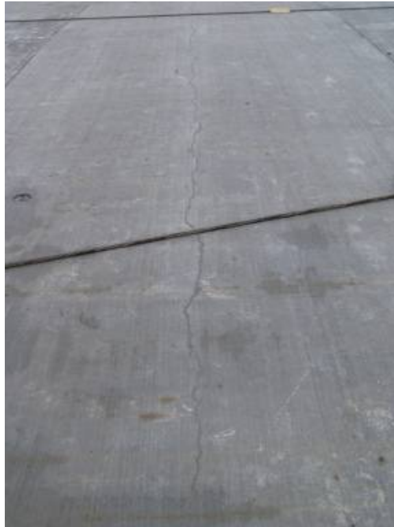
Figure 28. Photo. Typical hairline longitudinal crack observed at the fabrication plant (photo taken after precast panel was delivered to the project site).
