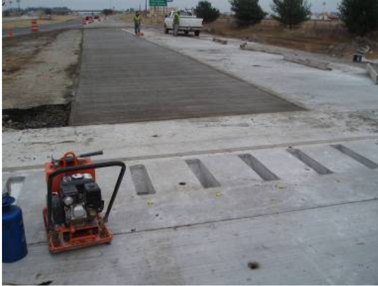
Figure 46. Photo. Adjacent cast-in-place pavement constructed at the end of the PPCP section. (photo from MoDOT)
