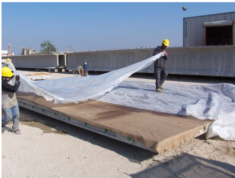
Figure 25. Photo. Wet burlap mat curing of the precast panels after removal from the forms.
