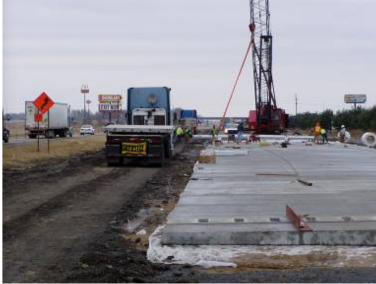
Figure 33. Photo. Staging of delivery trucks and the installation crane.
