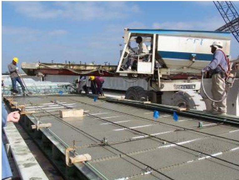
Figure 21. Photo. Concrete placement operation showing the two-lift procedure.
