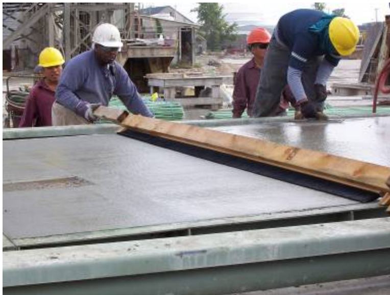
Figure 23. Photo. Application of the light broom texture to the panel surface.
