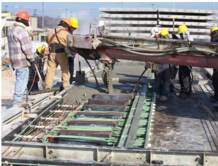
Figure 18. Photo. Fabrication of the first half of a joint panel.
