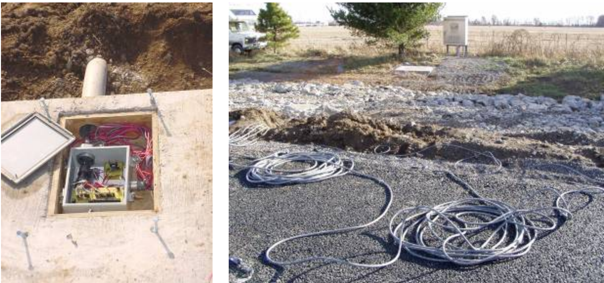
Figure 58. Photo. Junction box within an instrumented precast panel (left) and instrumentation cabinet next to the project site for collecting and uploading data (right).
