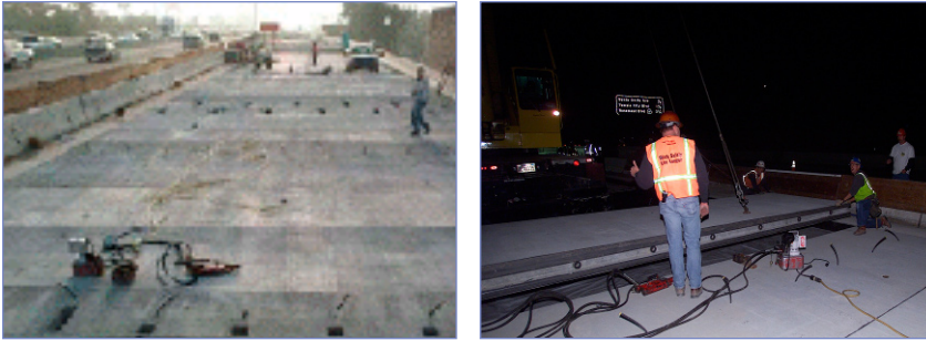
Figure 6. PCPP installation along I-10 in El Monte, California.
