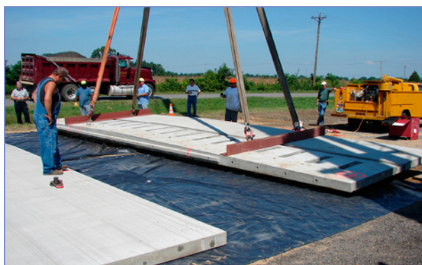
Figure 3. PPCP panel being placed over polyethylene sheet placed over a base.
