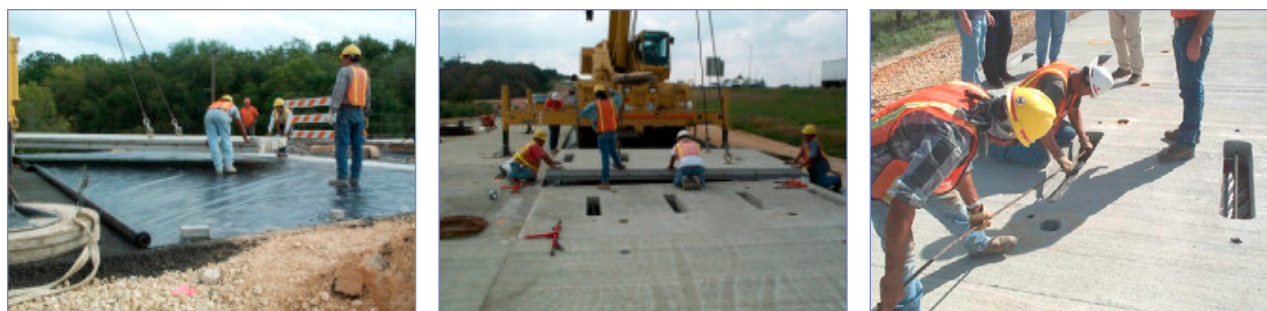
Figure 5. Installation of the precast prestressed concrete pavement system in Georgetown, Texas.
