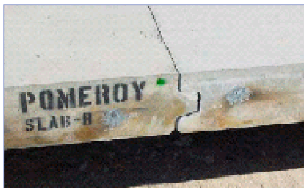
Figure 2. Tongue-and-groove keyway.
