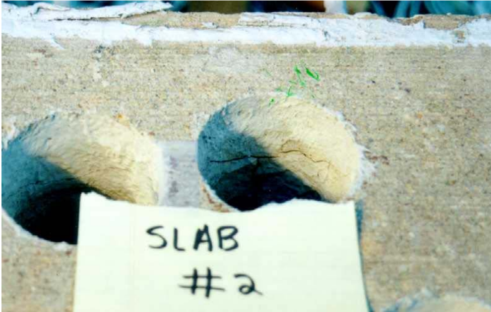
Figure 7. Photo. Cracking and rust staining at the level of reinforcing steel in core holes of slab 2.
