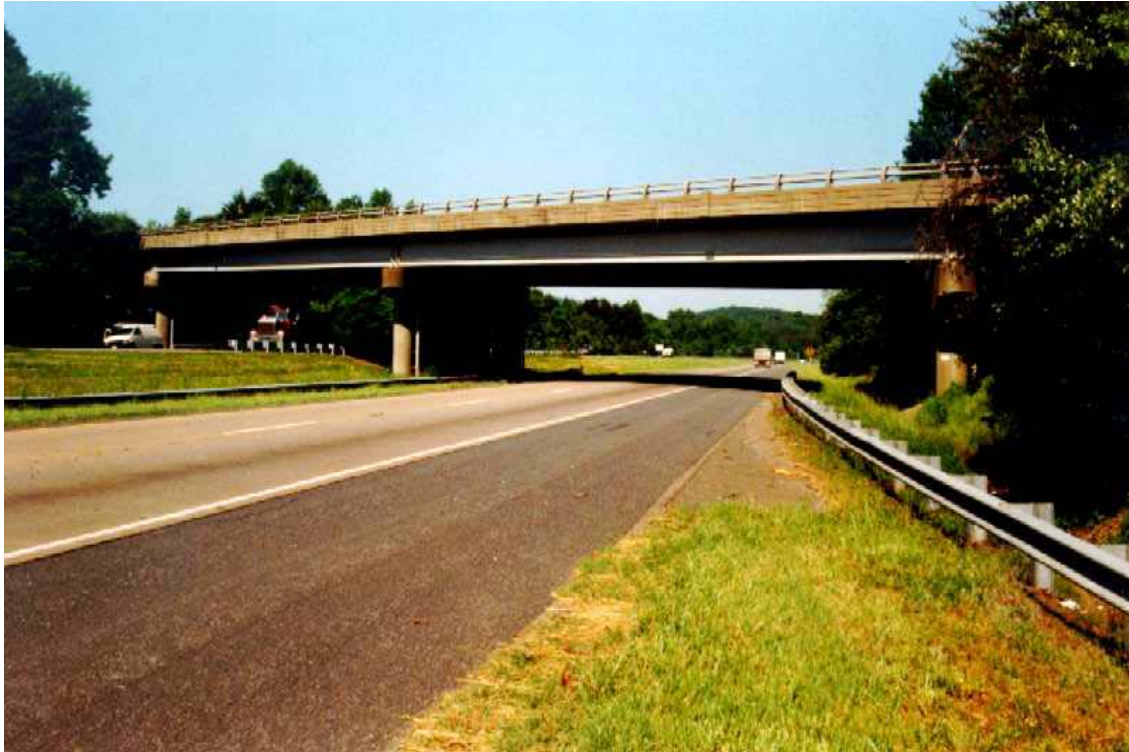
Figure 52. Photo. Route 631 over I-64 bridge in Charlottesville, VA.
