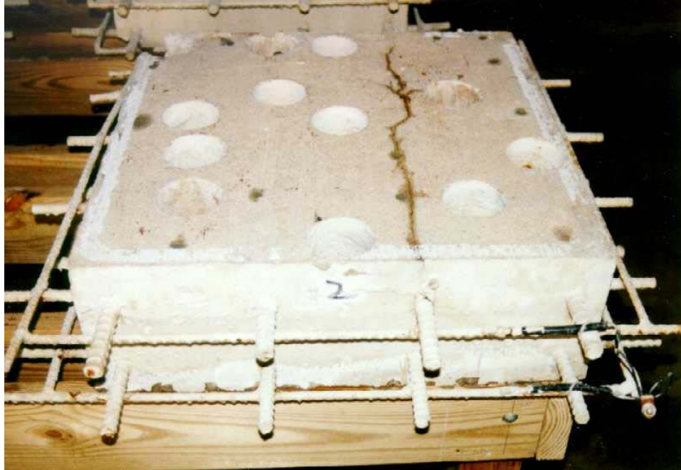
Figure 4. Photo. Condition of crack on the top surface of slab 2 in August 1994.
