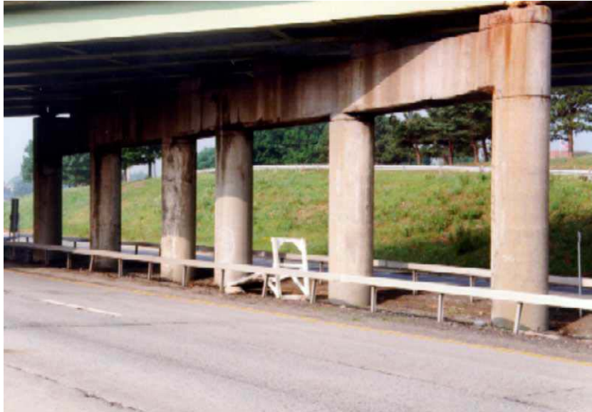
Figure 36. Photo. Pier 2 of the Campus Loop Bridge in Albany, NY.
