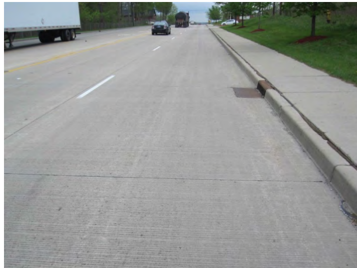
Figure 34. Photo. Overview of SR-19–Section 3, Indiana.
