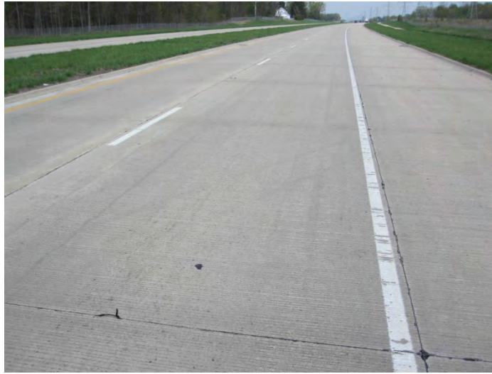
Figure 35. Photo. Overview of SR-331–Section 4, Indiana.
