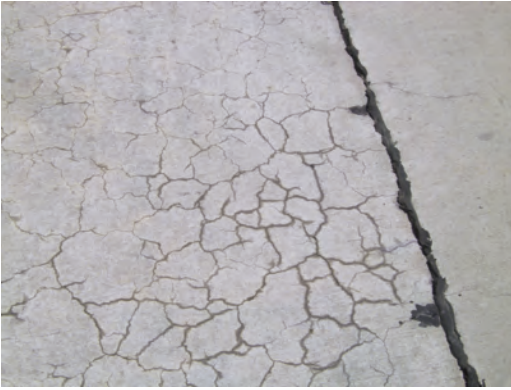
Figure 12. Extrusion of joint-sealing material between adjacent sections of concrete pavement.
