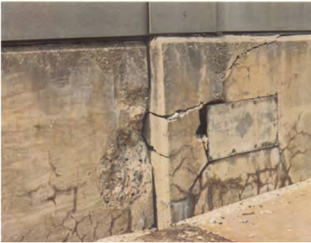
F Figure 11. Expansion with associated spalling of concrete in abutting Jersey barrier sections affected by ASR.
