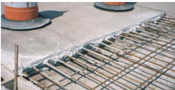
Figure 4. Prepared repair area with exposed longitudinal steel bars.
