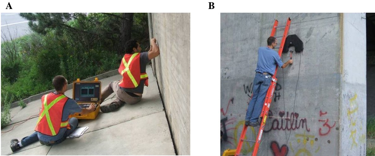
Figure 7.8. Non-destructive testing of ASR-affected concrete structures. A. Impact-echo. B. Non-linear acoustic technique.
