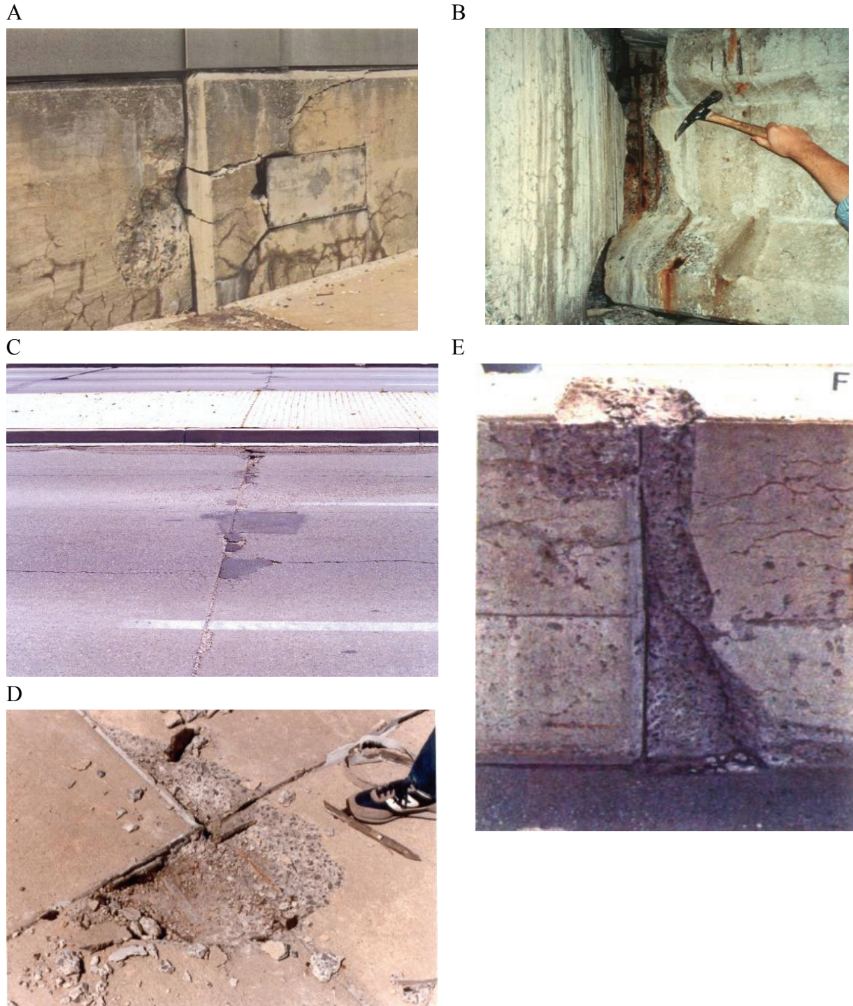
Figure 3.4. (A). Relative movement of abutting sections of parapet wall in a bridge structure affected by ASR (Stark 1991). (B). Expansion of bridge girder leading to loss of clearance between the girder and embankment and eventually crushing of the girder end with localized spalling. (C). Expansion causing spalling at joints in a concrete pavement incorporating a highly-reactive aggregate. (D). Expansion causing spalling at joints and extrusion of sealant material in a concrete pavement incorporating a highly reactive aggregate. (E). Expansion with associated severe spalling in abutting jersey barrier sections affected by ASR.
