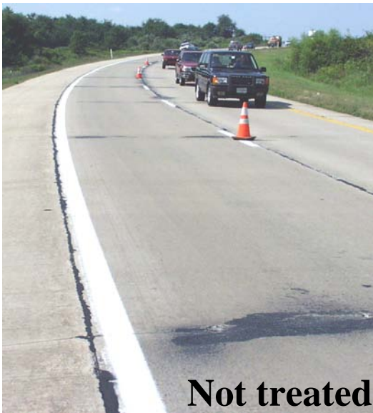
Figure 3. Concrete pavement affected by ASR.
