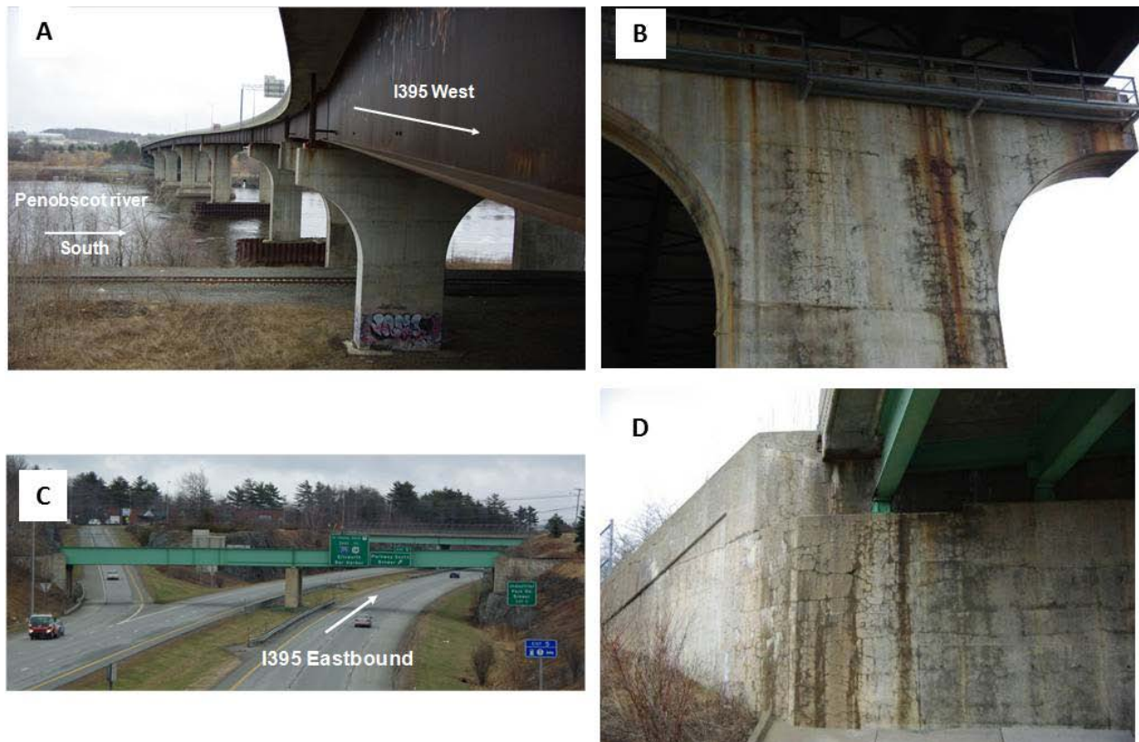
Figure 9. I-395 and 5 th Parkway bridges.
