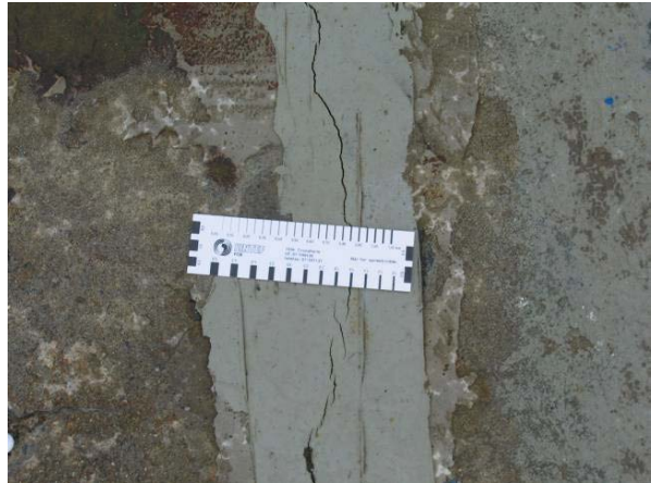
Figure 1. Large hydraulic dam affected by ASR in Norway. A: General view of the dam. B&C: View of the epoxy-injected pillars. D: Cracking reappearing in the injected cracks.
