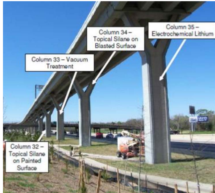
Figure 14. Columns 32-35 in Houston, TX.
