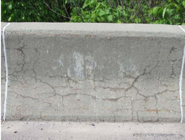
C – 100% silane + elastomeric coating 2013
