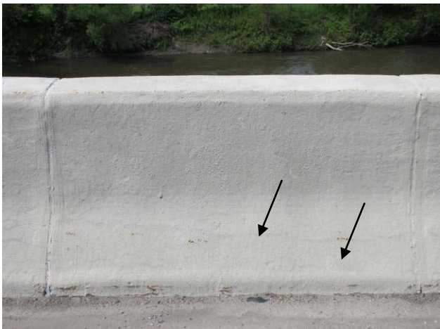
Figure 248. Typical examples of the condition of treated barrier walls (driving lane).
