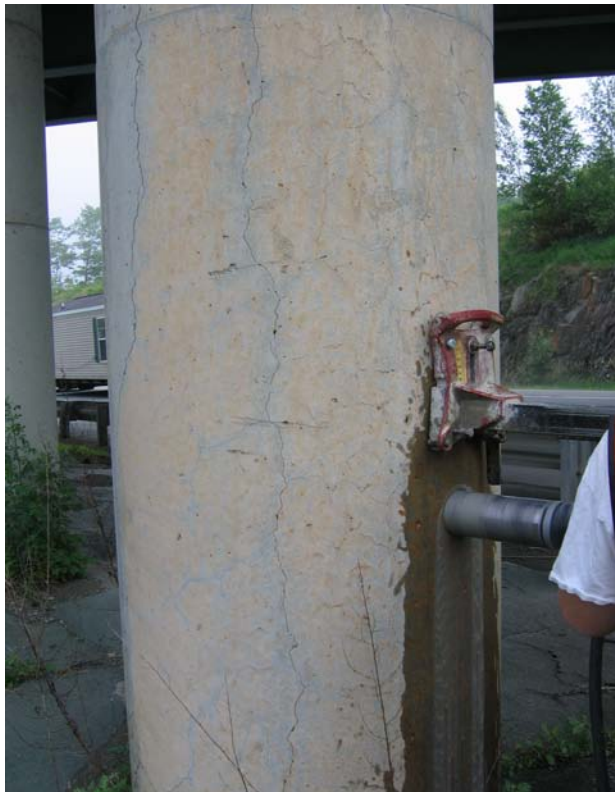
Figure 106. Condition of concrete columns of the South Parkway bridge over I-395. A&B: Site (column) 1. C&D: Site (column) 6.
