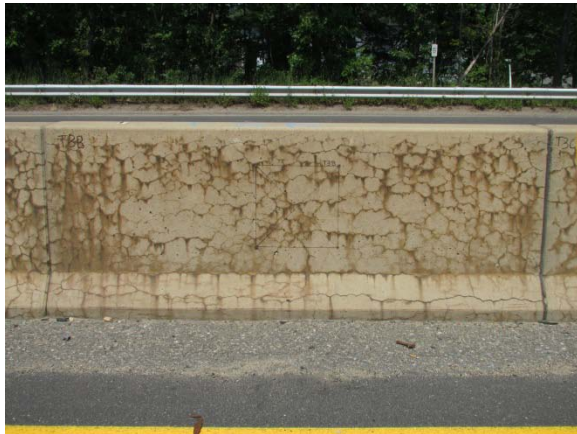
Figure 150. Visual observations over time of section T3B.
