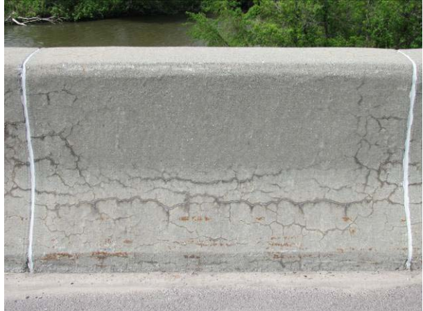
D – 100% silane + elastomeric coating 2013
