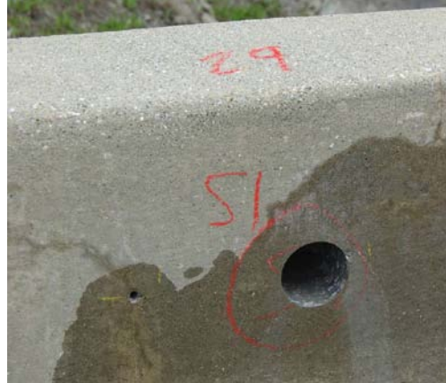
Figure 238. I-89 bridges and barrier walls.
