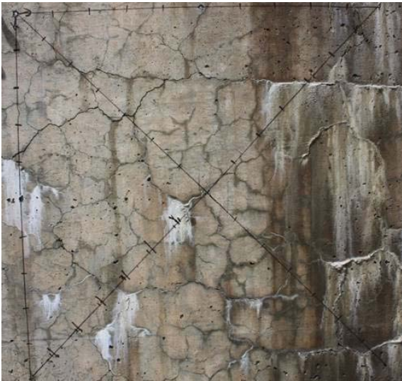
Figure 98. Examples of crack map sections before (2010) and after (2013) treatments (5 th Parkway (Robertson Road) bridge over I-395).
