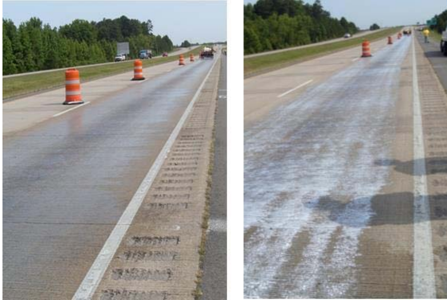
Figure 50. Photograph of pavement sections treated topically with 100 percent silane (left) and 40 percent silane (right). The slow drying of the 40 percent silane section resulted in a slick surface that required lane closures for about 48 hours.
