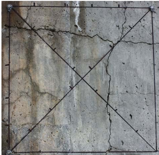
Figure 114. Examples of crack map sections before (2010) and after (2013) treatments (Green Point Road bridge over 1-395).
