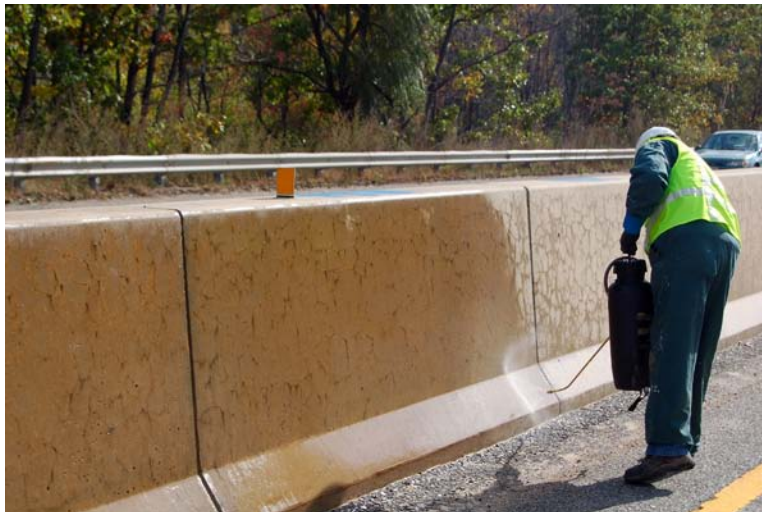
Figure 126. Silane product applied with a handheld pump sprayer.
