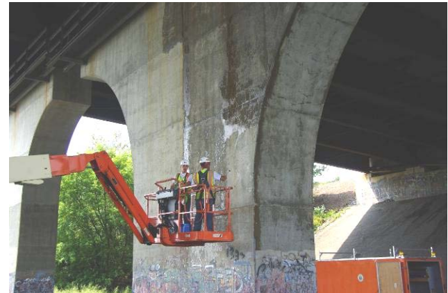
Figure 72. Application of surface treatments.
