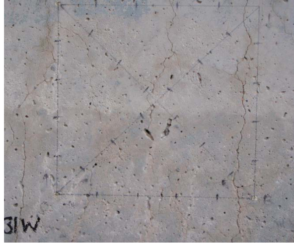
B – Column 31 – West Face 2009
