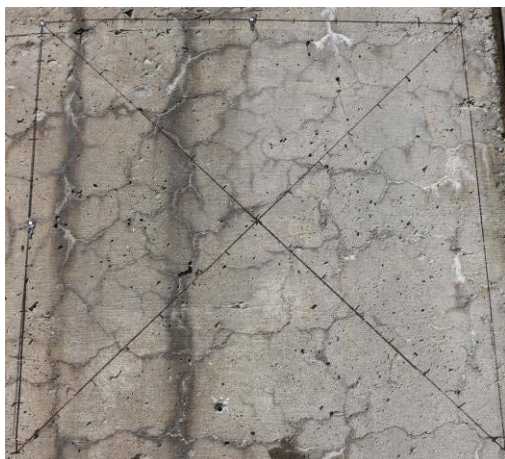
Figure 80. Examples of crack map sections before (2010) and after (2013) treatments (I-395 bridge over Main Street).
