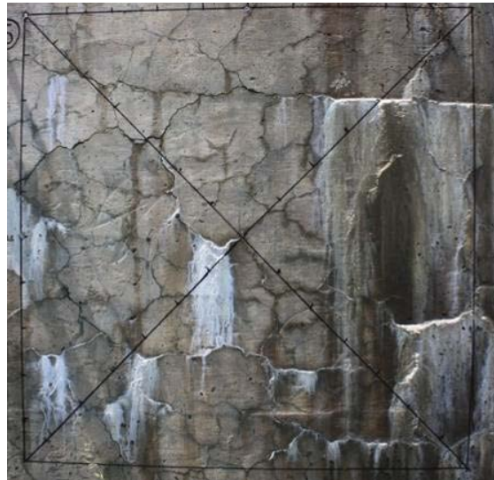
Figure 98. Examples of crack map sections before (2010) and after (2013) treatments (5 th Parkway (Robertson Road) bridge over I-395).
