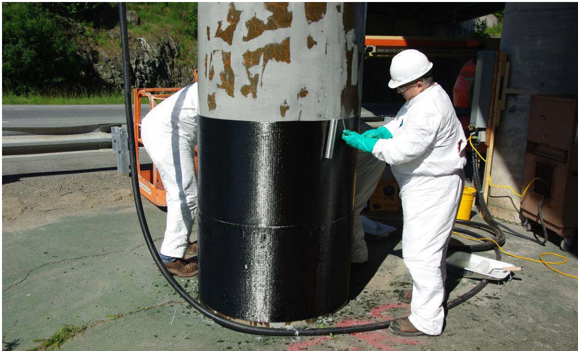
Figure 27. Application of FRP to bridge column in Maine.
