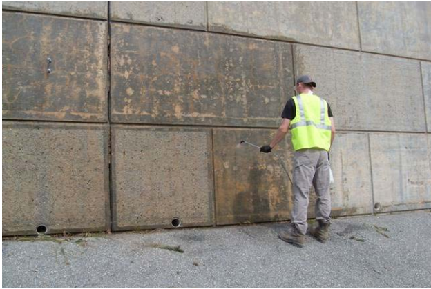
Figure 231. Application of surface treatments.
