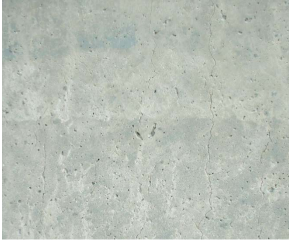
A – Column 31 – West Face 2006
