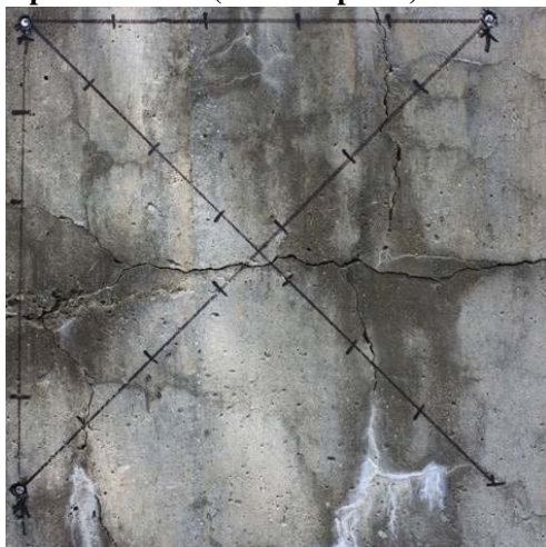
Figure 113. Examples of crack map sections before (2010) and after (2013) treatments (Green Point Road bridge over 1-395).
