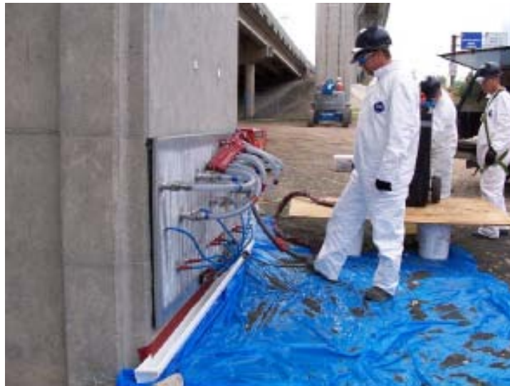
Figure 190. Lithium vacuum treatment on Column 45.
