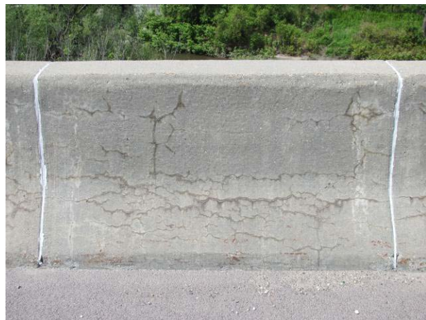
Figure 247. Typical examples of the condition of control and treated barrier walls (driving lane).
