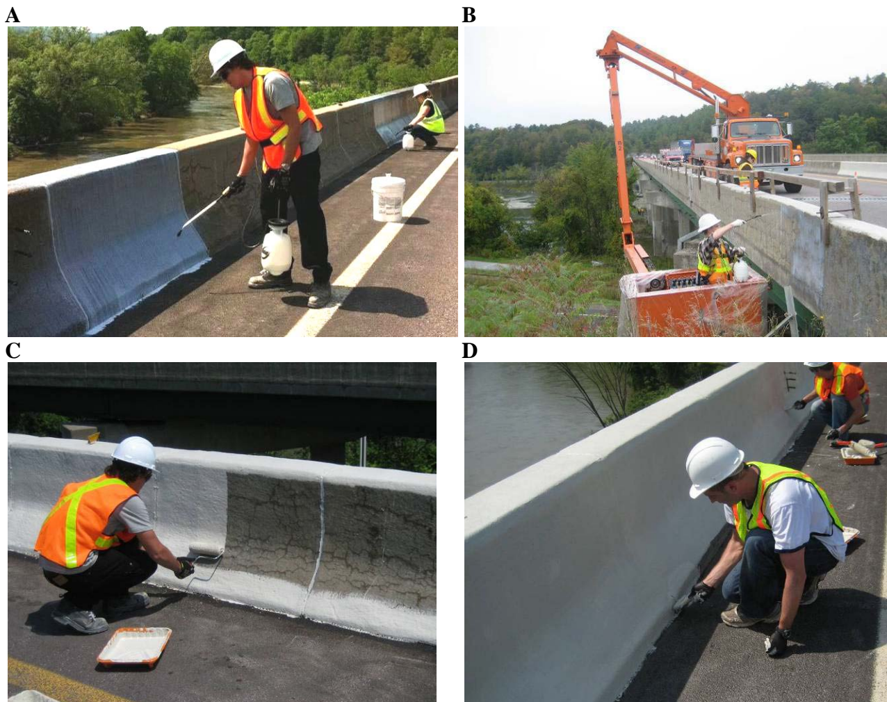
Figure 243. Application of surface treatments.
