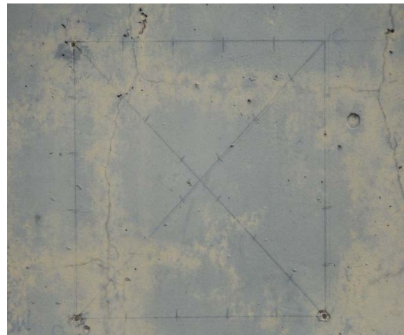
Figure 216. Visual observation of Column 43 Southwest face.
