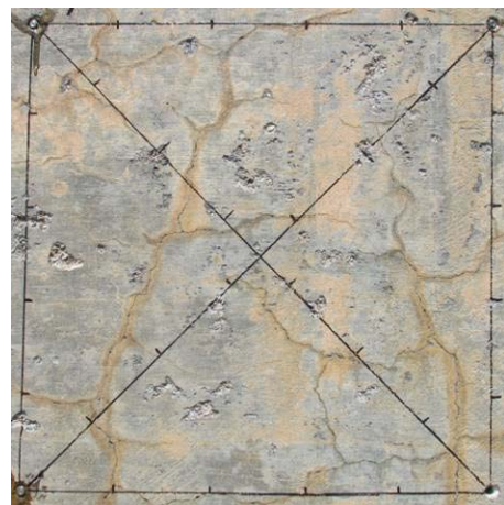
Figure 235. Examples of crack map sections before (2012) and after (2013) treatments (retaining wall).
