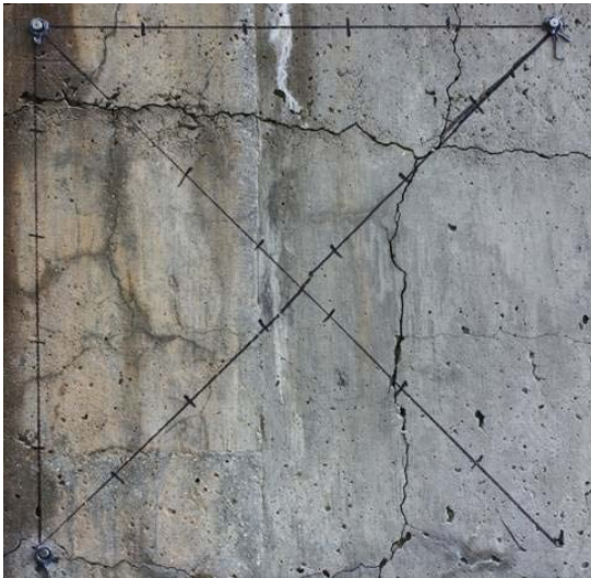
Figure 114. Examples of crack map sections before (2010) and after (2013) treatments (Green Point Road bridge over 1-395).
