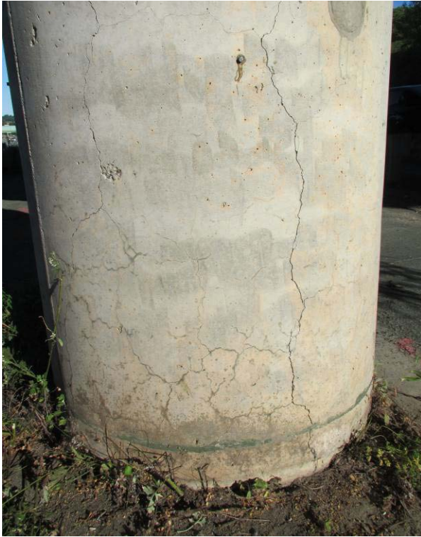
C – Lithium electrochemical (site 2: exposed) 2012
