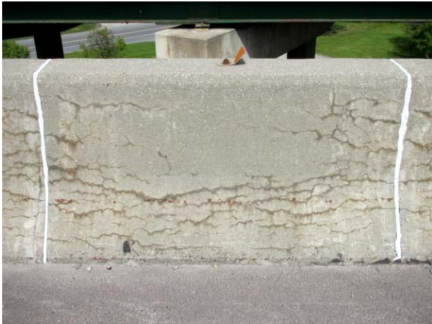
Figure 249. Typical examples of the condition of control and treated barrier walls (passing lane).
