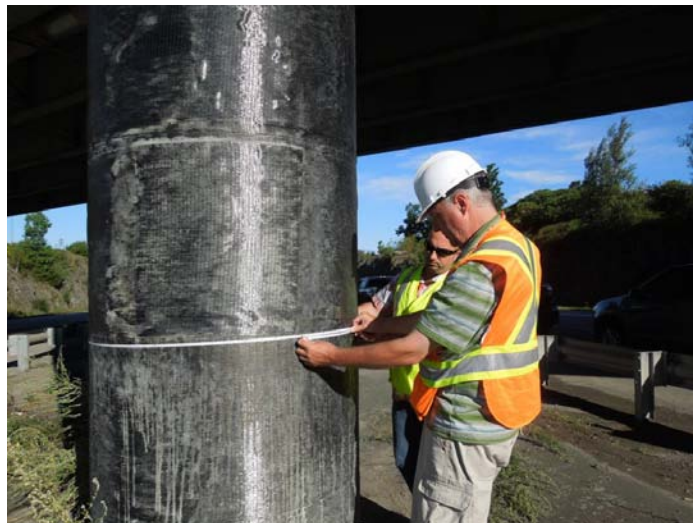
Figure 11. Measurement of the circumferential expansion on concrete columns.
