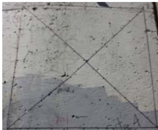
Figure 80. Examples of crack map sections before (2010) and after (2013) treatments (I-395 bridge over Main Street).
