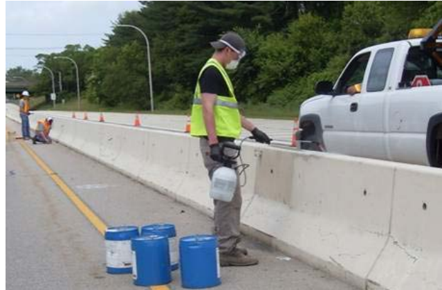
Figure 231. Application of surface treatments.
