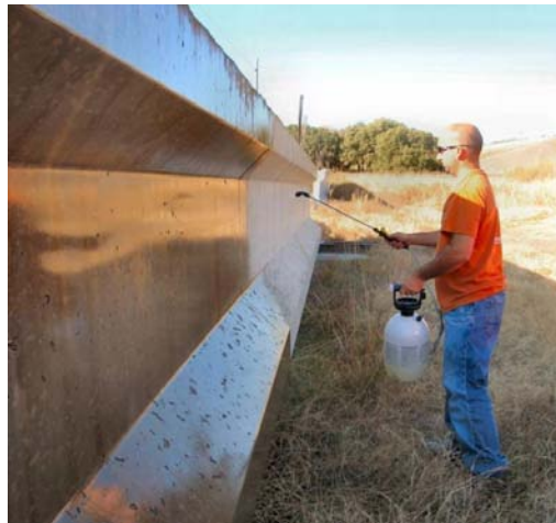
Figure 177. Topical silane application on the precast beams
