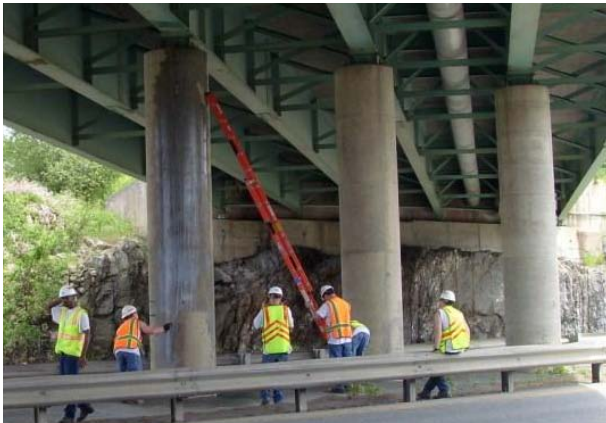
Figure 72. Application of surface treatments.
