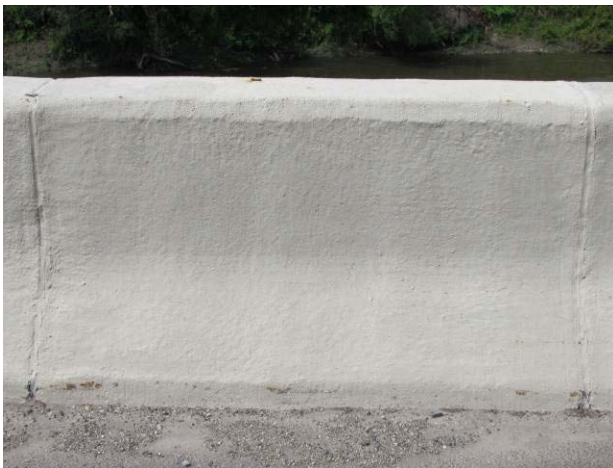
Figure 248. Typical examples of the condition of treated barrier walls (driving lane).
