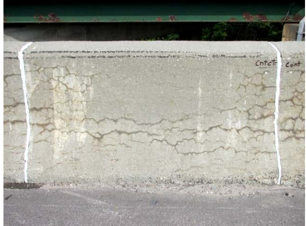
D – 100% silane + elastomeric coating 2013
