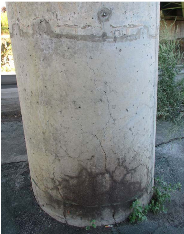
Figure 108. Condition of concrete columns of the South Parkway bridge over I-395. A&B: Site (column) 5. C&D: Site (column) 2.
