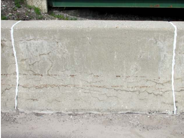
C – 100% silane + elastomeric coating 2013
