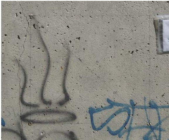
Figure 212. Visual observation of Column 41 Southwest face.
