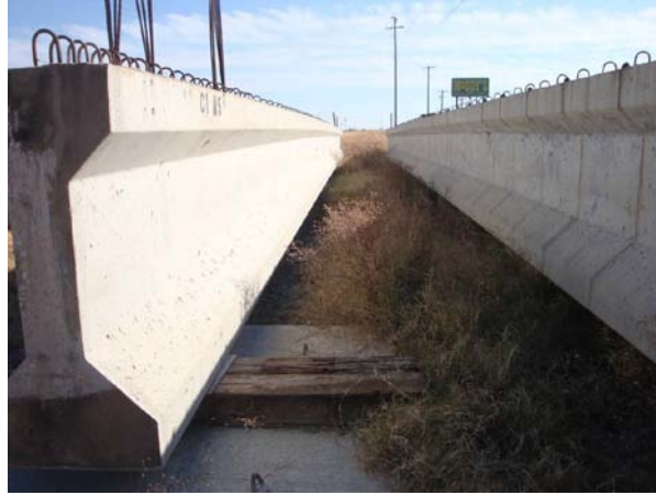
Figure 171. Beams 1 and 2 resting on railroad ties.
