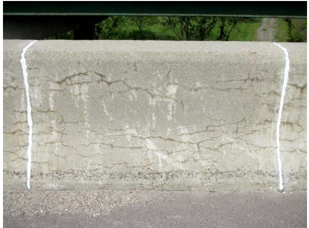
Figure 249. Typical examples of the condition of control and treated barrier walls (passing lane).
