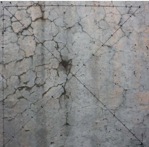
Figure 99. Examples of crack map sections before (2010) and after (2013) treatments (5 th Parkway (Robertson Road) bridge over I-395).
