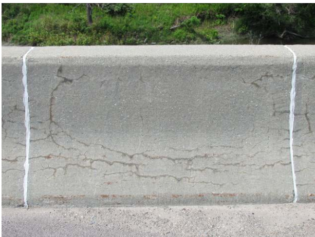
Figure 247. Typical examples of the condition of control and treated barrier walls (driving lane).
