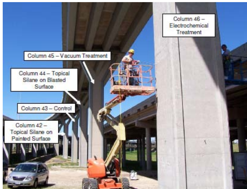
Figure 188. Columns 42-46 in Houston, TX, along with their treatments.
