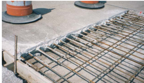
Figure 9. Maintaining reinforcing steel continuity in CRCP. (1)
