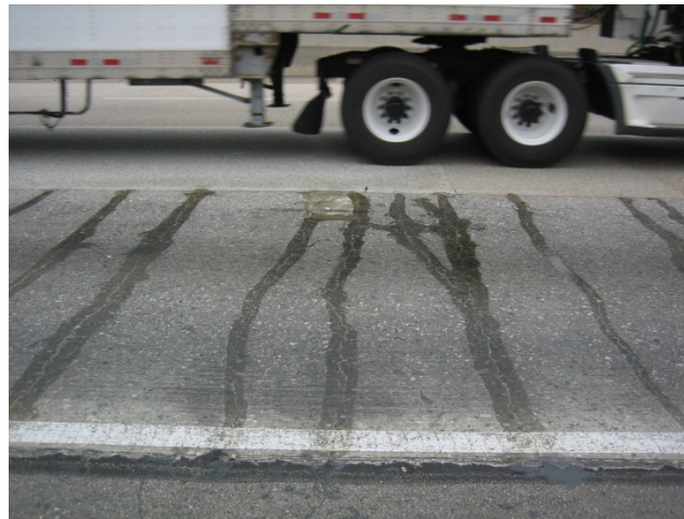
Figure 16. Epoxy sealing of CRCP cracks.
