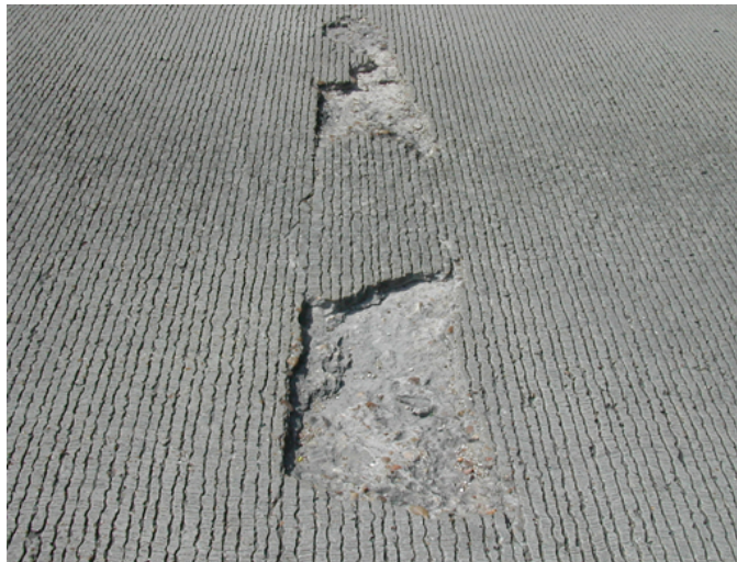
Figure 15. Shallow spall. (19)
