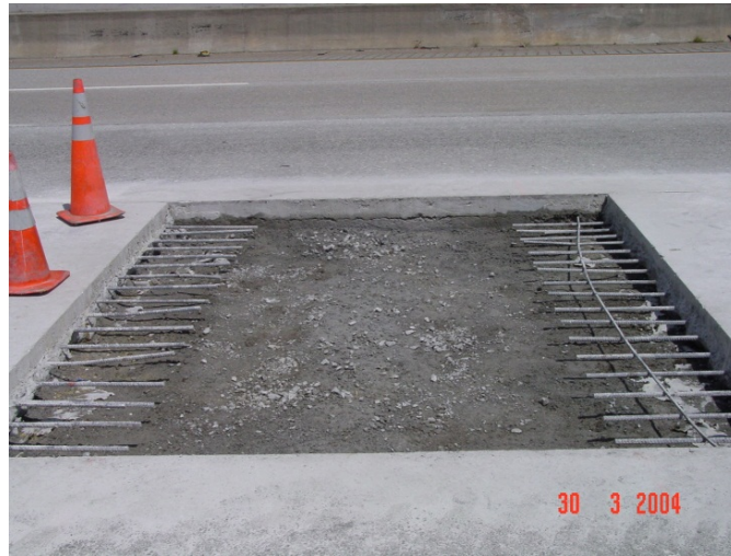
Figure 8. Exposed steel for splicing new rebars in CRCP.
