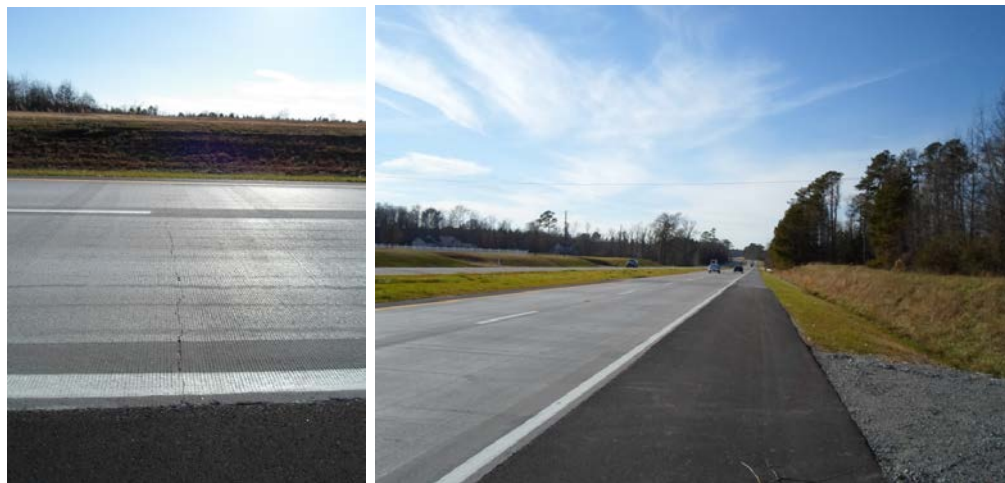
Figure 19. Bonded overlay on U.S. Route 58 in Virginia, as constructed.
