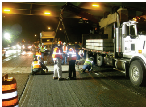
Figure 2. Photo. Installation of intermittent repair.
