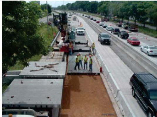
Figure 3. Photo. Example of JPrCP application.
