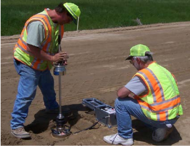
Figure 2. Photo. Lightweight deflectometer testing on a base material.
