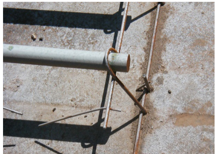
Figure 5. Stake anchoring a dowel basket in place
