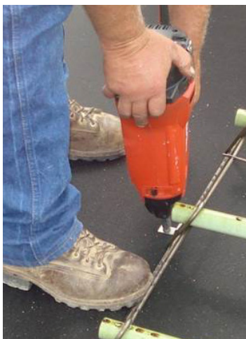
Figure 8. Nail-down clip installation using pneumatic tool
