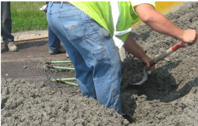
Figure 11. Crew addressing a collapsed dowel basket during paving, a very difficult challenge once the paving is underway, underscoring the need for proper anchoring and basket stability
