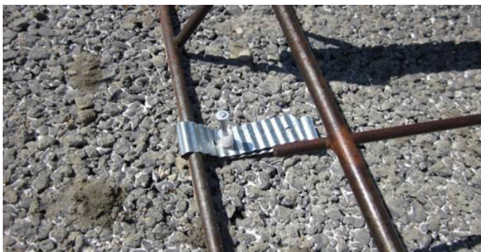
Figure 6. Wrap-around dowel basket clip
