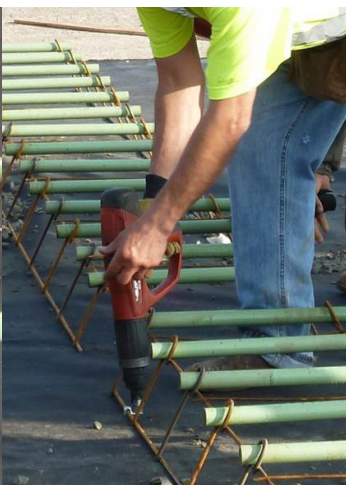
Figure 9. Nail-down clip installation using a powder-actuated gun
