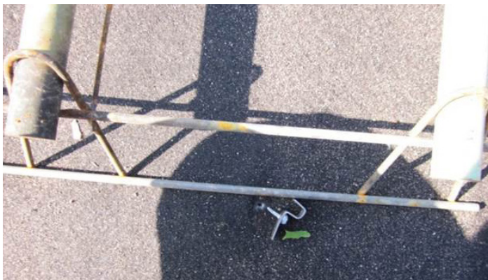
Figure 7. Nail-down basket clip
