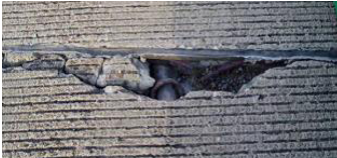
Figure 2. Mislocated dowel too close to the surface causing joint deterioration (spalling)
