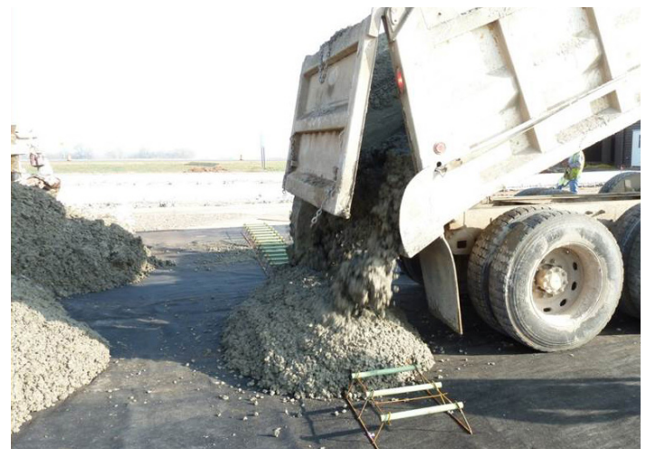
Figure 13. Haul truck end-dumping concrete directly onto dowel basket
