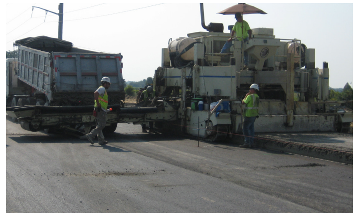
Figure 12. Side-belt placer operation
