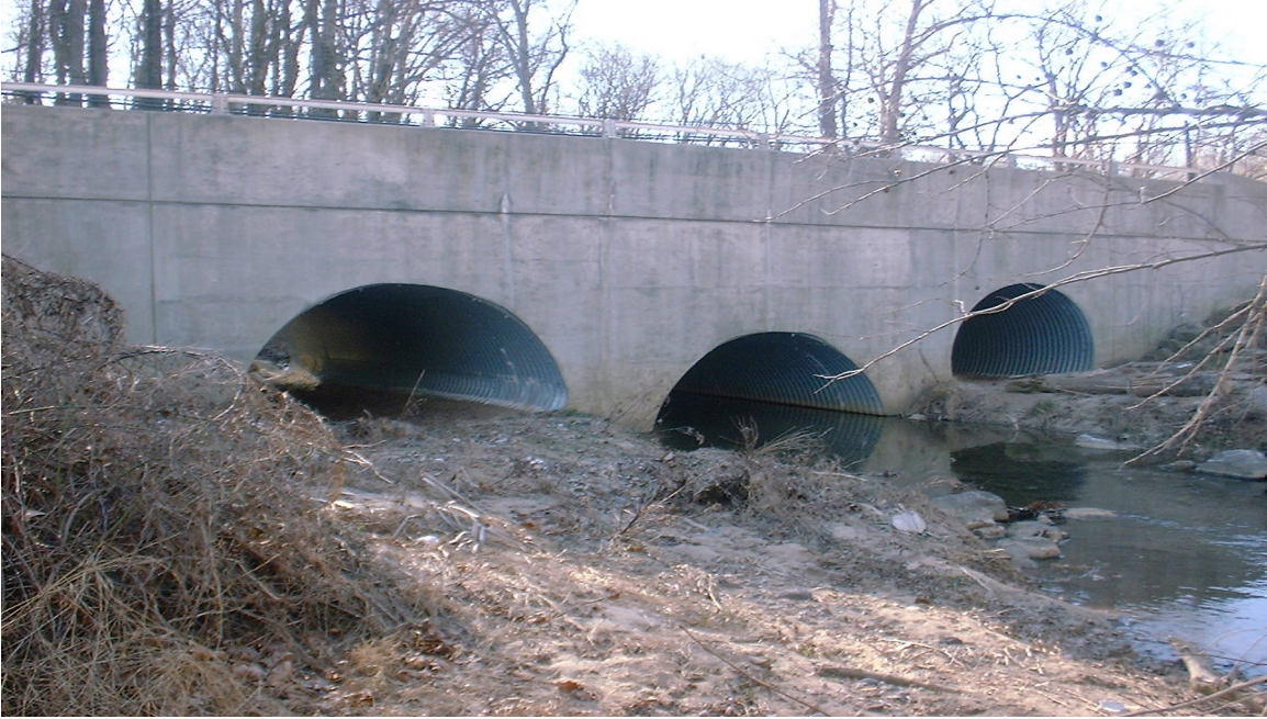
Figure 8.8 Downstream of culvert, shortly after project completion in 1994
