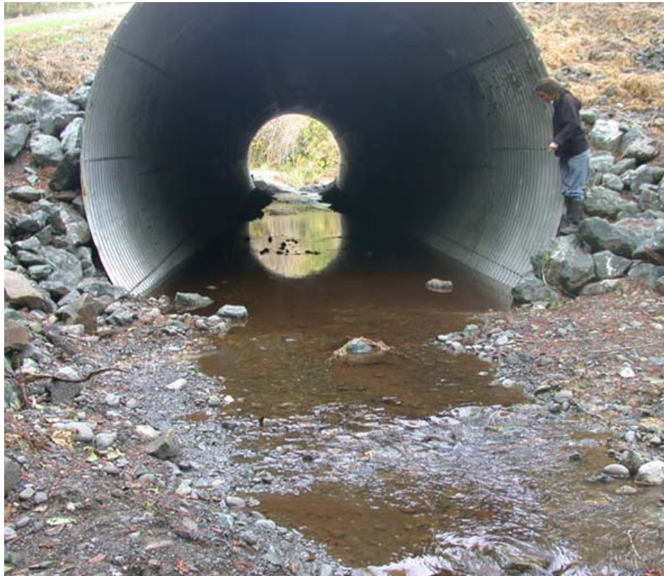
Figure 8.4 Replacement culvert (United States Forest Service 2006b)
