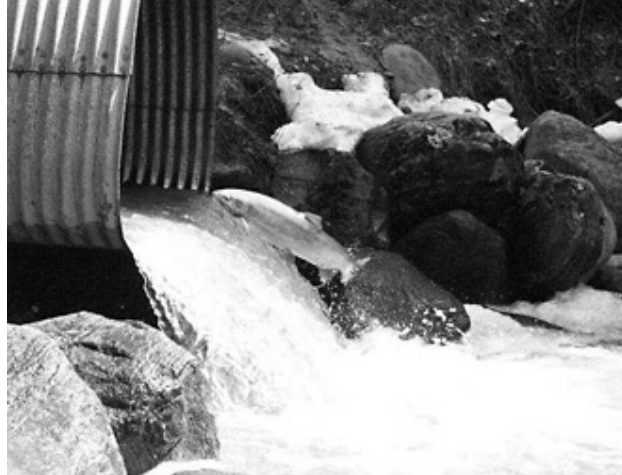
Figure 3.4 Drop and velocity barrier (Alaska Department of Fish and Game 2005)
