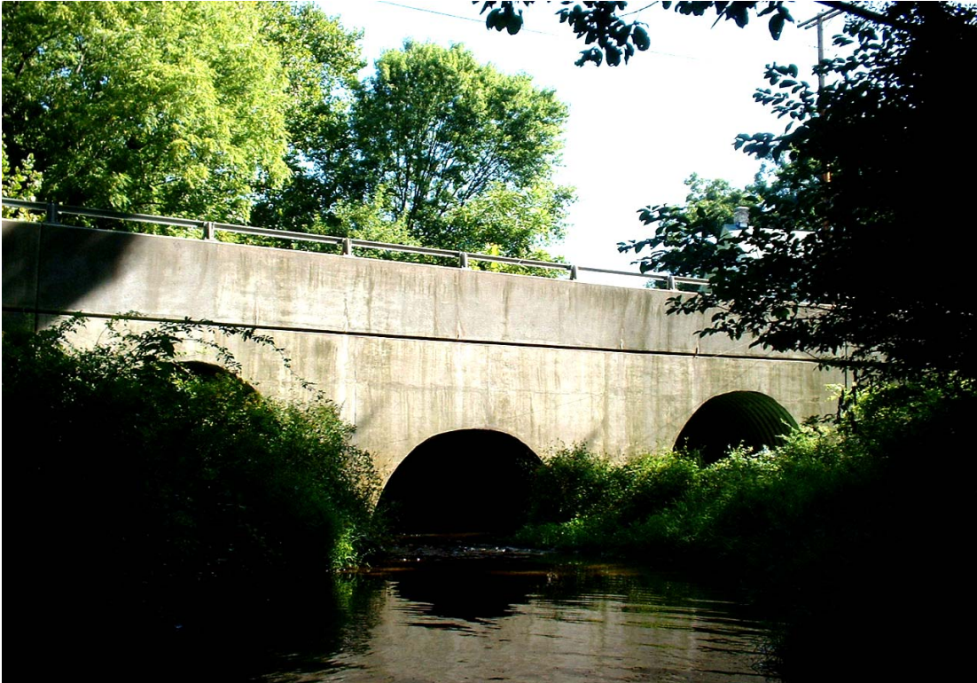
Figure 8.9 Upstream of current crossing in 2005
