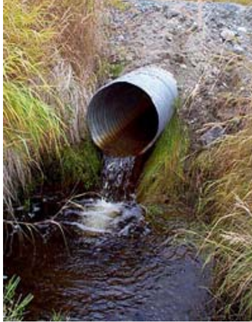
Figure 3.3 Perched outlet, leap barrier (Alaska Department of Fish and Game 2005)
