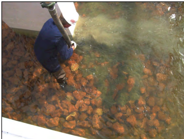
Figure 12.11. Underwater partial grouting of riprap.
