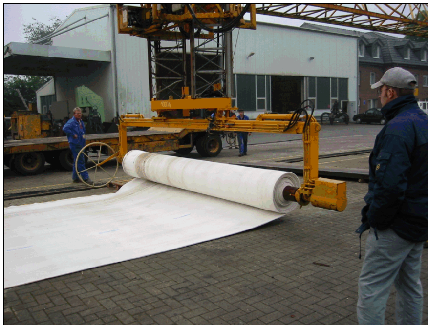
Figure 11.18. SandMat™ geocomposite blanket being unrolled. (photo from NCHRP Project 24-07(2), courtesy Colcrete – Von Essen Inc.)
