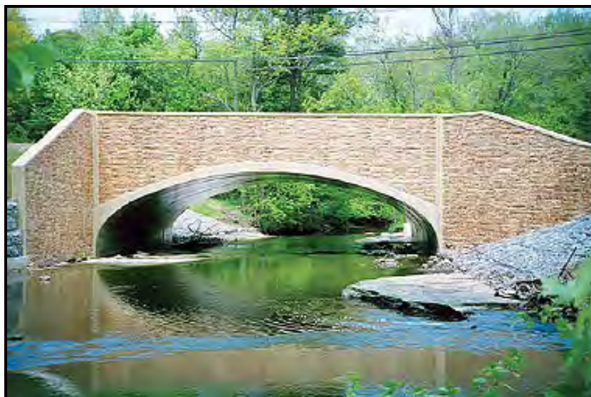
Figure 18.1 Bottomless Culvert on Whitehall Road over Euclid Creek in Cuyahoga County, OH.
