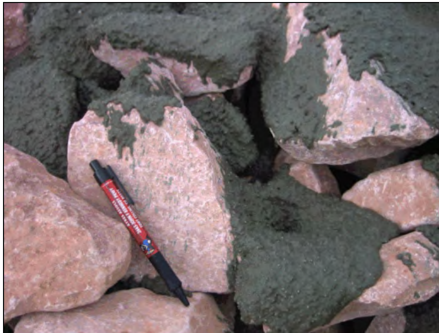
Figure 12.9. Surface of the riprap after partial grouting.
