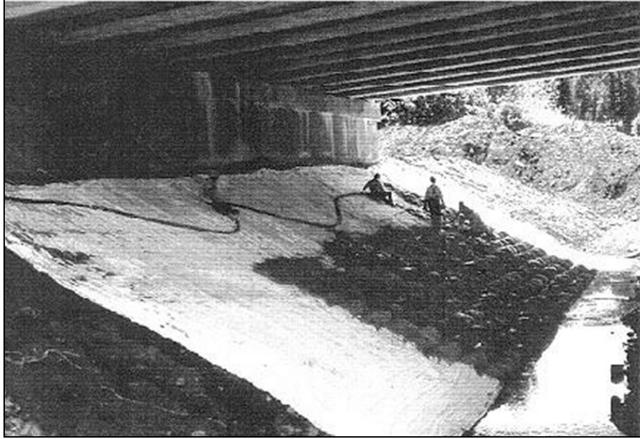
Figure 9.9. Installation of articulating grout filled mat proceeding upslope (ODOT).
