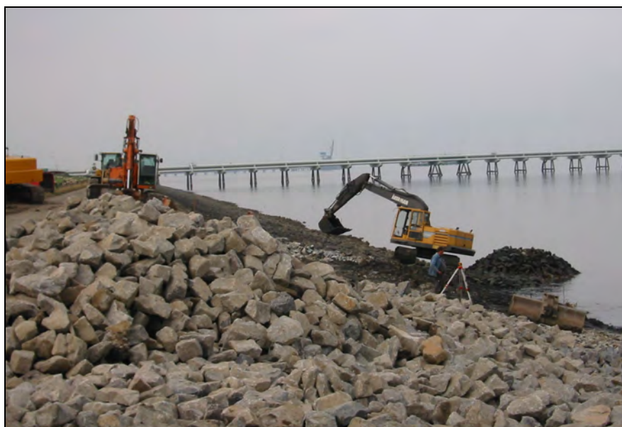
Figure 4.11. Placing riprap with hydraulic excavators.
