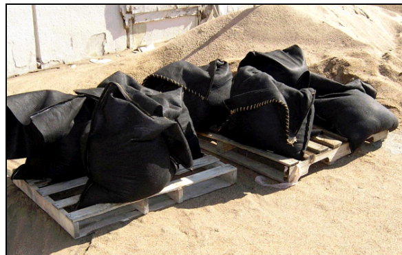
Figure 11.10. Geotextile containers before installation around the pier.
