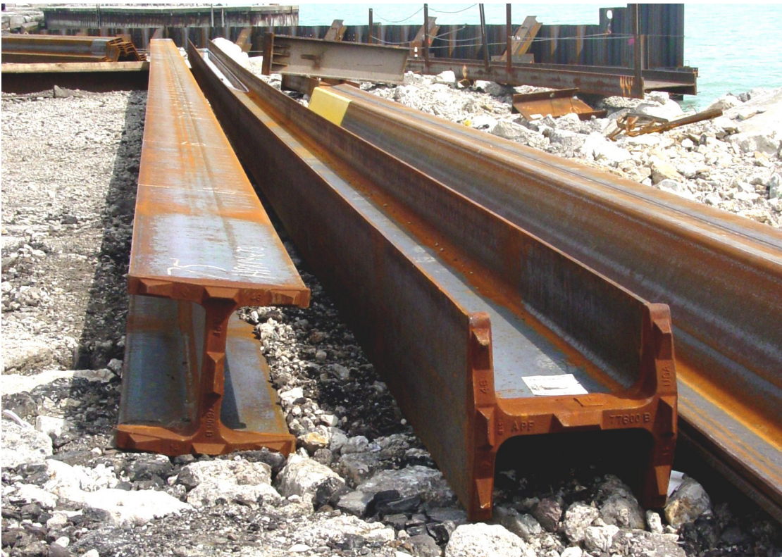
Figure 6-10 H-piles with driving shoes.
