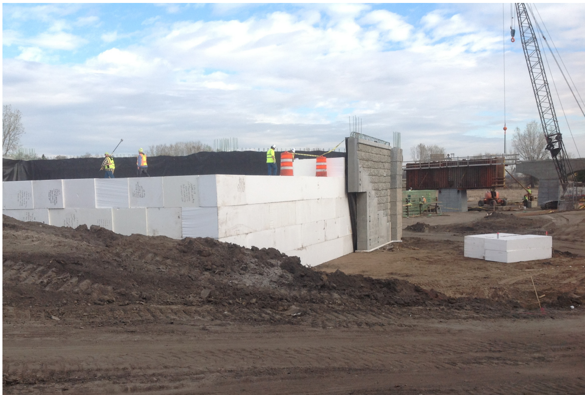
Figure 7-61 Geofoam block approach embankment (courtesy MnDOT).
