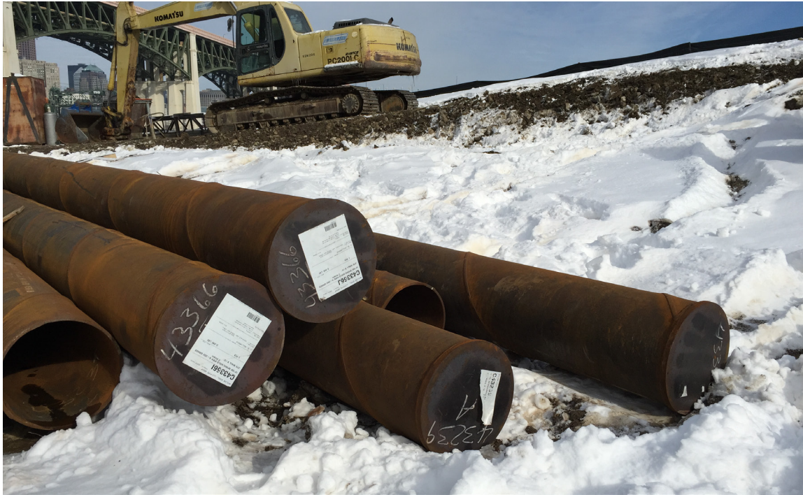
Figure 6-11 Typical 16 inch closed end pipe pile.
