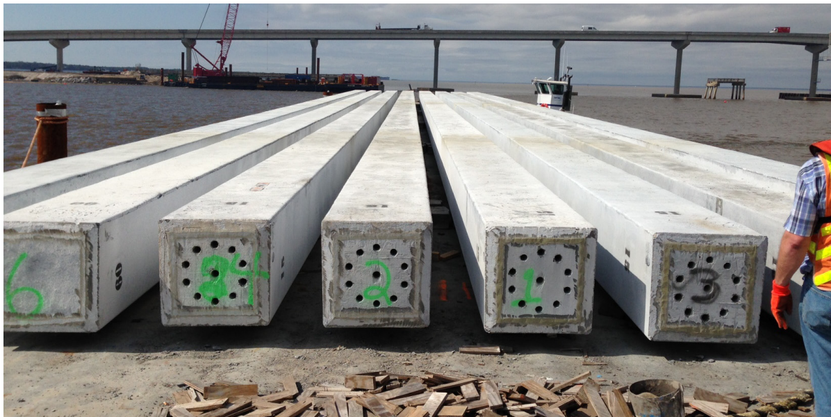
Figure 6-21 Square prestressed concrete piles.
