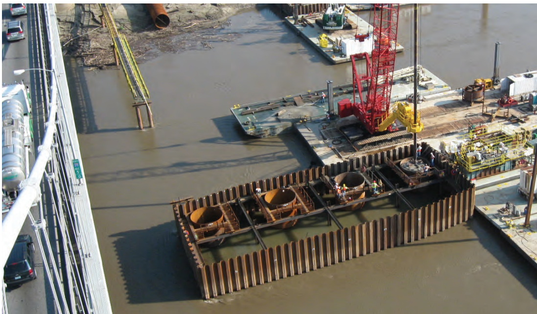
Figure 1-9 Construction of 12-ft Diameter Drilled Shafts for the Main Pylon Foundation, Christopher S. Bond Bridge, Kansas City (photo by Gary Naugle, MoDOT)
