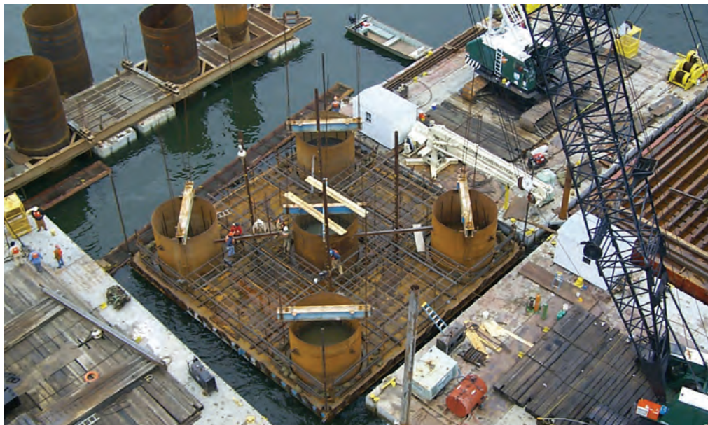
Figure 1-13 Group of Drilled Shafts for Large Loads
