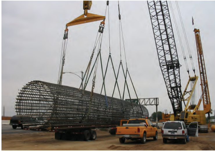
Figure 8-23 Photograph of Rebar Cage Being Delivered to Site
