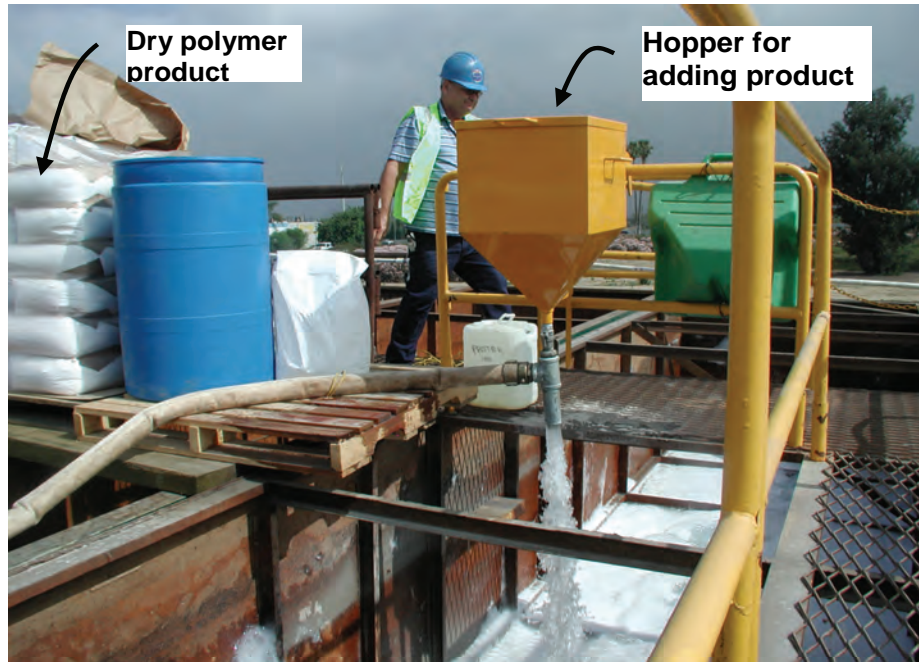
Figure 7-6 Field Mixing Polymer Slurry by Circulating Between Tanks
