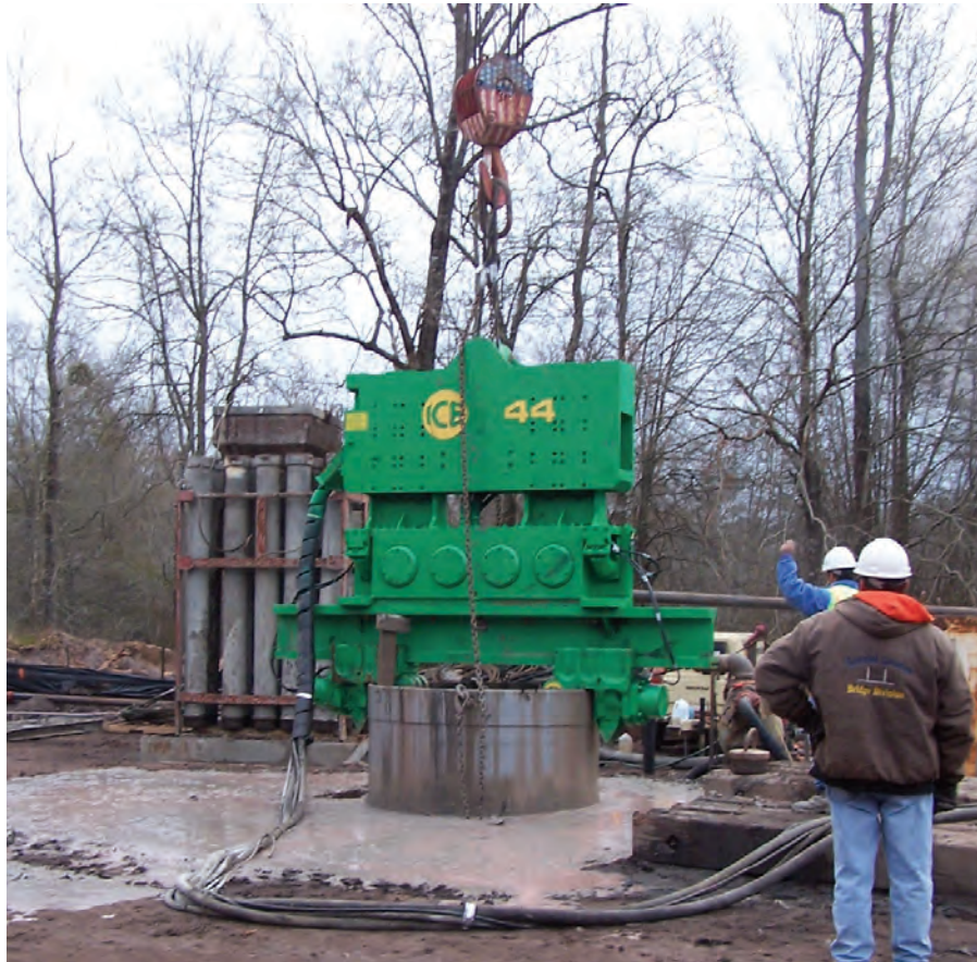
Figure 6-8 Extraction of Temporary Casing Using a Vibratory Hammer
