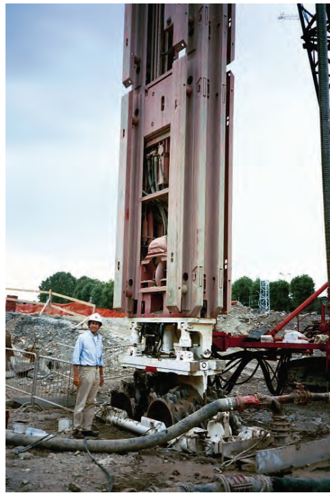
Figure 5-13 Excavation of a Diaphragm Wall or Barrette Using a Clam
