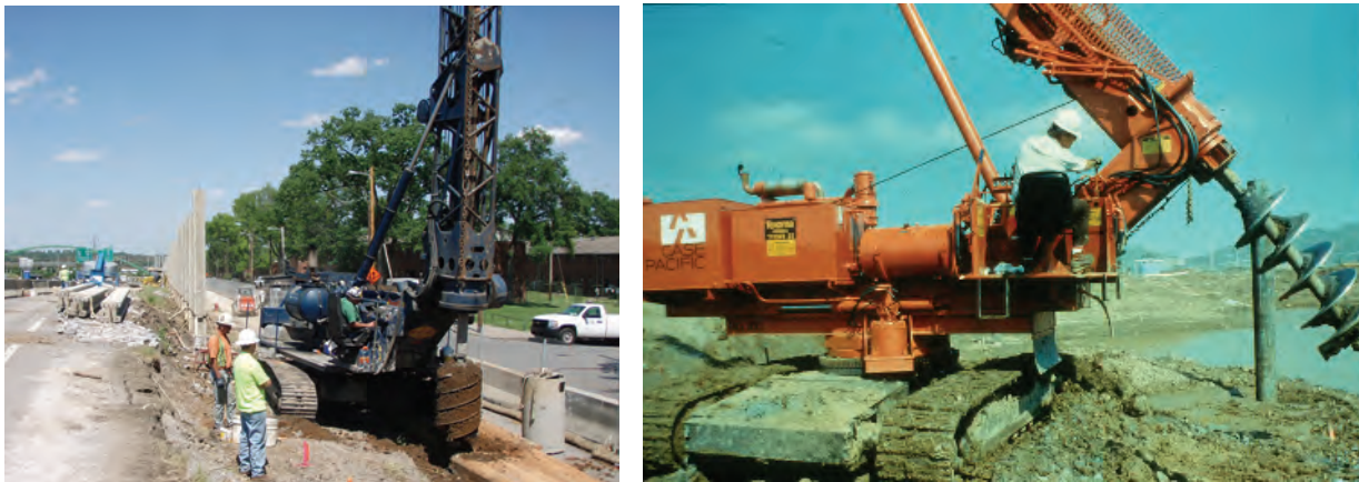
Figure 1-16 Drilled Shafts for Soundwall (left) and Sign (right)
