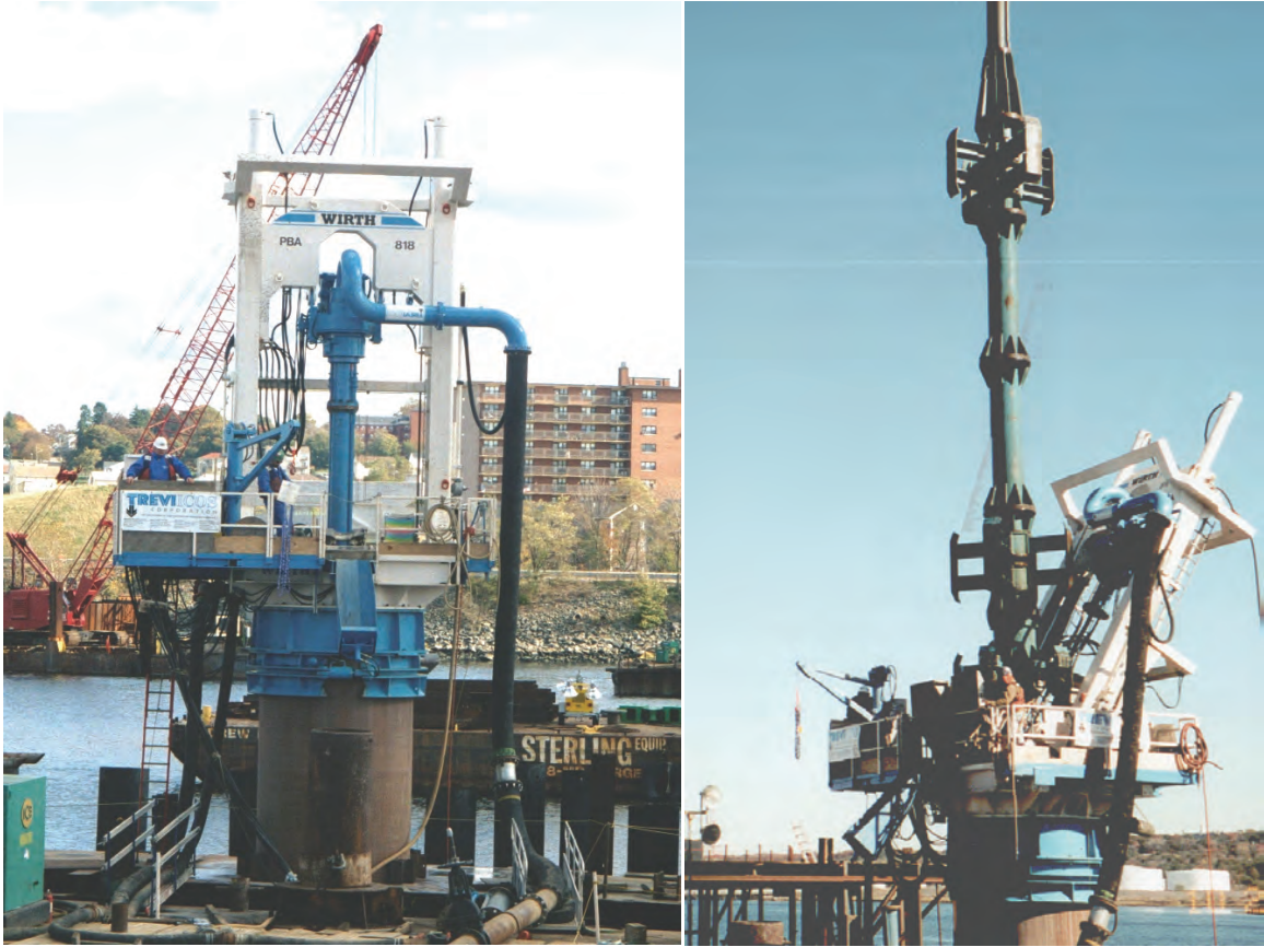
Figure 5-10 Top-Drive Reverse Circulation Drill
