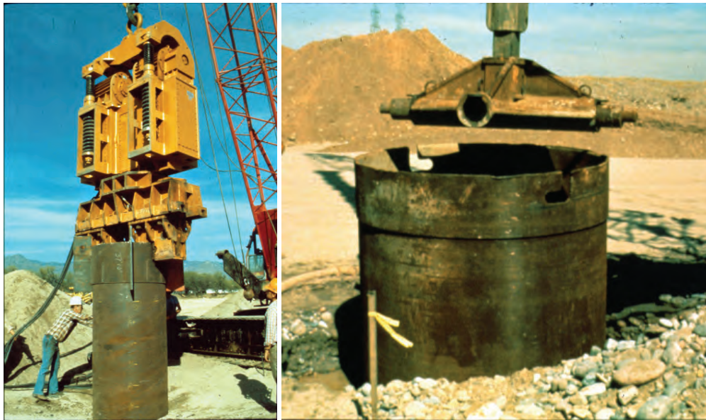
Figure 4-10 Use of a Vibro-Hammer (Left) and Twister Bar (Right) to Advance Casing
