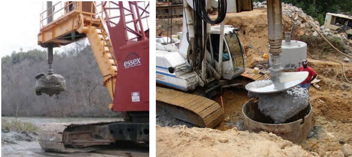
Figure 1-8 Typical Modern Drilled Shaft Rigs
