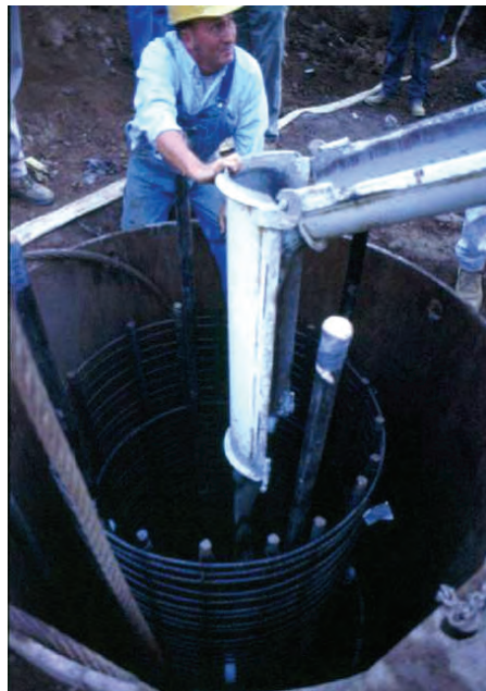
Figure 4-4 Placement of Concrete into a Dry Excavation
