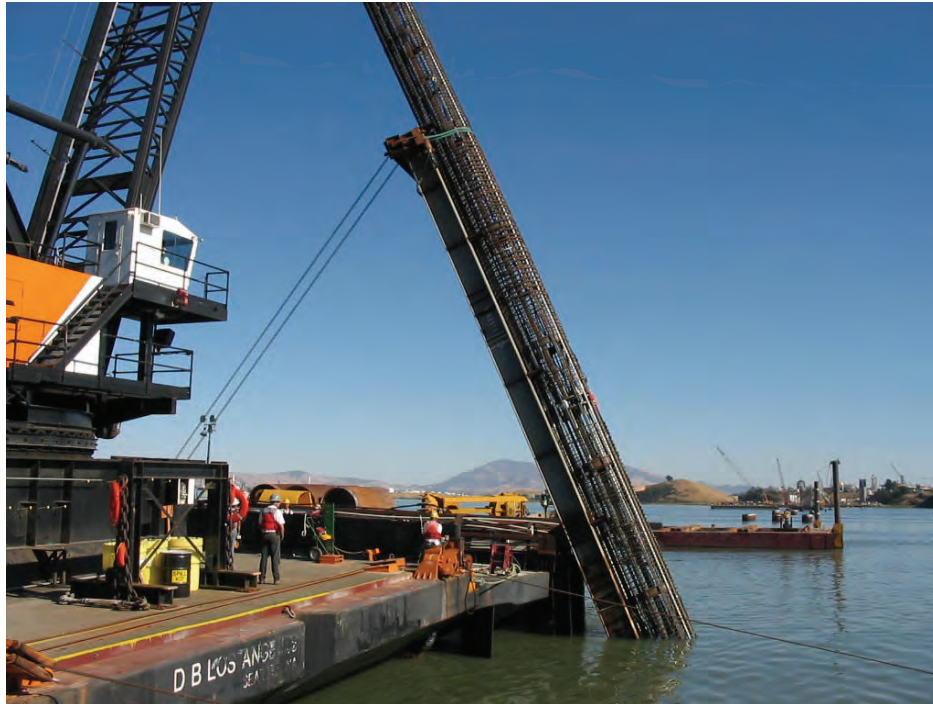
Figure 8-22 Photograph of Rebar Cage Being Lifted with a Tipping Frame (photo courtesy Malcolm Drilling)
