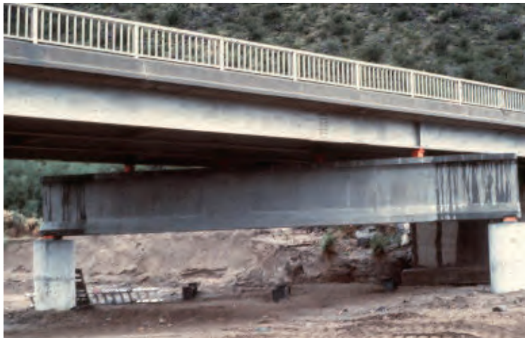
Figure 21-3 Use of Straddle Shafts to Replace an Existing Foundation (photo by B. Berkovitz)
