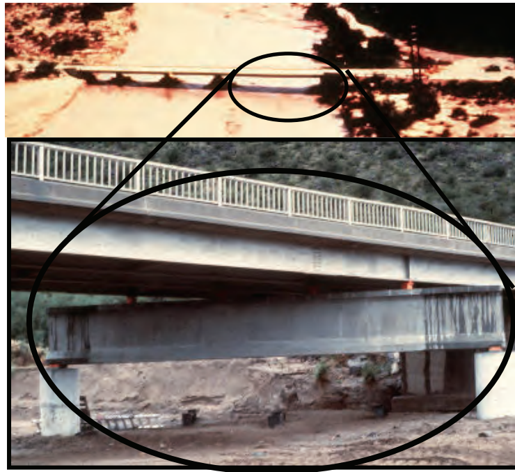
Figure 1-14 Drilled Shafts Installed for Deep Scour Problem
