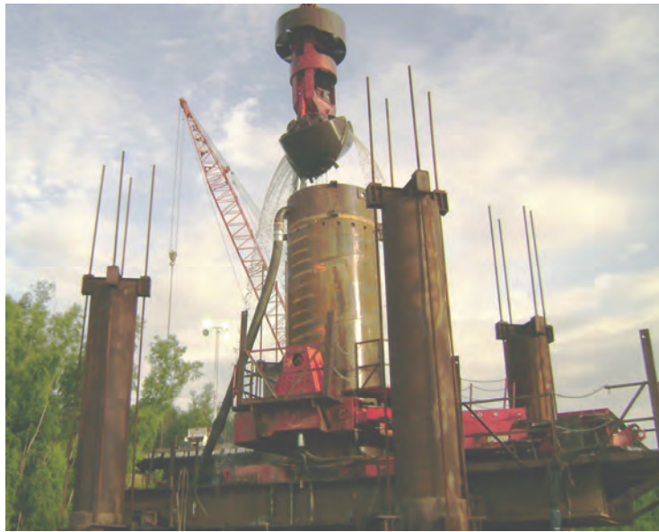
Figure 5-8 Oscillator Machine
