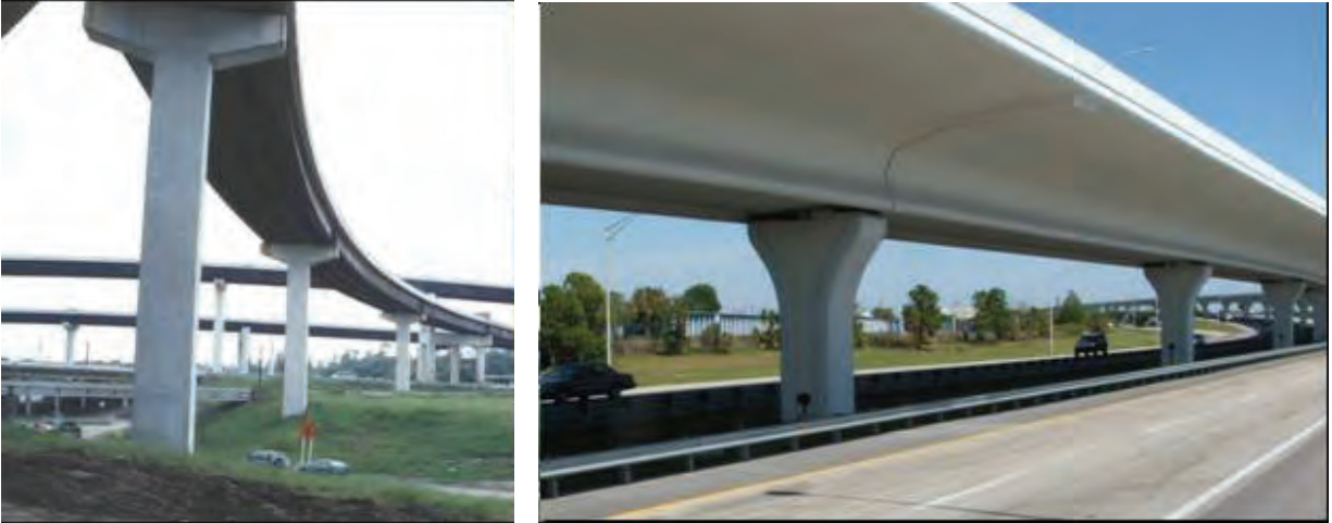
Figure 12-1 Single Column Piers with Monoshaft Foundations
