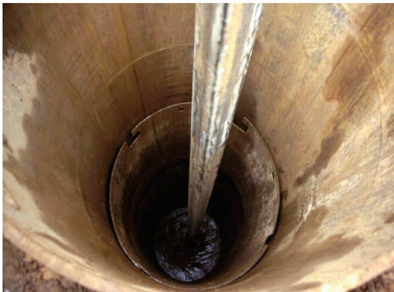
Figure 6-7 Use of Telescoping Casing
