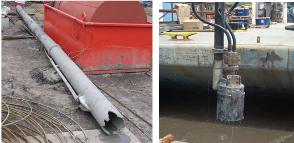
Figure 5-34 Airlift and Hydraulic Pumps for Shaft Base Cleanout
