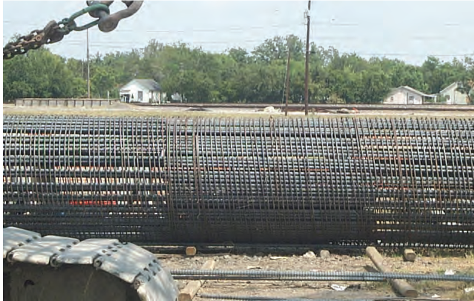
Figure 8-8 Constructability Problem from Excessive Concentration of Lap Splices
