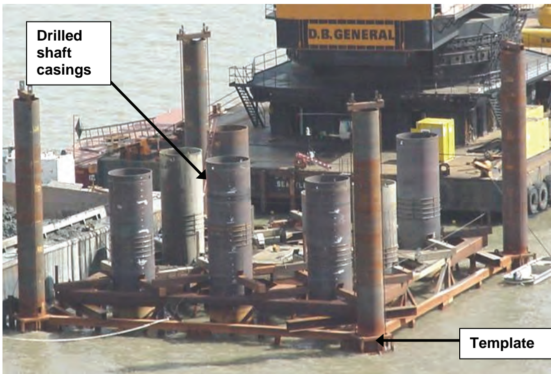
Figure 14-1 Group of Drilled Shafts During Construction of the Benetia-Martinez Bridge near San Francisco
