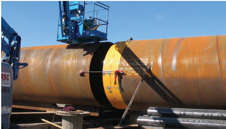
Figure 6-4 Installation of Casing Joint on Standard Pipe
