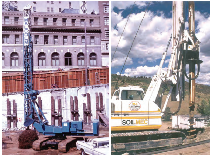
Figure 5-3 Mechanical (left) and Hydraulic (right) Powered Drilling Machines
