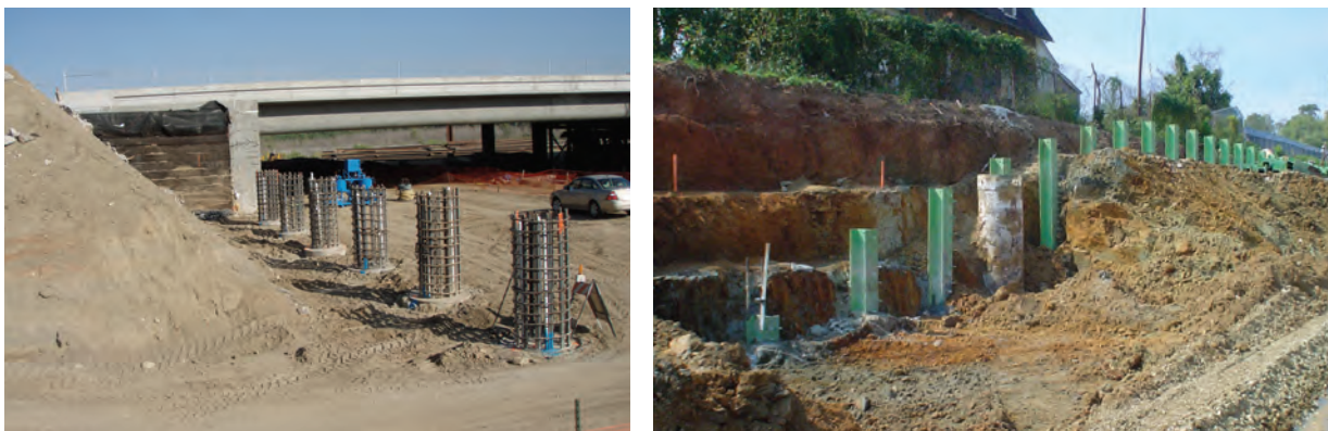
Figure 1-17 Drilled Shafts Used to Support Earth Retaining Structures
