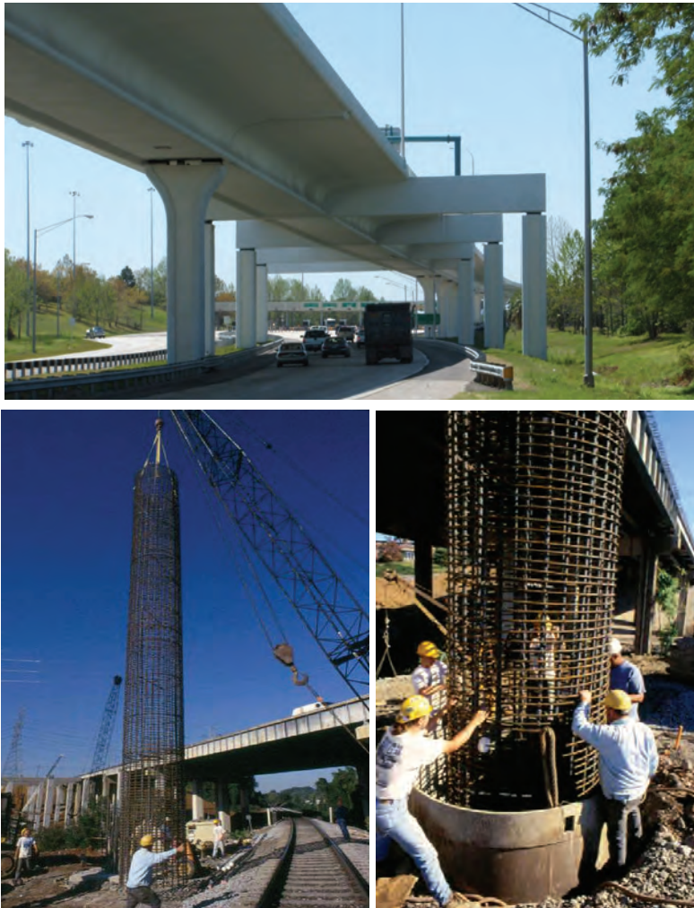
Figure 1-11 Drilled Shafts for Bridge Foundations where Small Footprint is Desirable
