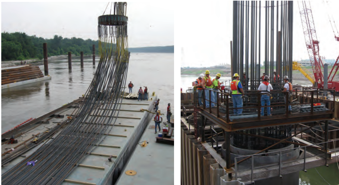
Figure 8-24 Photograph of Rebar Cage Being Assembled Over the Shaft Excavation
