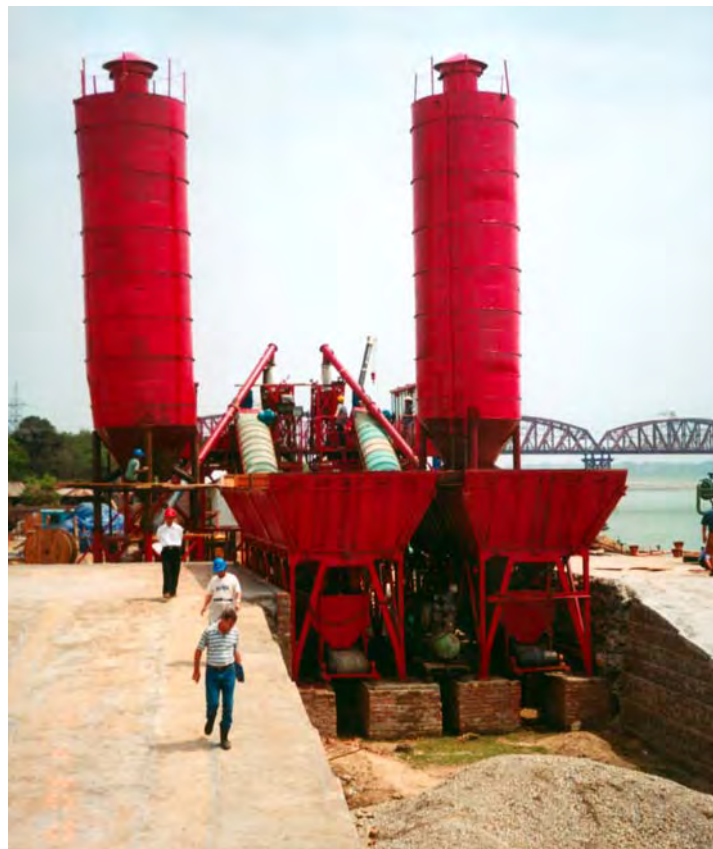
Figure 9-29 Worksite Concrete Batch Plant Capable of Batching 130 yd 3 /hr
