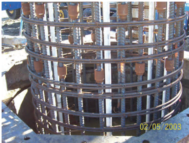
Figure 8-9 Bar Couplers Used to Construct Splices
