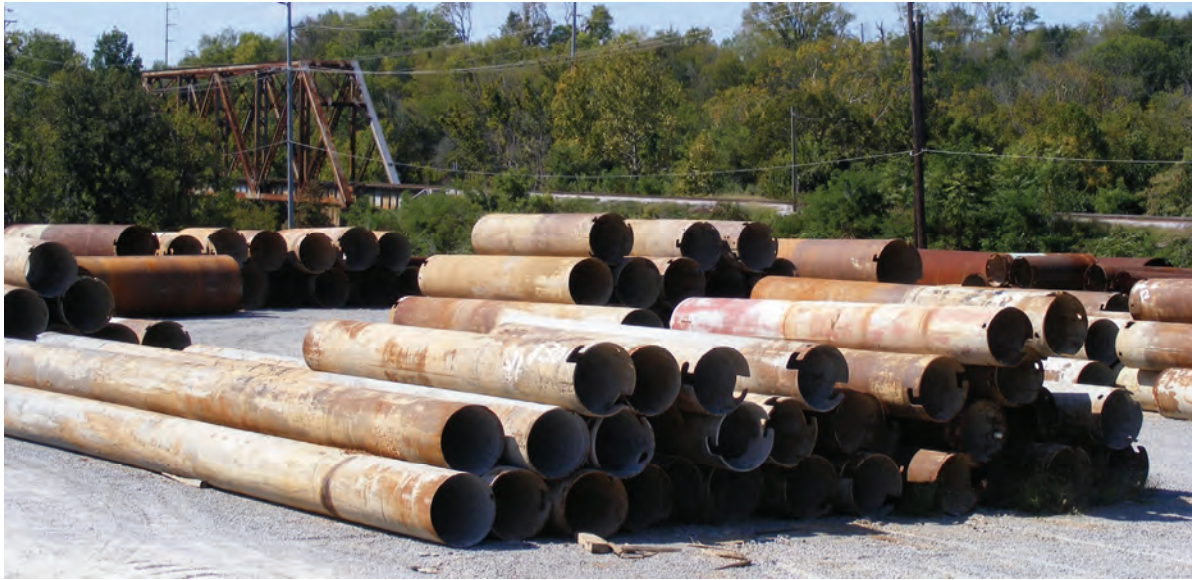
Figure 6-1 A Typical View of Stored Temporary Casing
