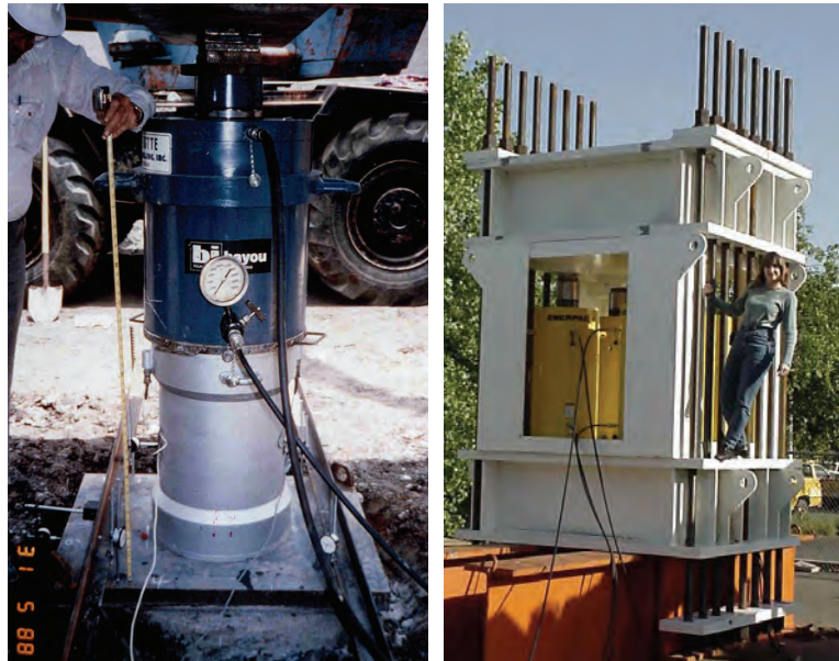
Figure 17-45 Hydraulic Jacks for Static Load Tests
