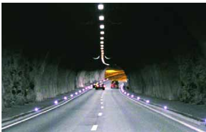
Figure 14. LED lights on roadway edges in the Grilstad Tunnel. (SINTEF).
