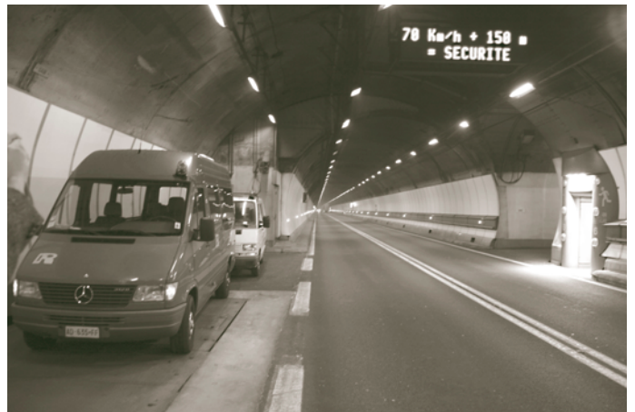
Figure 19. Emergency pullout area across from refuge room in the Mont Blanc Tunnel.
