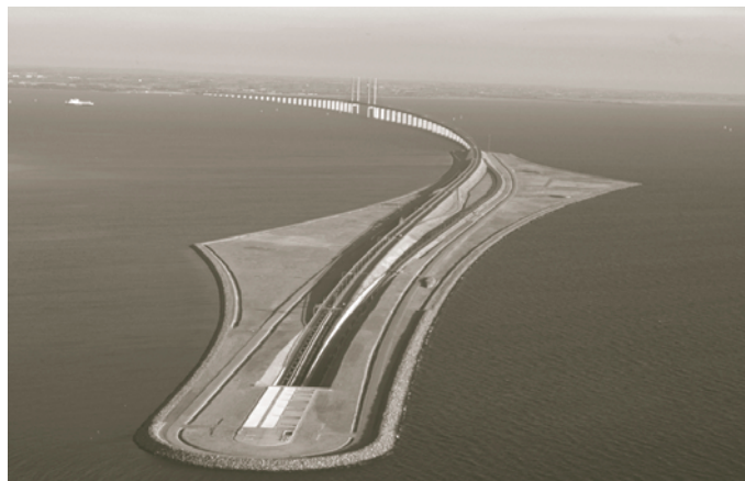
Figure 4. Oresund fixed link between Copenhagen, Denmark, and Malmo, Sweden. Shown is the island portal and bridge approach looking toward Sweden.
