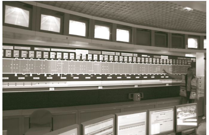
Figure 18. “One-button” response for incident management in the Mont Blanc Tunnel.
