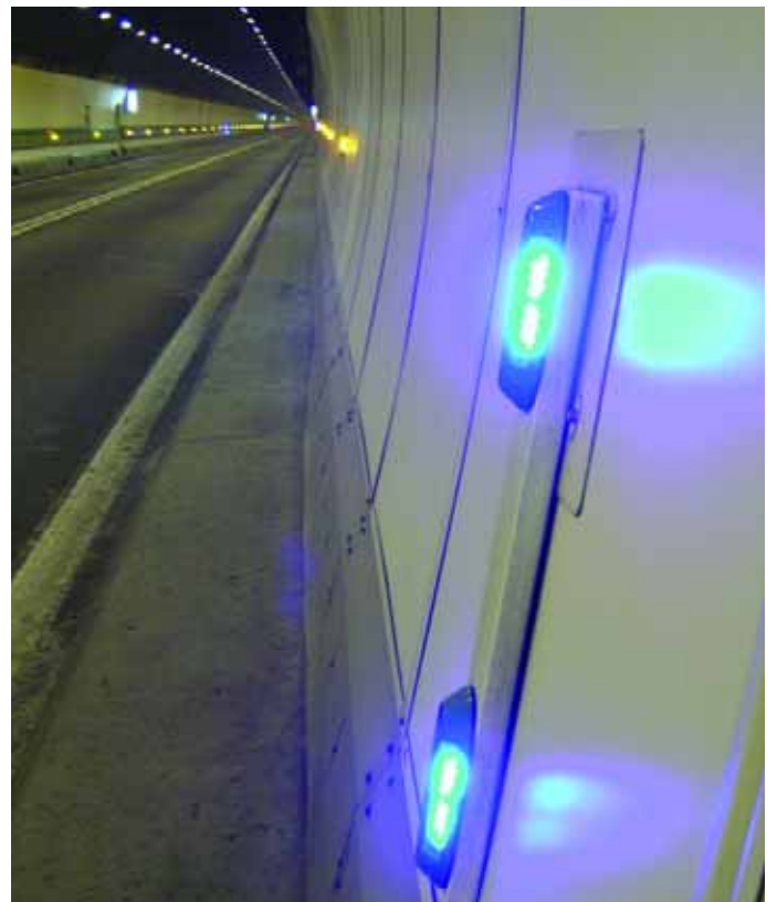
Figure 15. LED lights in the Mont Blanc Tunnel: yellow for edge delineation and blue for vehicle spacing.
