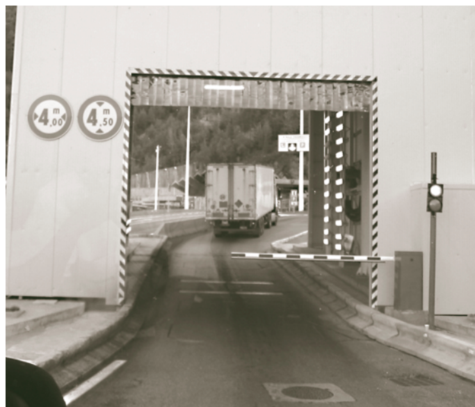
Figure 17. Truck thermal detector at the Mont Blanc Tunnel.
