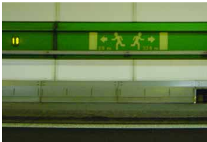
Figure 13. Examples from the Mont Blanc Tunnel. Top: tunnel escape route. Bottom: tunnel escape route sign.
