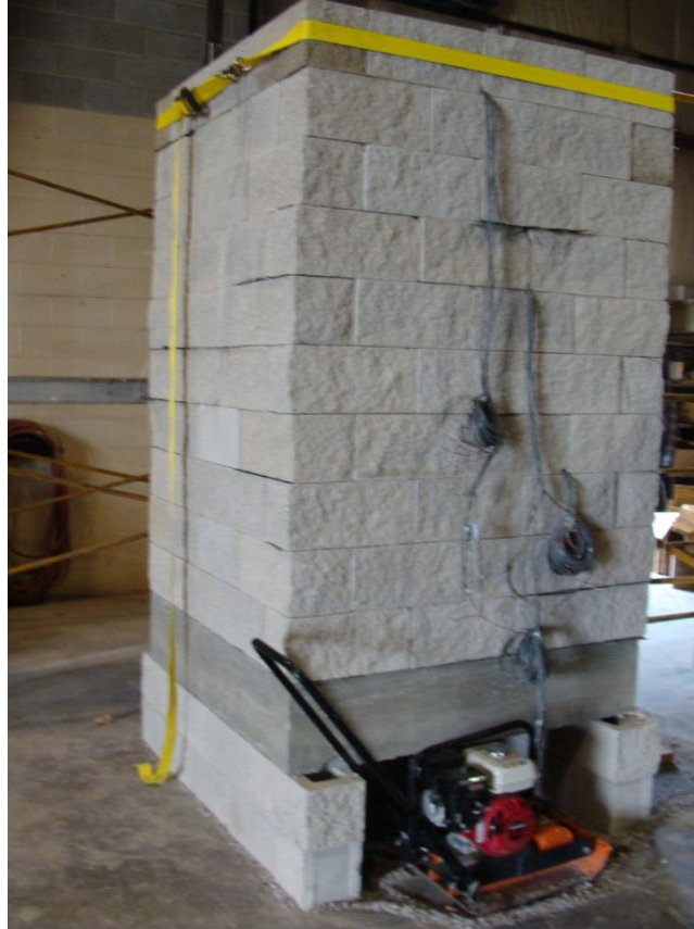
Figure 16. Photo. DC-1 GRS PT (before testing).
