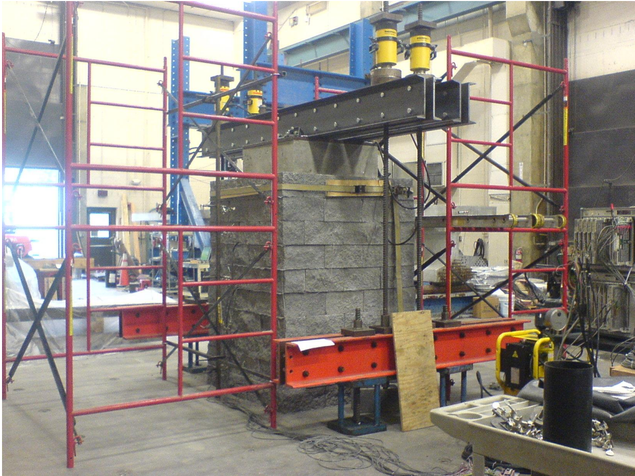
Figure 19. Photo. TF-1 PT setup with reaction frame.
