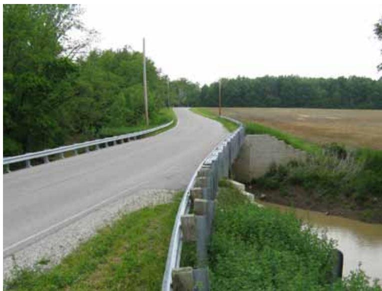
Figure 23. Photo. Bowman Road Bridge after 4.5 years.
