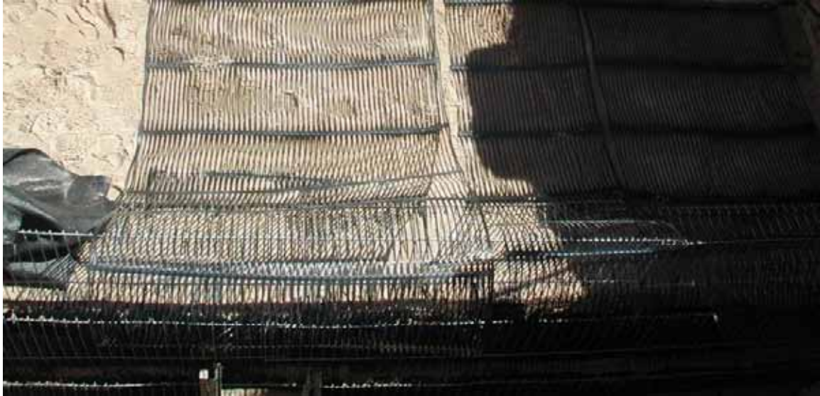
Figure 4. Photo. MSE extensible reinforcement (geogrid).
