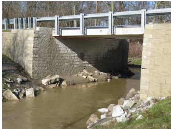
Figure 21. Photo. Huber Road Bridge.
