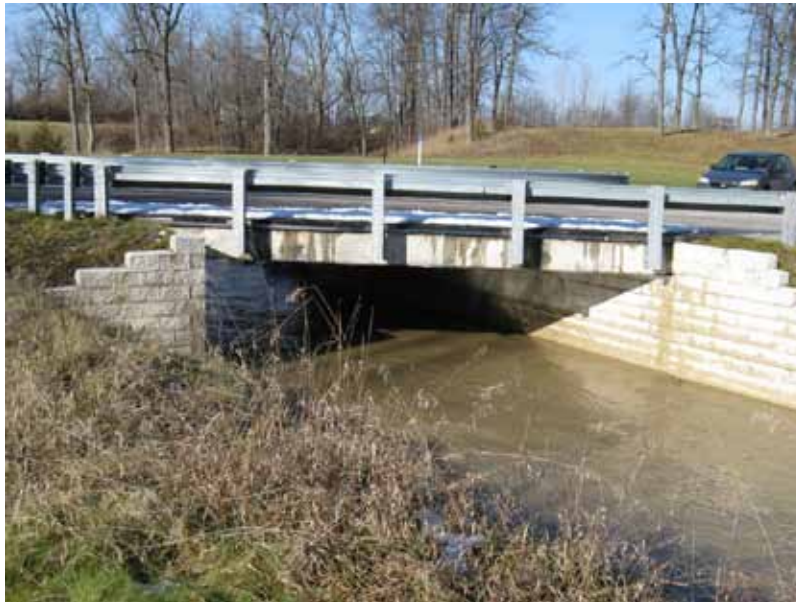
Figure 17. Photo. Vine Street Bridge.
