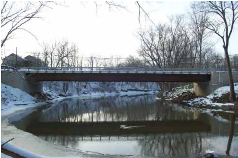
Figure 25. Photo. Tiffin River Bridge.
