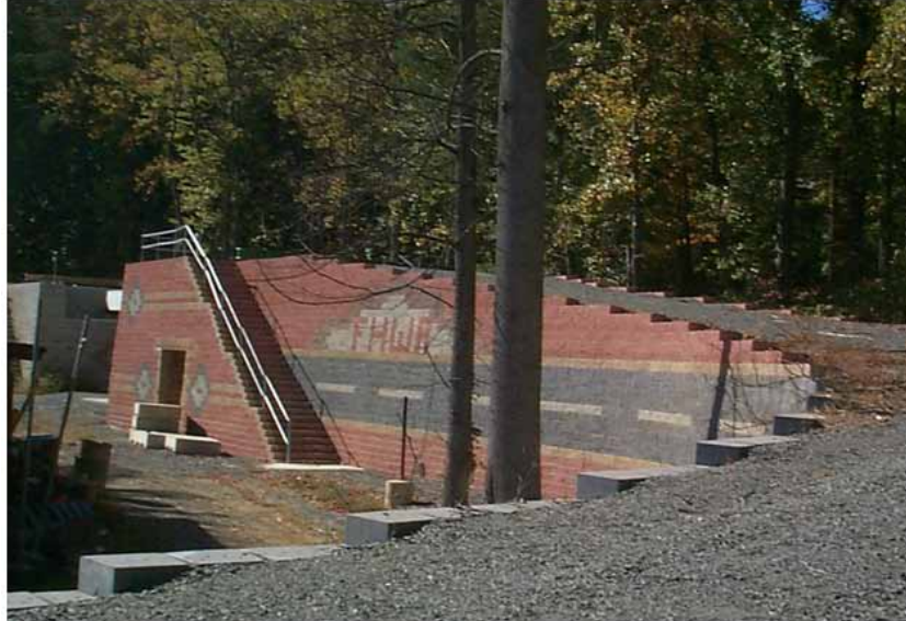
Figure 28. Photo. GRS-IBS tunnel at TFHRC.
