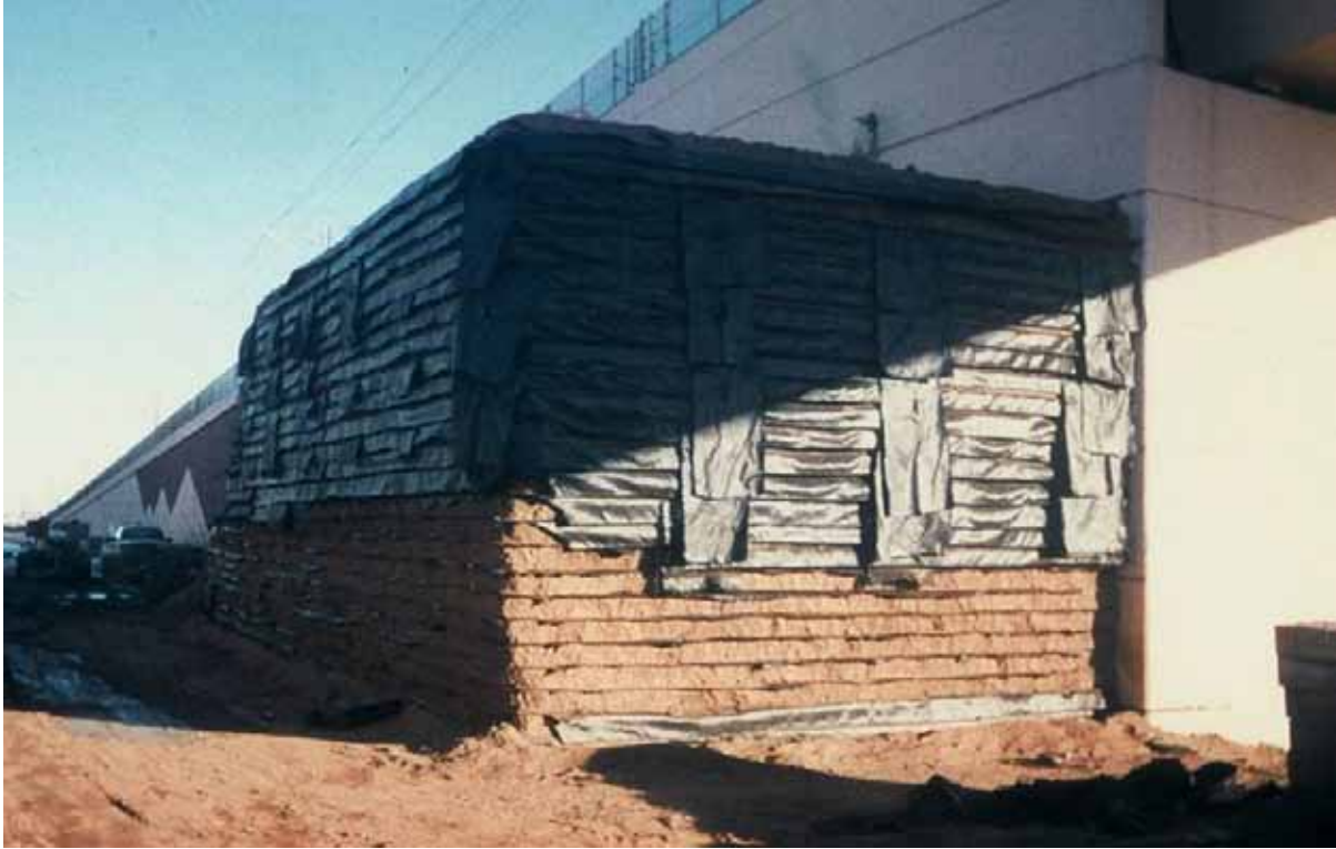
Figure 8. Photo. Internally supported GRS structure.
