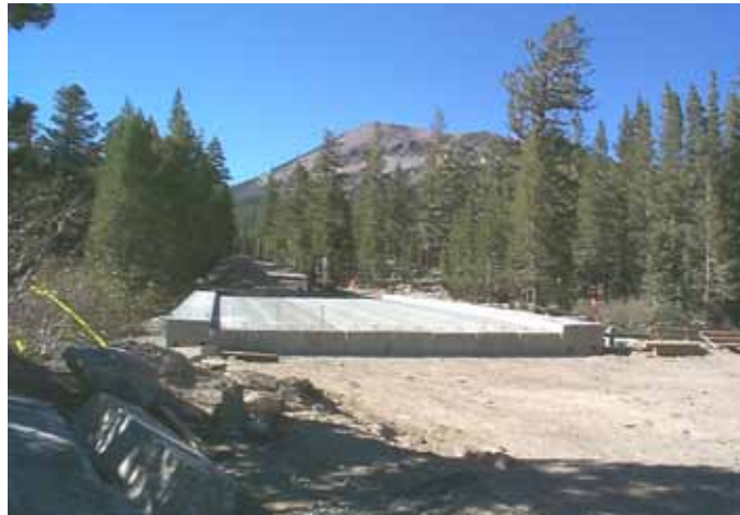
Figure 33. Photo. Concrete box bridge on GRS abutment in Mammoth Lake, CA.
