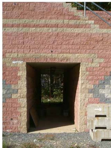
Figure 29. Photo. Close-up of GRS-IBS tunnel at TFHRC.
