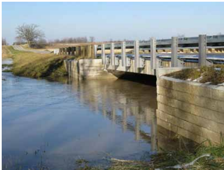
Figure 19. Photo. Glenburg Road Bridge under flood conditions.
