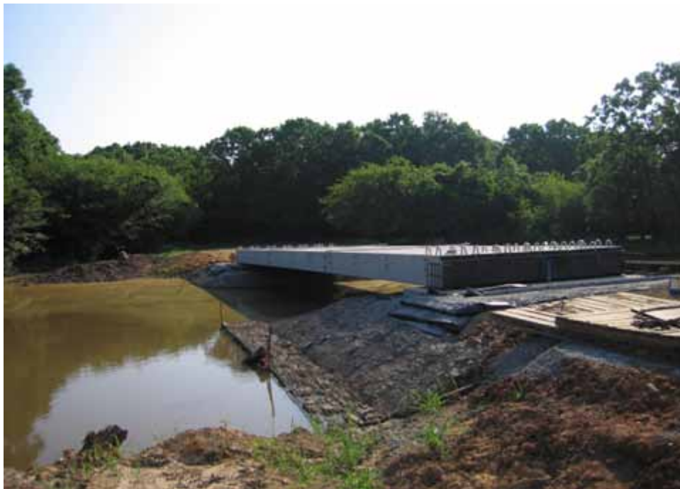
Figure 35. Photo. Concrete box bridge on GRS abutment in Ouachita wildlife refuge.
