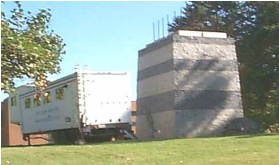
Figure 41. Photo. TFHRC pier test.
