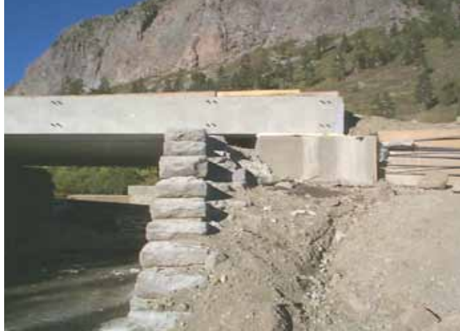
Figure 32. Photo. GRS abutment behind historic stone abutment.
