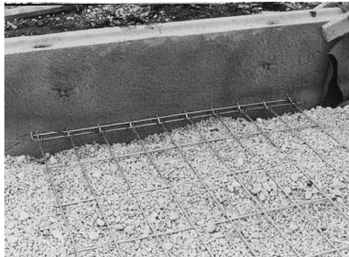
Figure 3. Photo. MSE inextensible reinforcement—wire mats. (3)
