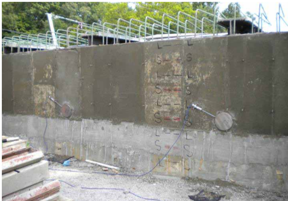
Figure 39. Photo. Pressure cells behind back wall on Tiffin River Bridge.
