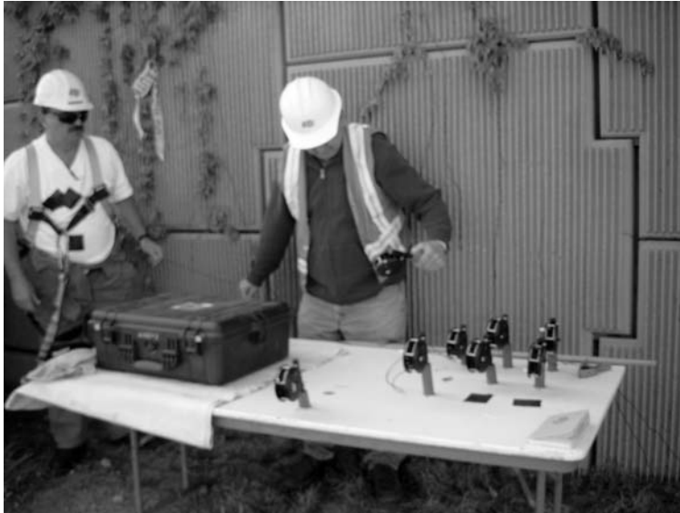
Figure 3-10. Junction platform and wire spools used to organize connections to inspection elements for electrochemical testing.
