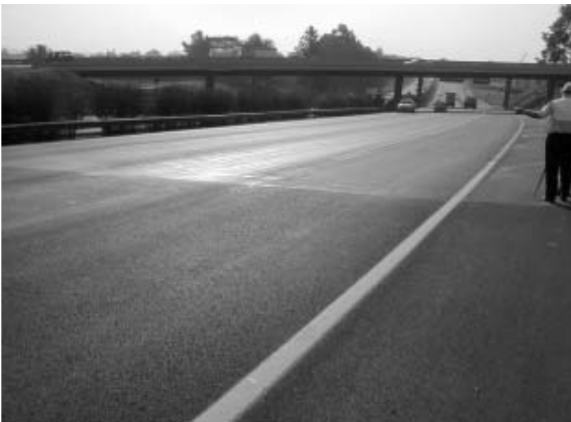
A surface treatment has been applied to this highway near Johannesburg, South Africa.
