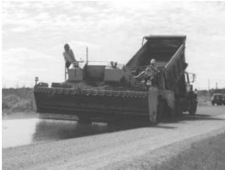
Preventive maintenance treatments, such as the chip seal shown here, can preserve the roadway and retard future deterioration.
