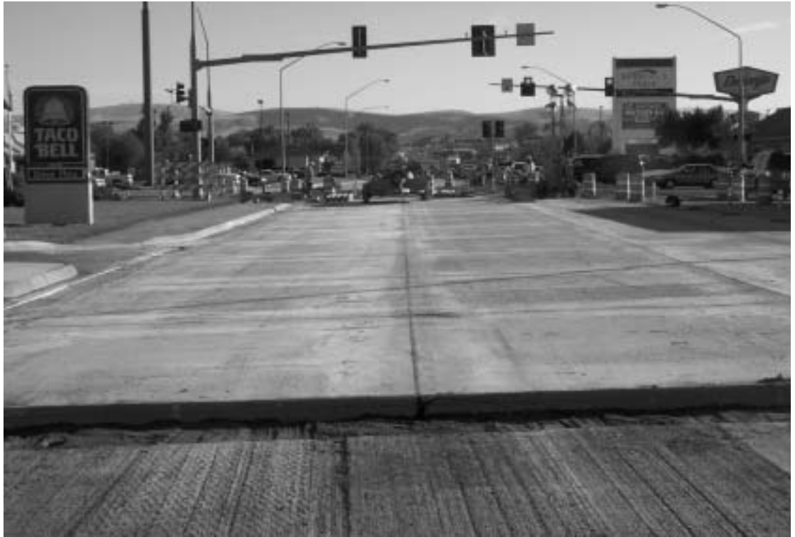
The three intersections were reconstructed with full depth concrete.
