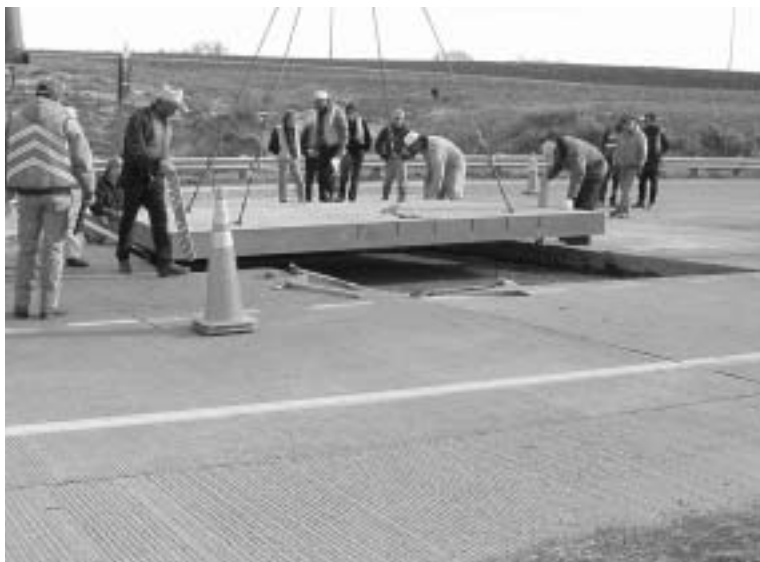
Full depth restoration is performed on US 287 near Fort Collins, Colorado, using precast concrete panels.
