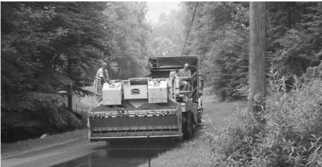
The North Carolina Department of Transportation places a chip seal, which is one of the pavement preservation practices covered in FHWA's new training courses.
