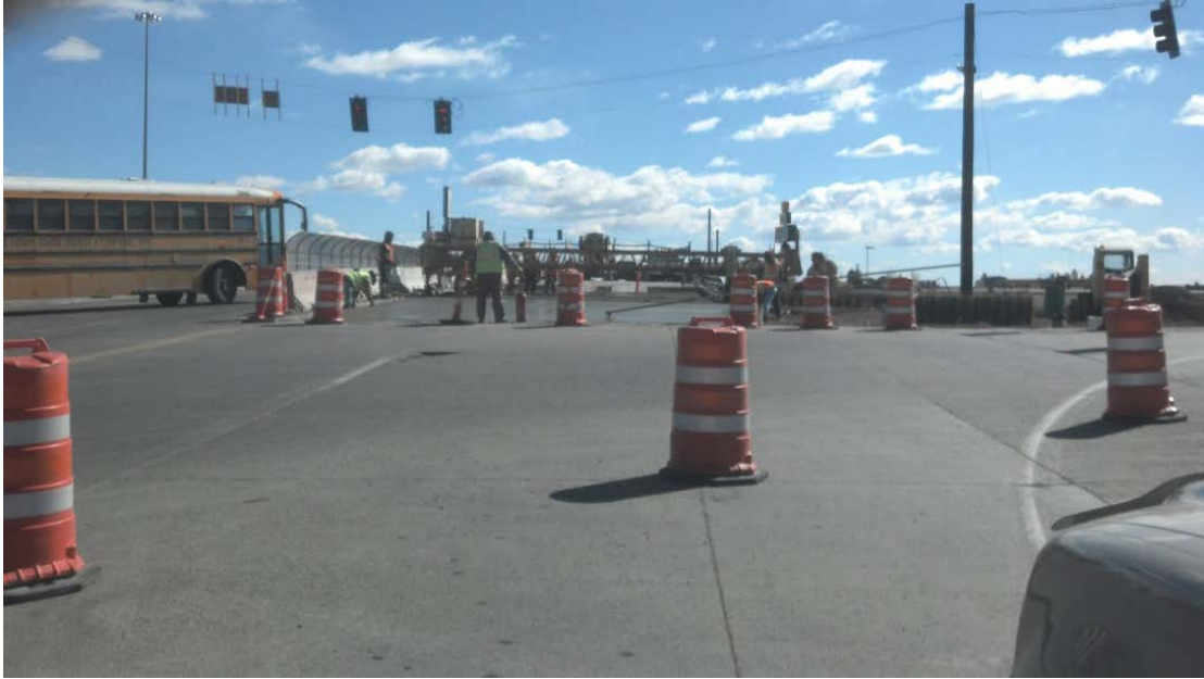
Figure 6. Photo. During construction, showing traffic still using the bridge.
