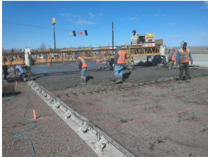
Figure 18. Photo. Concrete paving and dowel alignment during construction.
