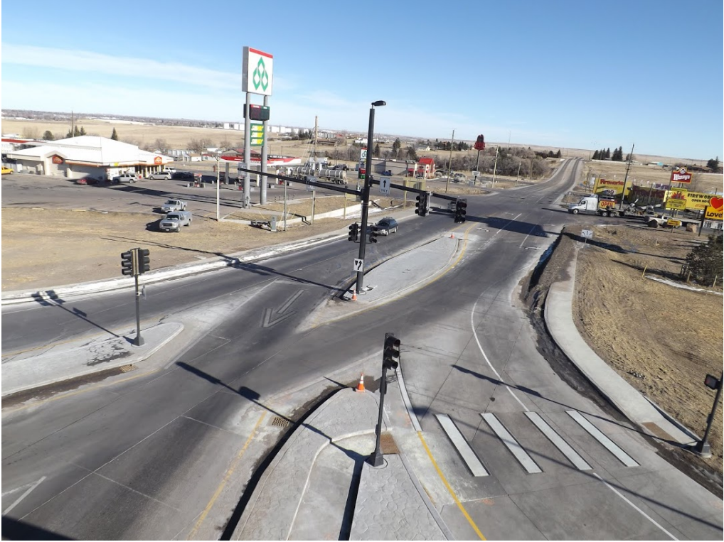
Figure 8. Photo. Arrows were painted on the roadway to help guide drivers.
