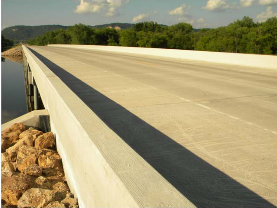
Figure 14. Finished deck of bridge #3.
