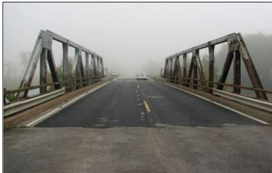
Figure 2. The pony truss bridge #1 prior to reconstruction.
