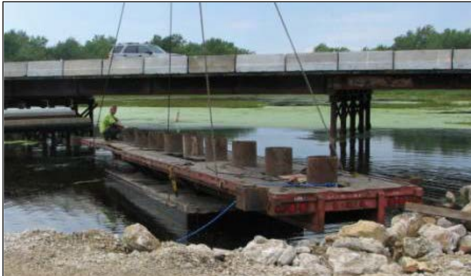
Figure 10. Template for driving the steel piles (source: WisDOT).
