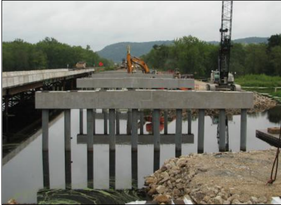
Figure 8. Open pile bent during construction at bridge #3 (source: WisDOT).
