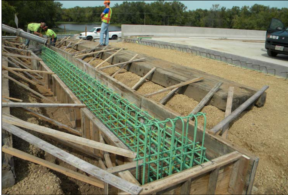
Figure 17. Formwork and reinforcing steel for the approach apron footing and header.
