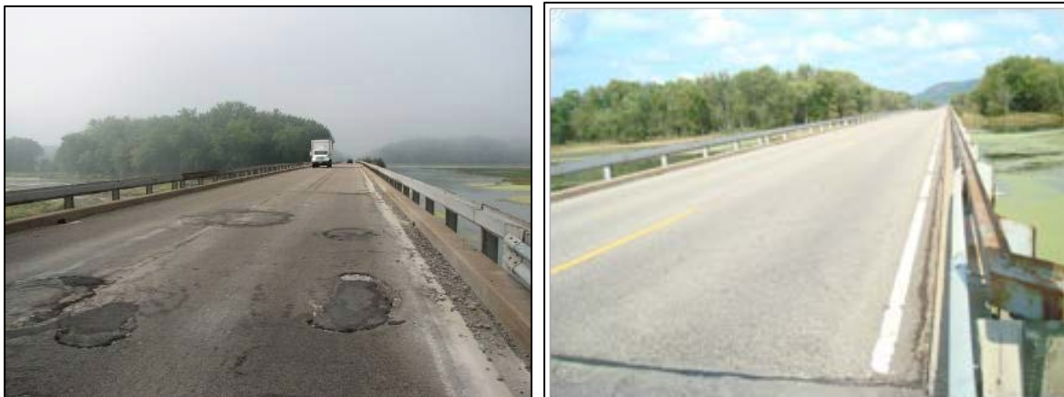
Figure 4. Existing bridge #3 (left) and existing bridge #4 (right).
