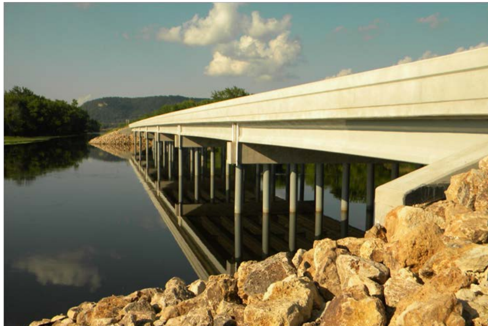
Figure 9. Finished open pile bents at bridge #3.
