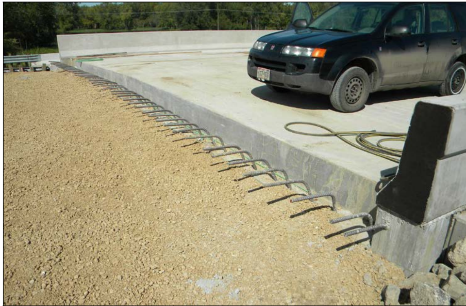
Figure 16. Stainless steel reinforcing extending out of the abutment.
