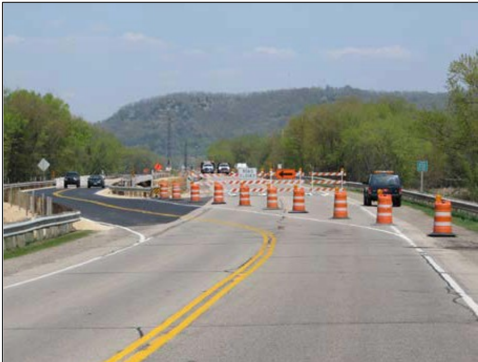
Figure 6. Temporary bypass bridge in use at bridge #3.
