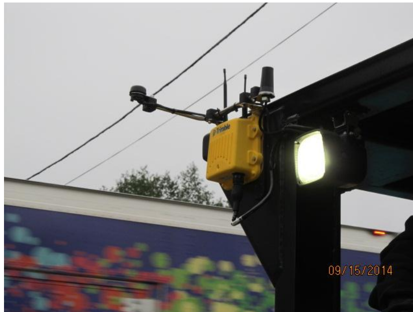
Figure 5. Photo. IC GPS and radio receiver mounted to paving roller Cat CB54 XW. (courtesy: Vermont Agency of Transportation)
