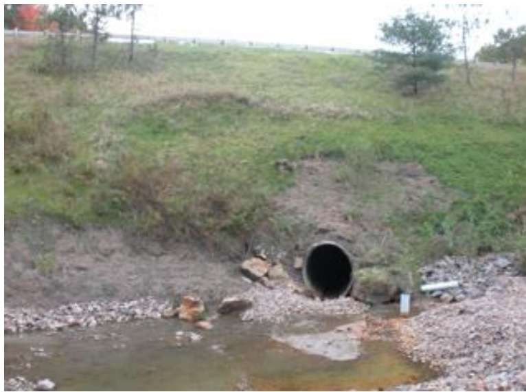
Figure 1 – Culvert Location Relative to Crest of Embankment
