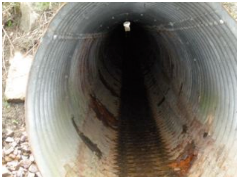
Figure 2 – Typical Condition of Existing Culverts
