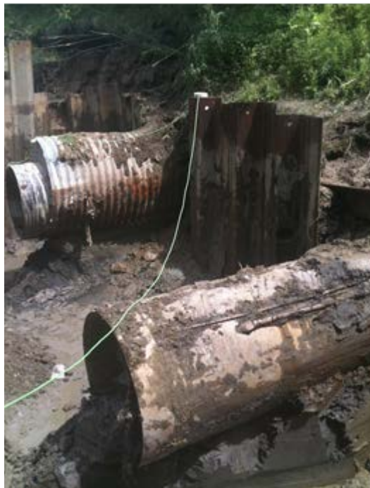
Figure 5 – Steel Casing and Existing Culvert with Liner
