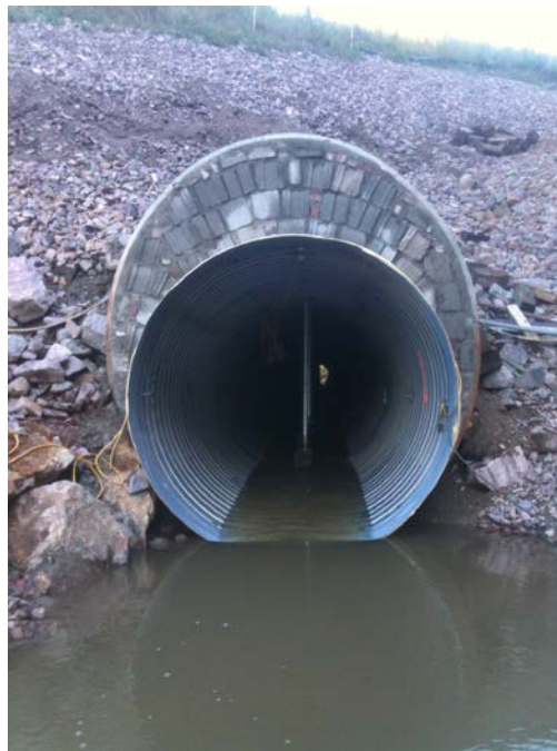
Figure 4 – End View of Slip Liner at Colchester Site
