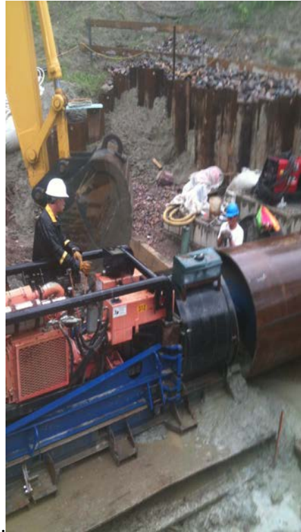
Figure 17. Auger bit removing the spoils from 24-in casing.
