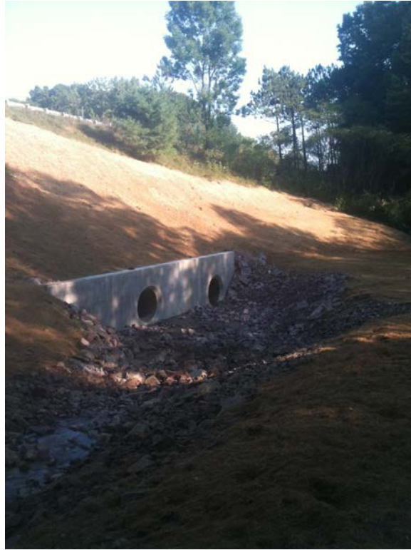
Figure 6 – Headwall with two openings.
