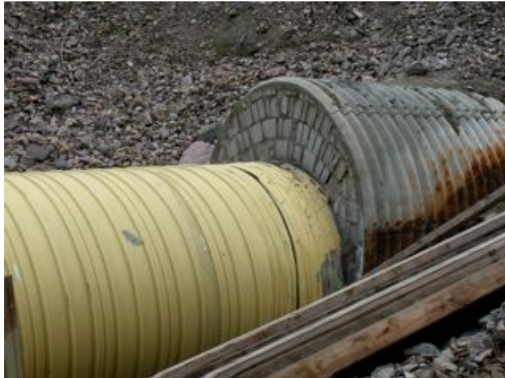
Figure 3 - Slip Liner in Existing Culvert at Colchester site
