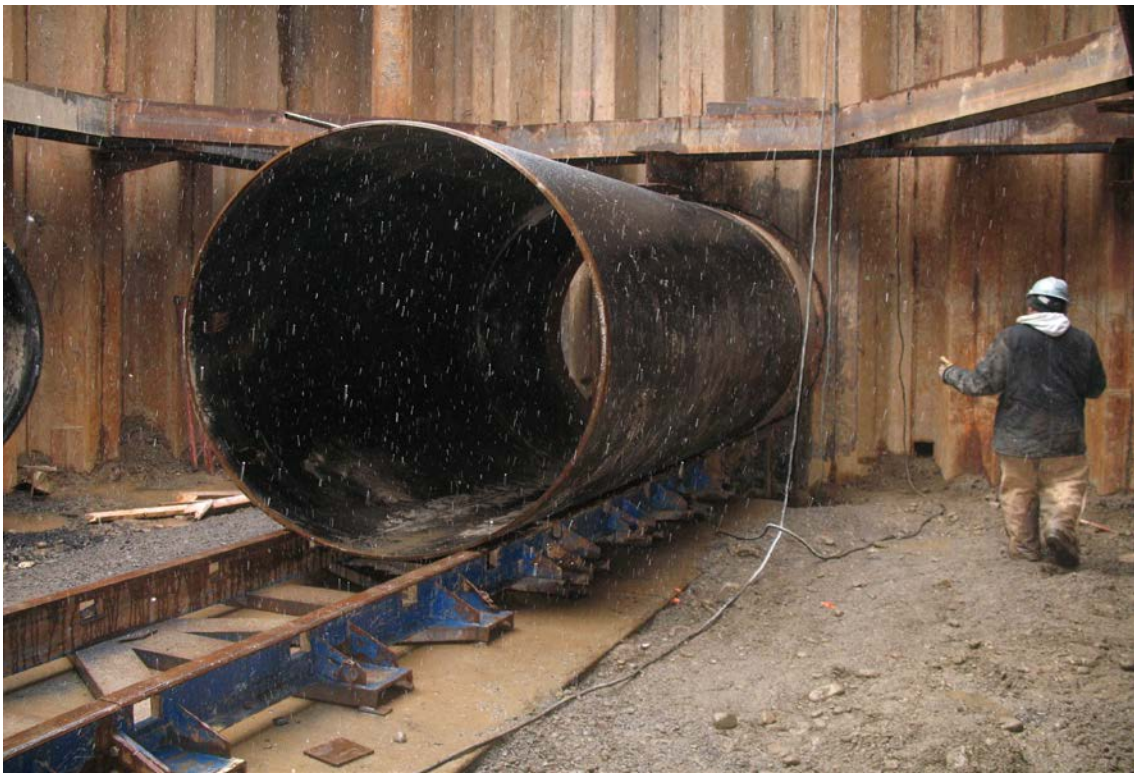
Figure 19. View of 60-in steel casing on guide rails.
