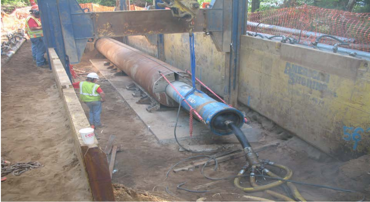
Figure 15. Ramming of pipe using Grundrum Koloss hammer.
