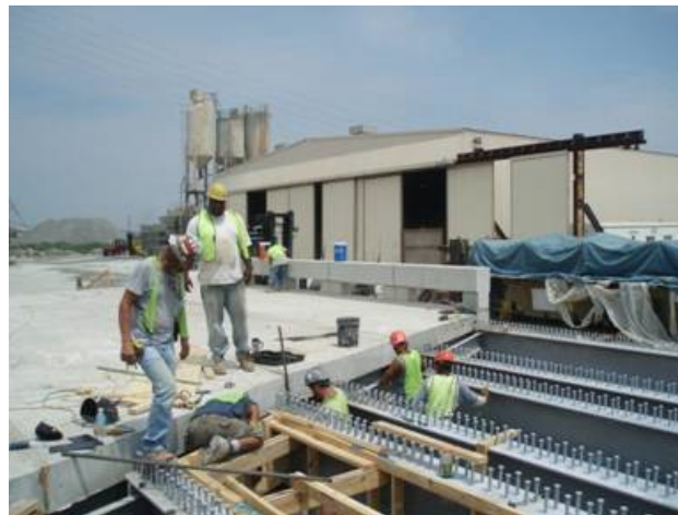
Figure 5. Steel beams for U.S. 15/29 bridge at Coastal Precast Systems precasting yard.
