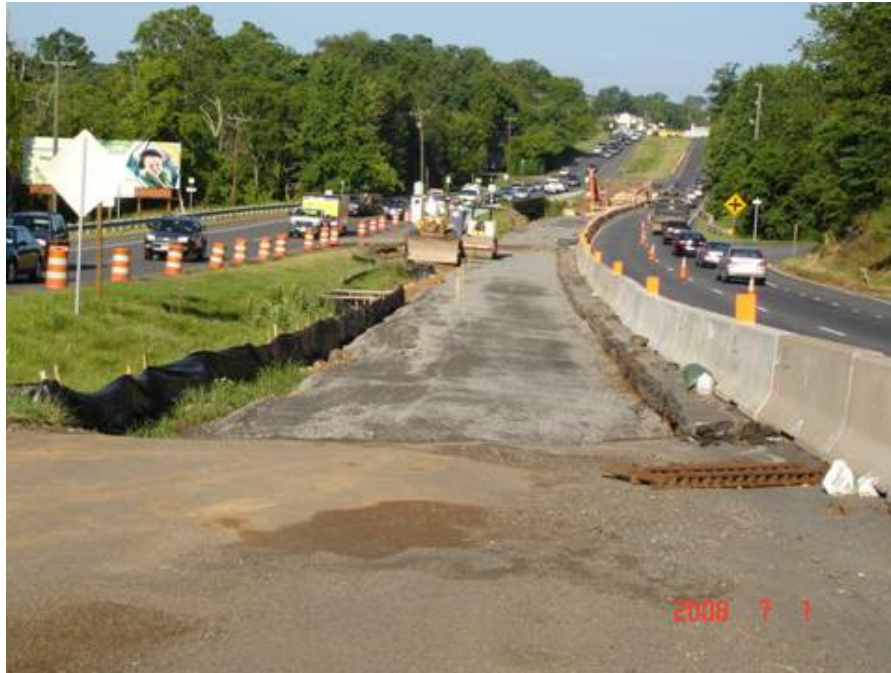
Figure 11. U.S. 15/29 bridge approach pavement preparation, looking south toward the bridge.
