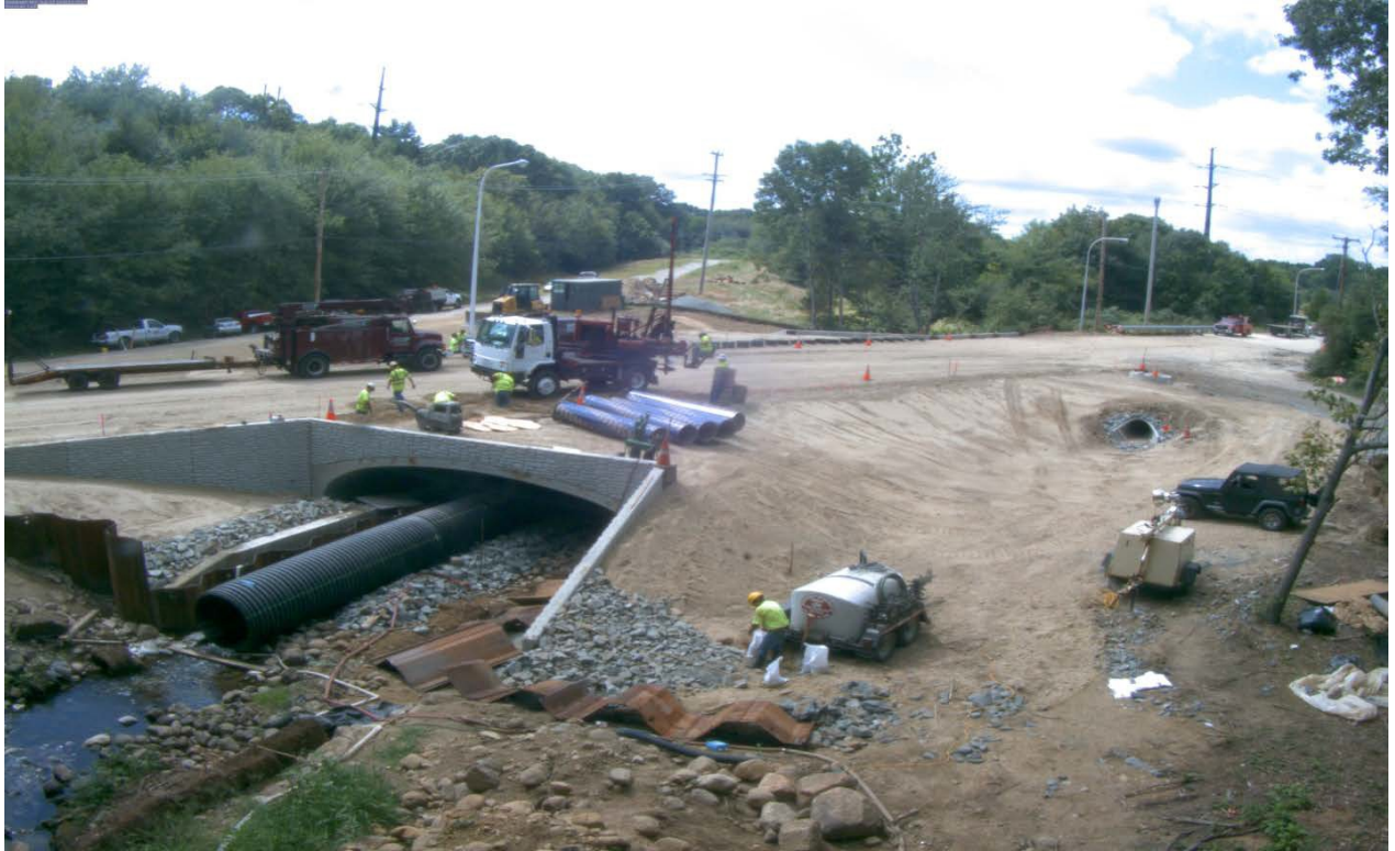
Figure 27. Gravel backfill being rolled into place.
