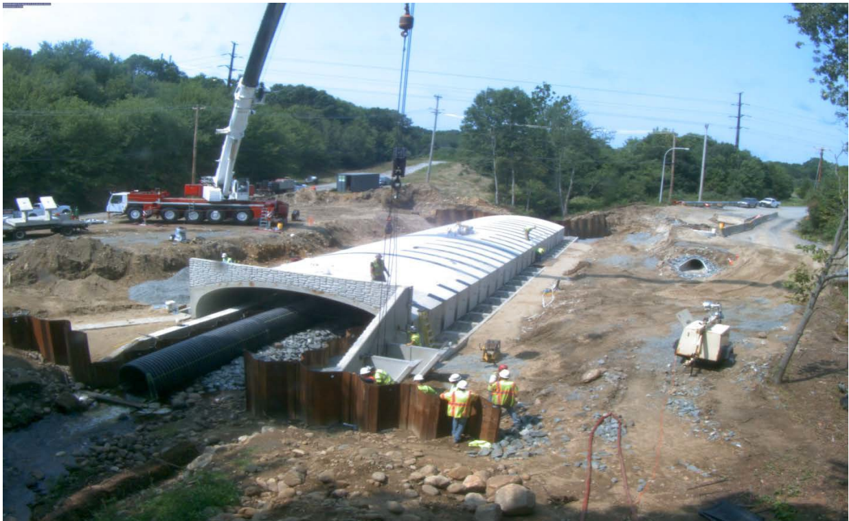
Figure 20. Modular wingwall being lowered into place.
