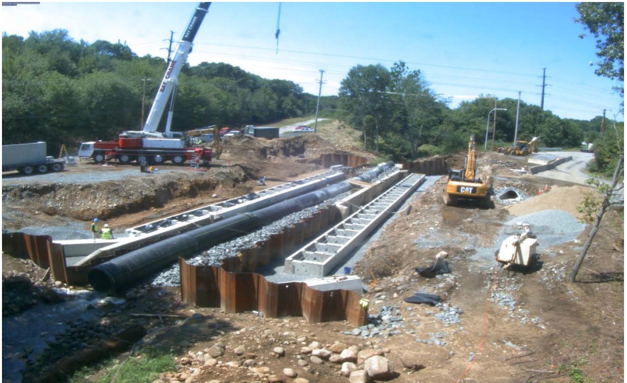
Figure 14. Modular prefabricated footings in place.
