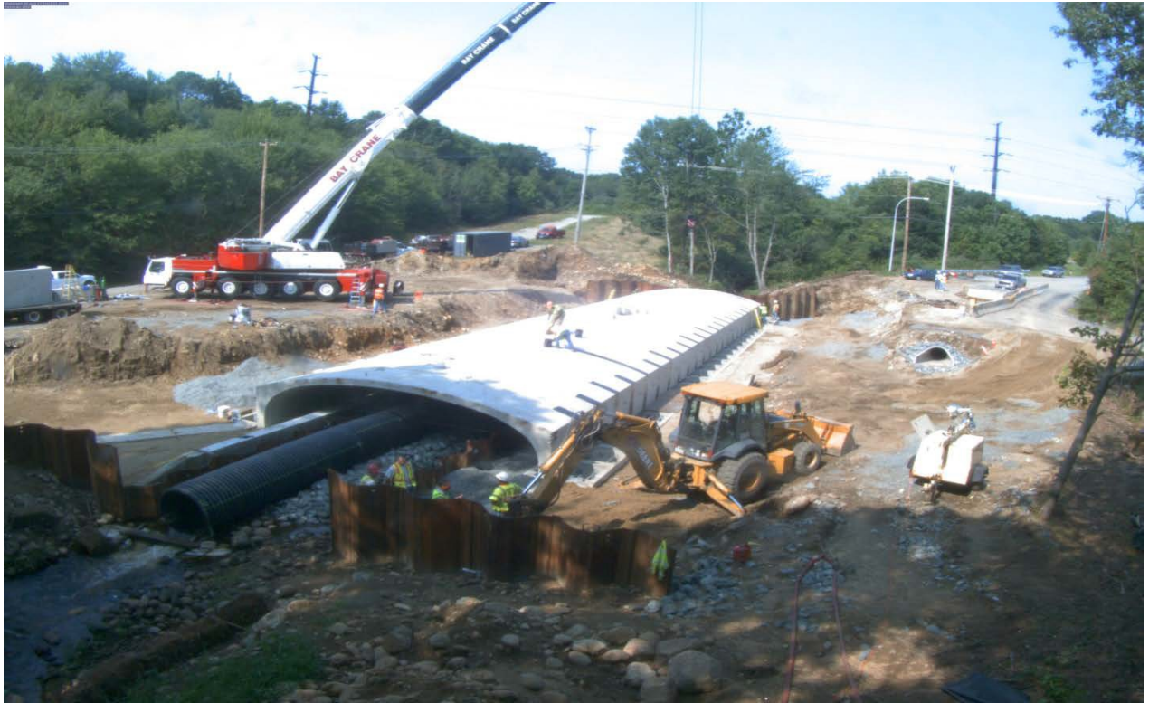
Figure 17. All 25 main bridge elements lowered into place.
