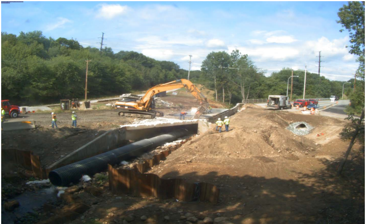
Figure 7. Demolition of old structure in process with stream diversion in place.
