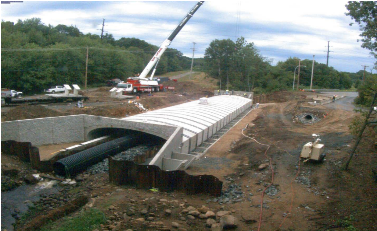
Figure 22. Far end headwall being lowered into place.
