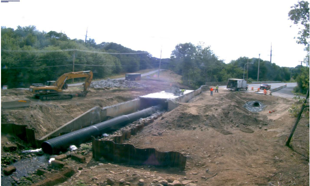
Figure 8. Demolition showing slab removal with abutment walls left in place.
