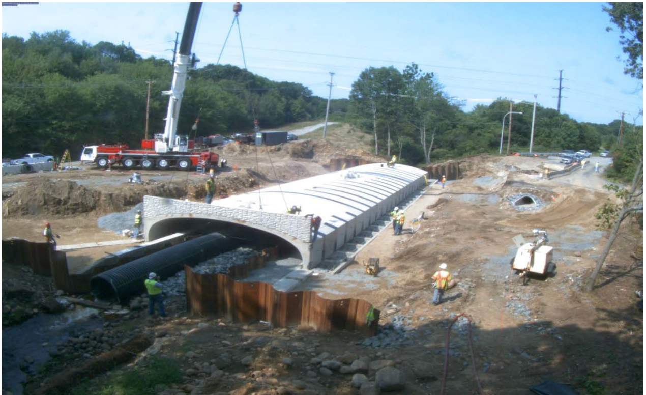
Figure 18. Modular headwall being lowered into place.
