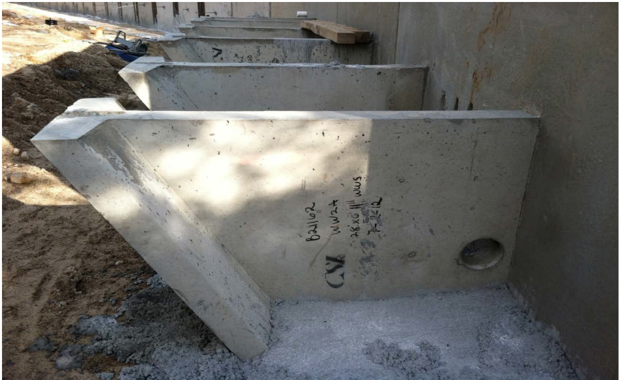
Figure 24. Closeup of wingwall anchors.
