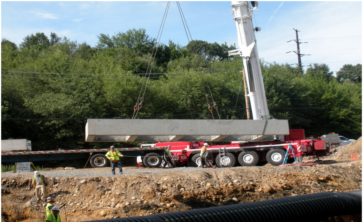
Figure 12. Precast foundation units being lifted off tractor-trailer.
