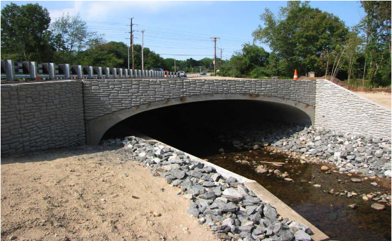
Figure 30. Completed structure with guardrail and riprap in place.
