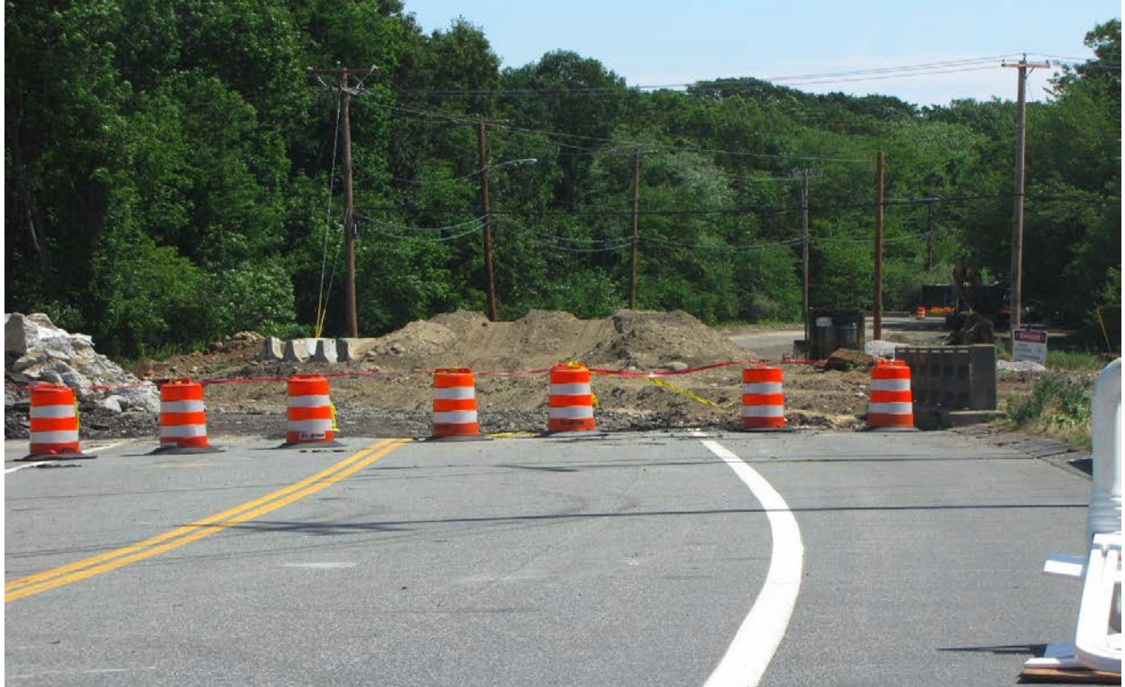
Figure 6. Closure of Davisville Road.
