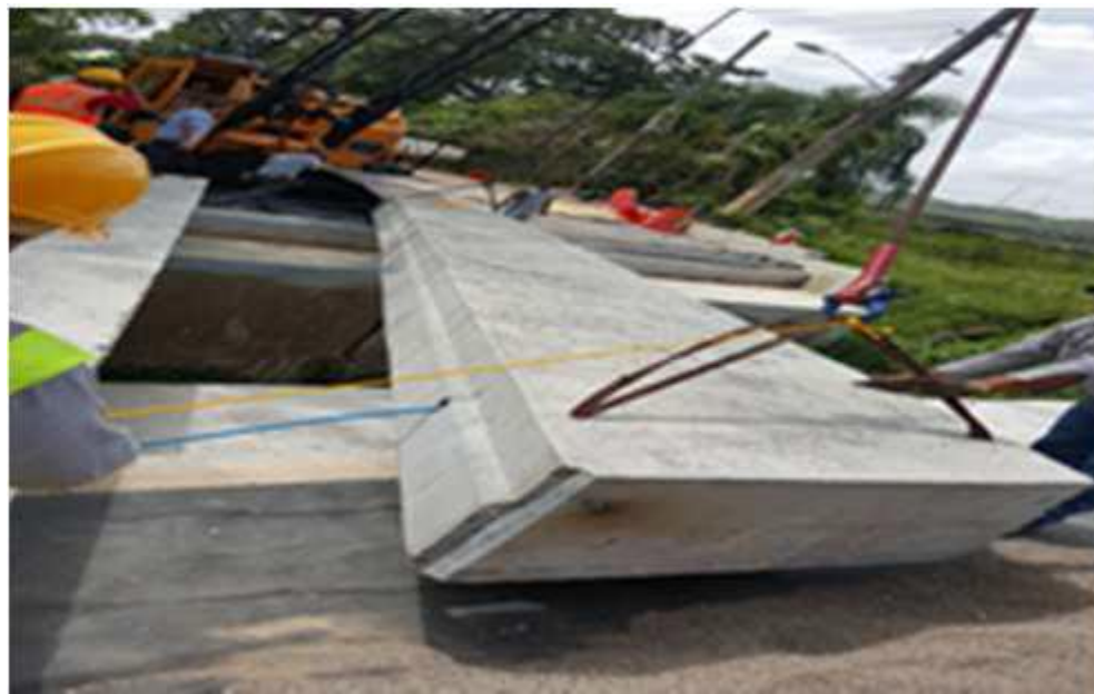
Figure 10. Photo. Installation of pre-stressed void slab.
