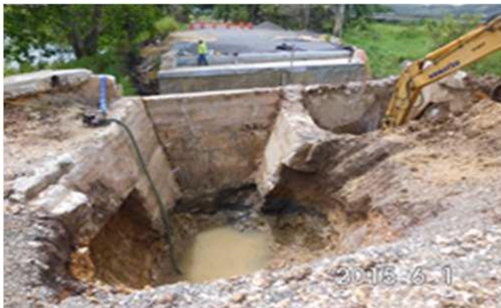
Figure 8. Photo. Excavation of west abutment.
