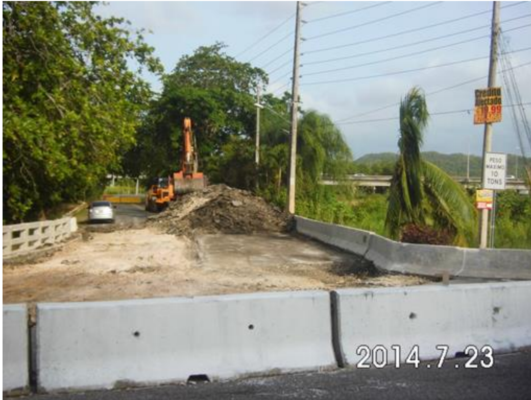
Figure 3. Photo. Existing Bridge No. 1828 on PR-140.
