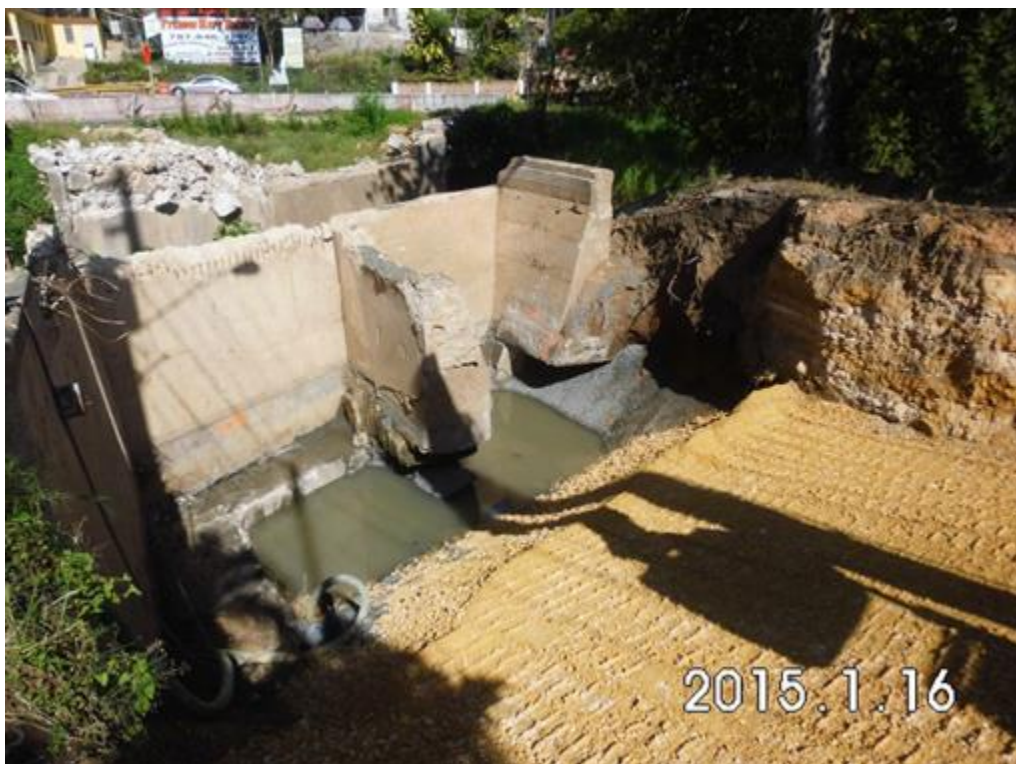
Figure 6. Photo. Excavation of east abutment.
