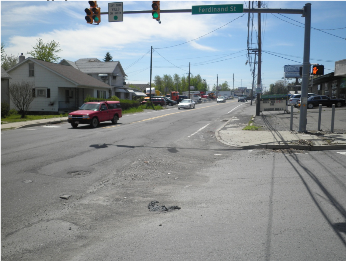
STA 549+50 Looking southbound from Ferdinand Street
