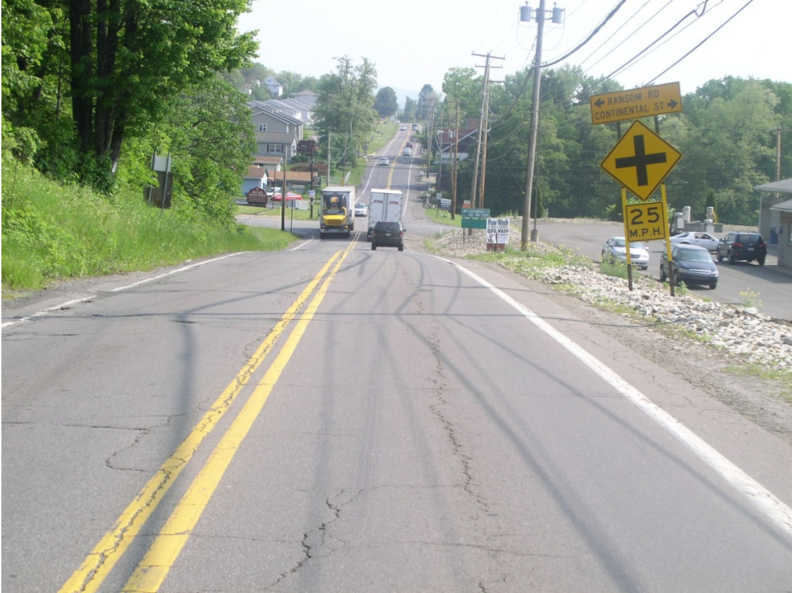
STA 400+00 Looking northbound toward Continental Street
