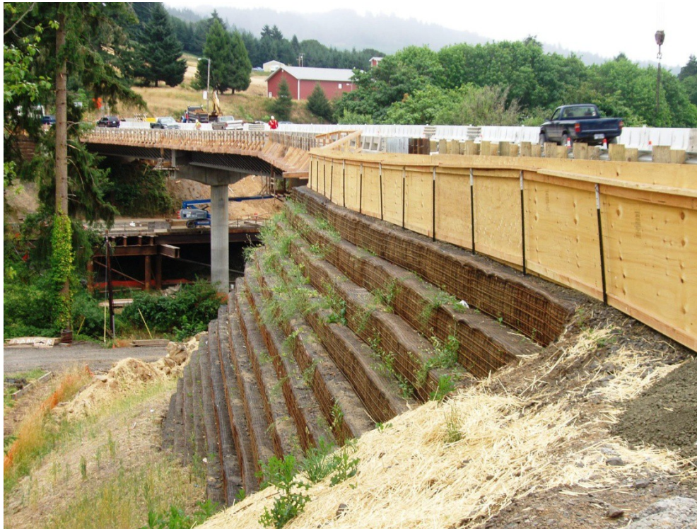
Figure 10. View of stepped-down geogrid system at crossing 1.
