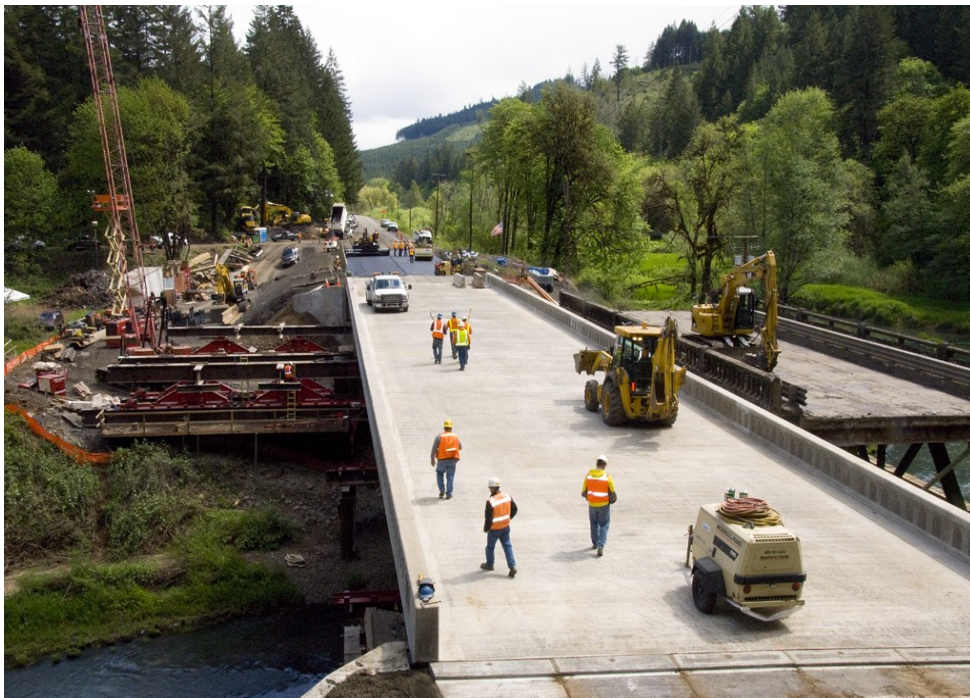
Figure 22. Replacement of superstructure and end panels at crossing 3.
