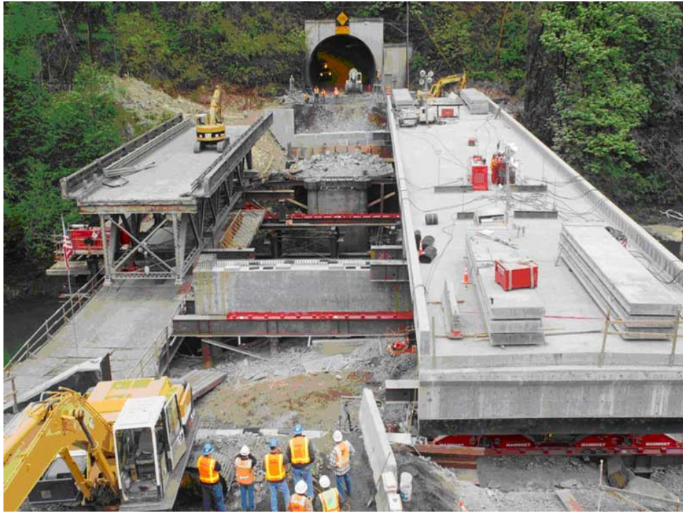
Figure 21. View of old and new superstructures at crossing 3.
