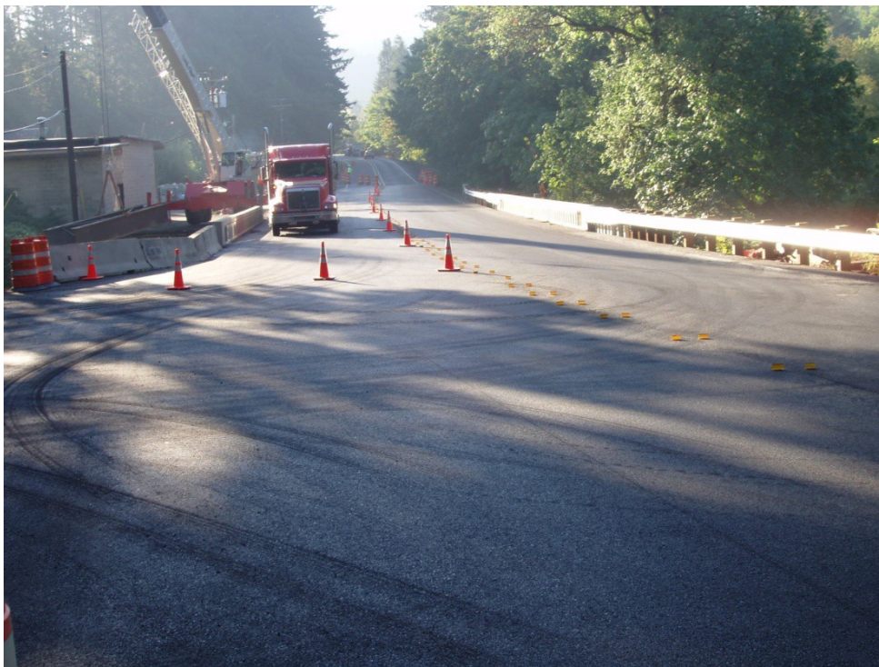
Figure 27. View of completed crossing 5 and dismantling of the detour bridge.
