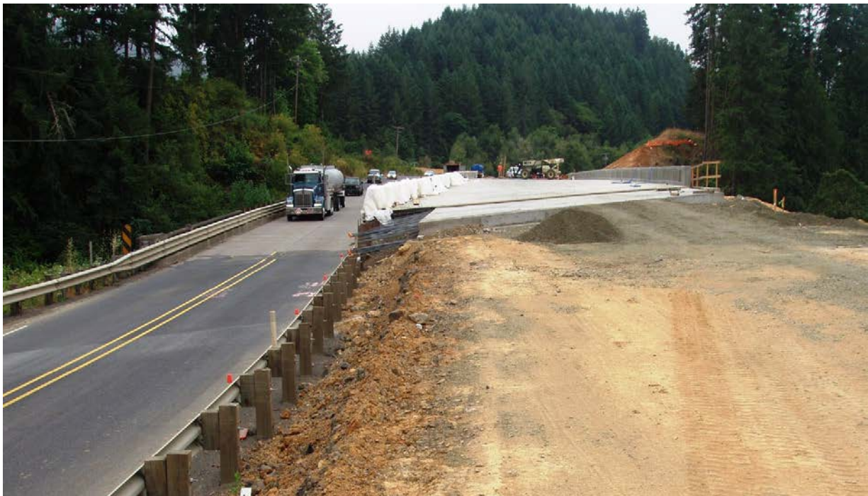
Figure 13. View of old and new crossing 2 looking west.
