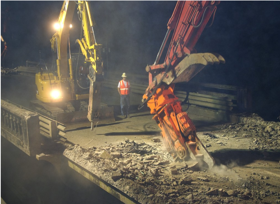
Figure 20. Demolition and dismantling of end panels.
