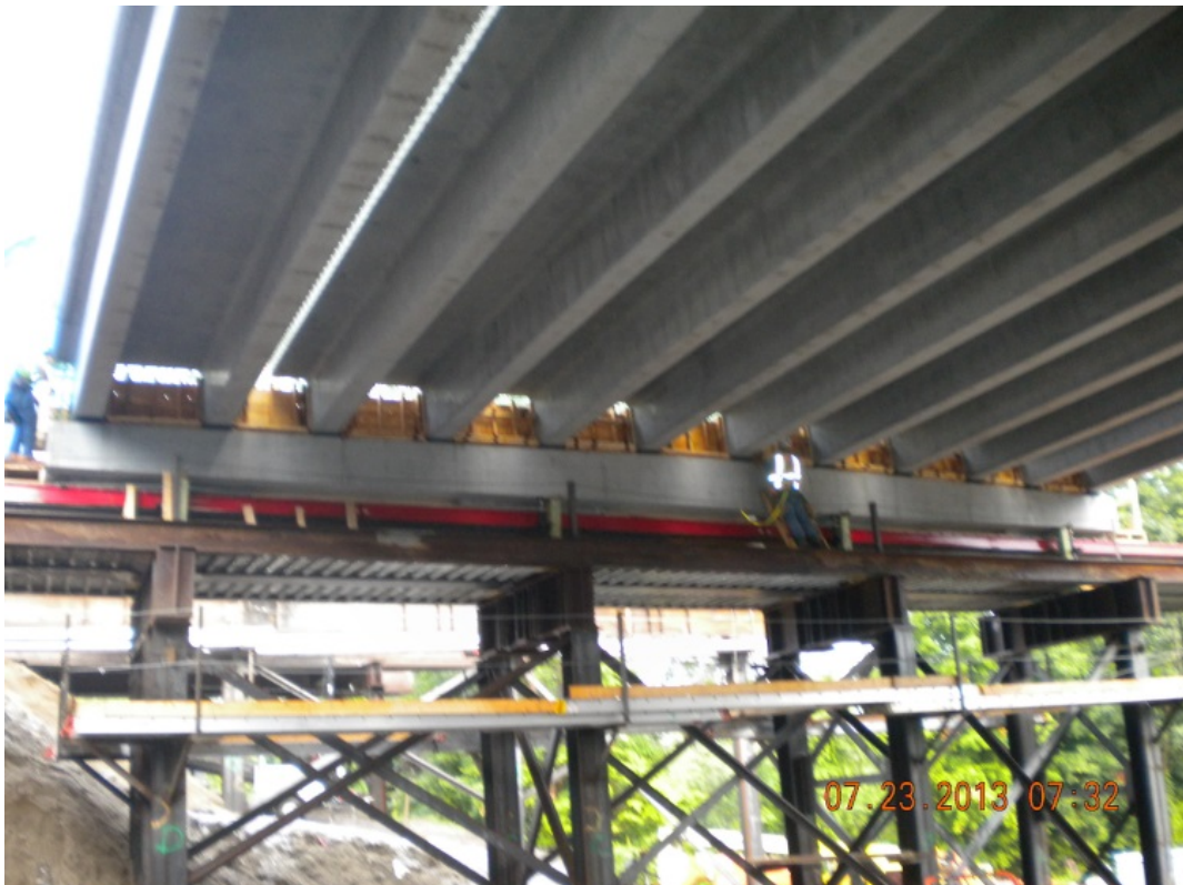
Figure 23. Photo. View of the superstructure from under the bridge.
