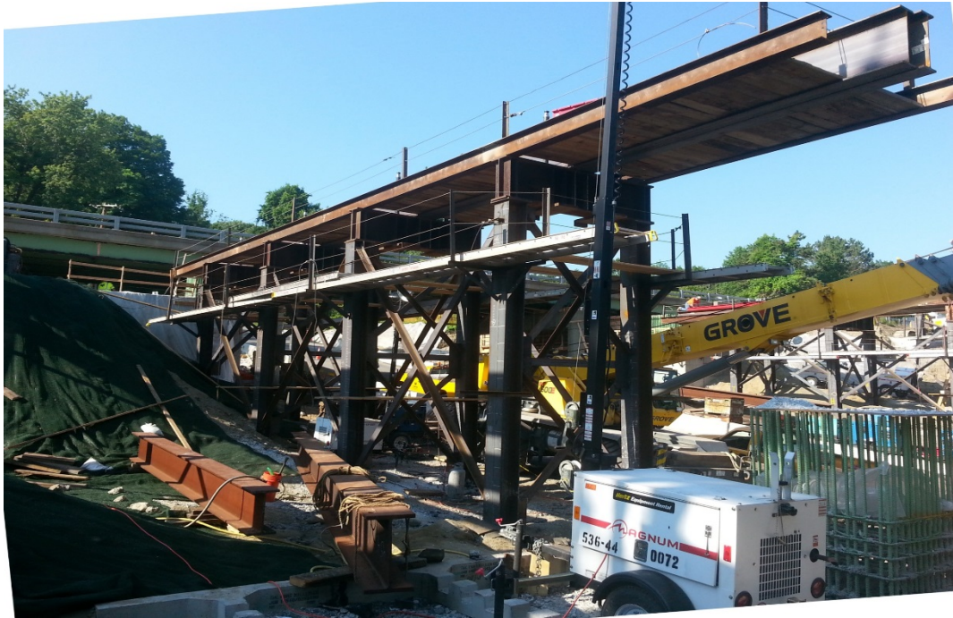
Figure 15. Photo. Construction of temporary bent nearing completion.
