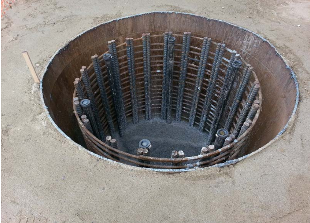
Figure 13. Photo. Drill shaft casing with reinforcement.
