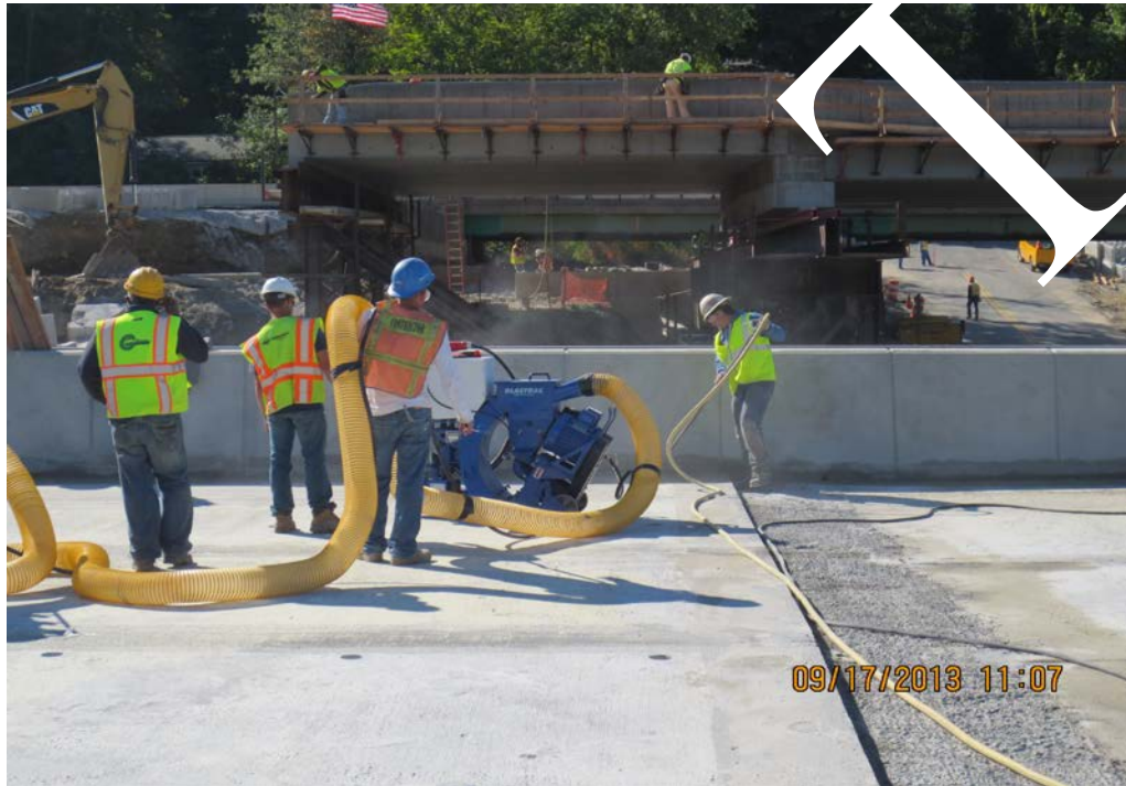
Figure 28. Photo. Blast cleaning deck surface.
