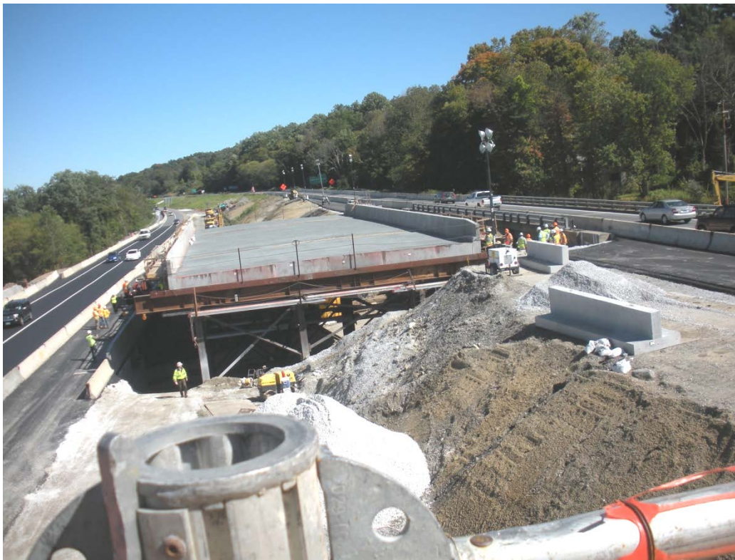
Figure 59. Photo. Showcase participants at job site.
