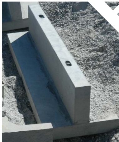
Figure 10. Photo. Typical precast sleeper slab element.
