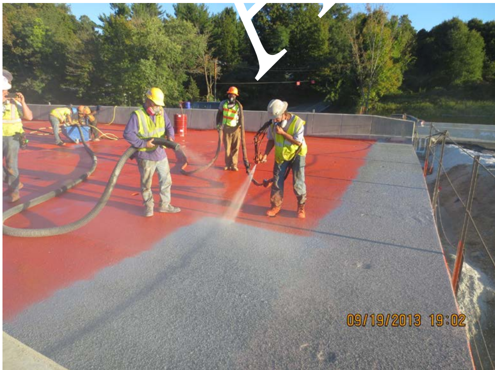
Figure 30. Photo. Placing the second layer of waterproofing membrane and fine aggregate.
