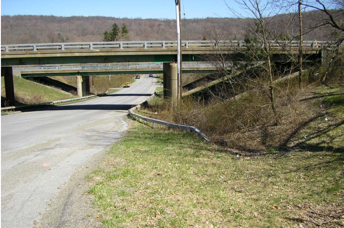
Figure 3. Photo. Original bridges over Dingle Ridge Road, showing elevation differential.
