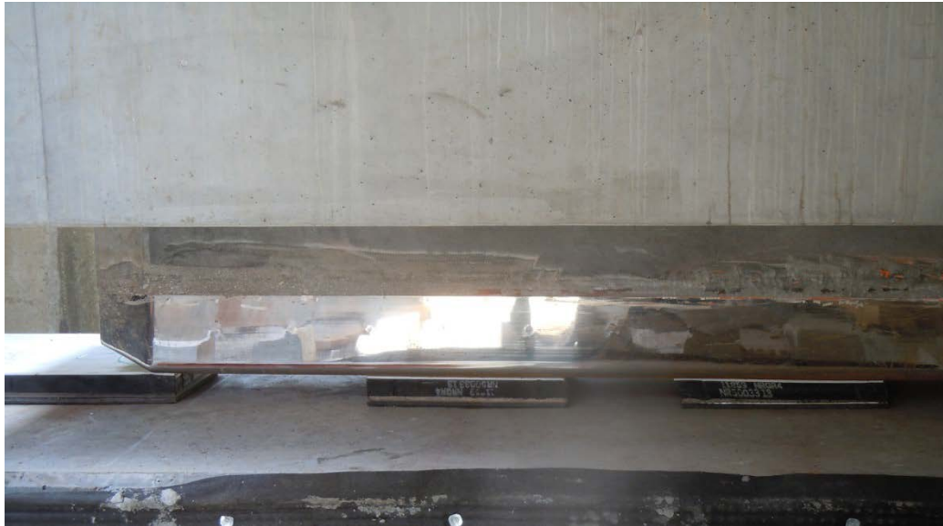
Figure 35. Photo. Close-up of stainless steel shoes sliding over PTFE bonded to elastomer pads.
