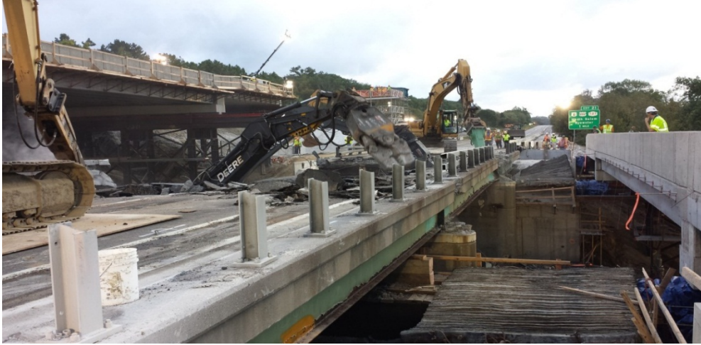
Figure 41. Photo. Demolition of the old structure.
