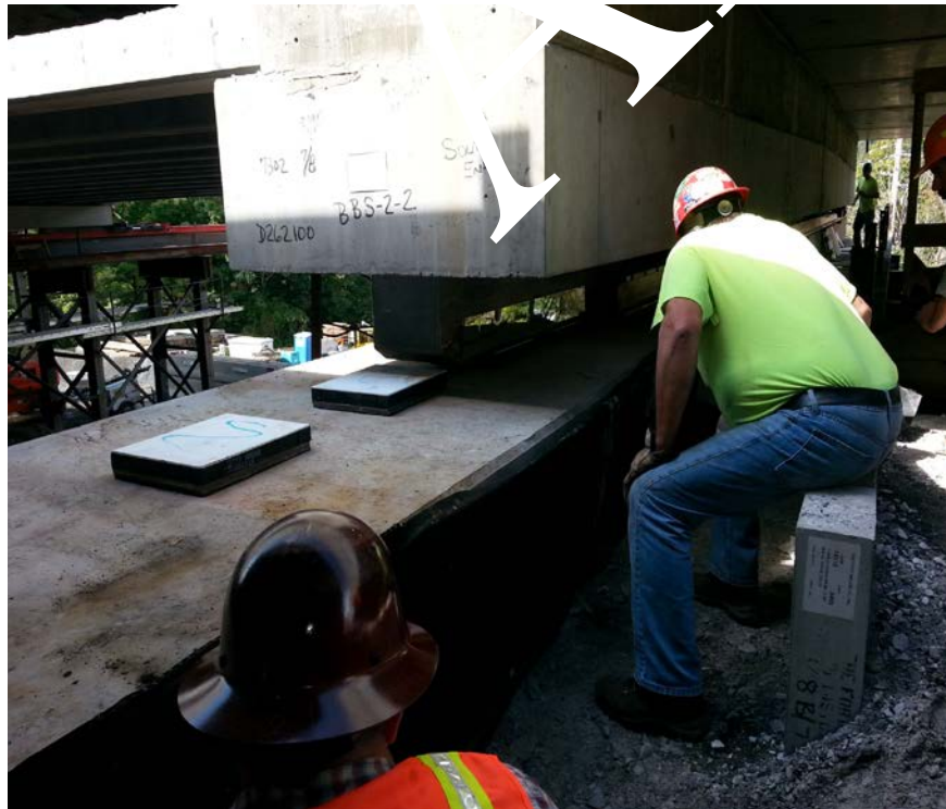
Figure 40. Photo. Monitoring of movement during trial slide.
