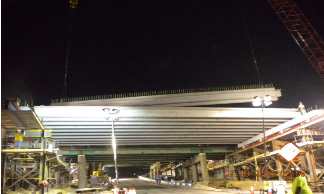
Figure 22. Photo. Near completion of NEXT beam placement.
