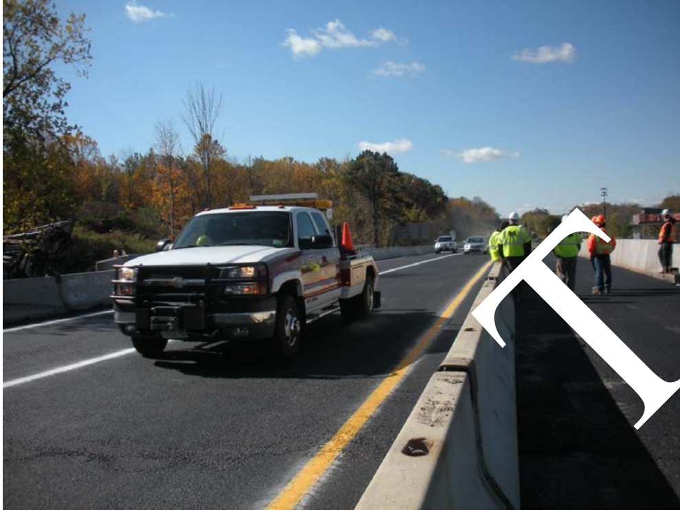
Figure 43. Photo. Bridge opened to traffic after line painting.
