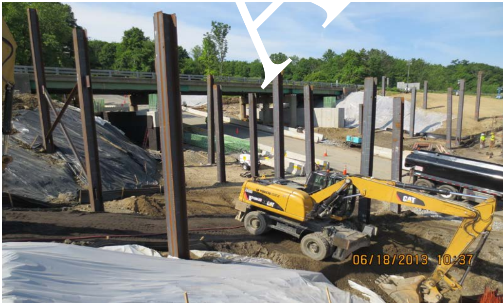
Figure 14. Photo. Construction of temporary bents, initial stage.
