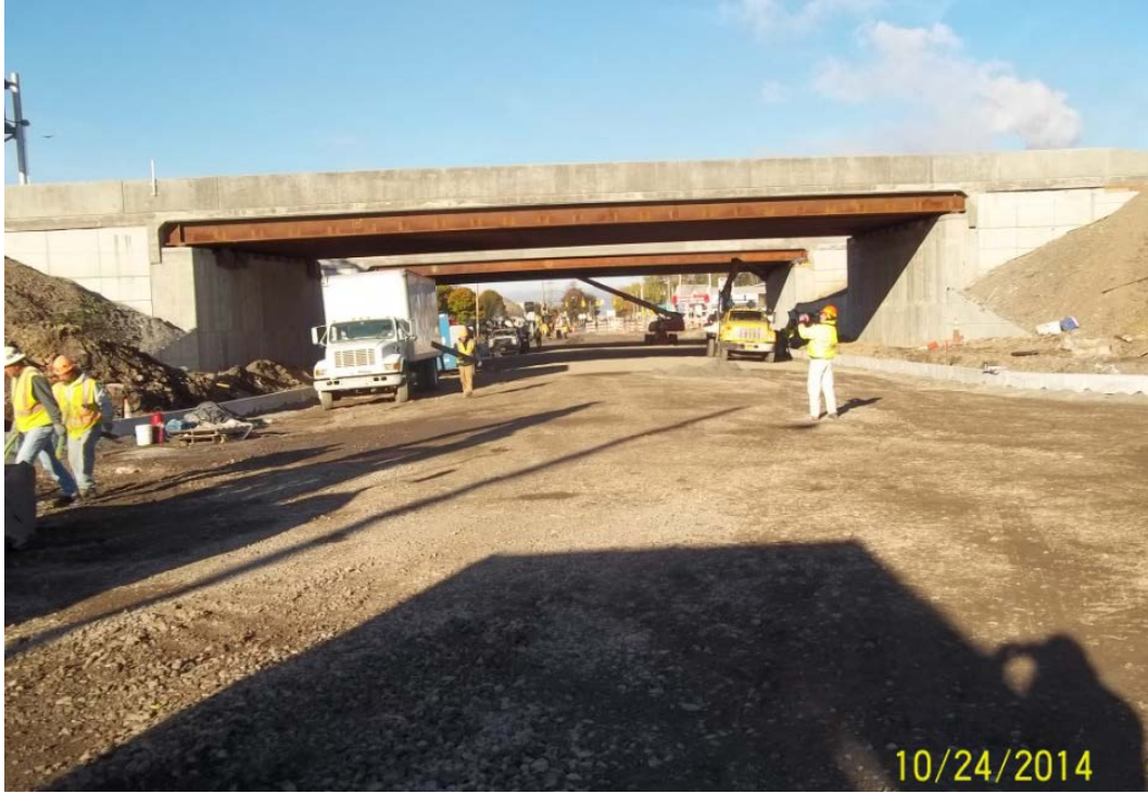
Figure 36. Photo. Buffalo Avenue reconstruction under the new bridges.
