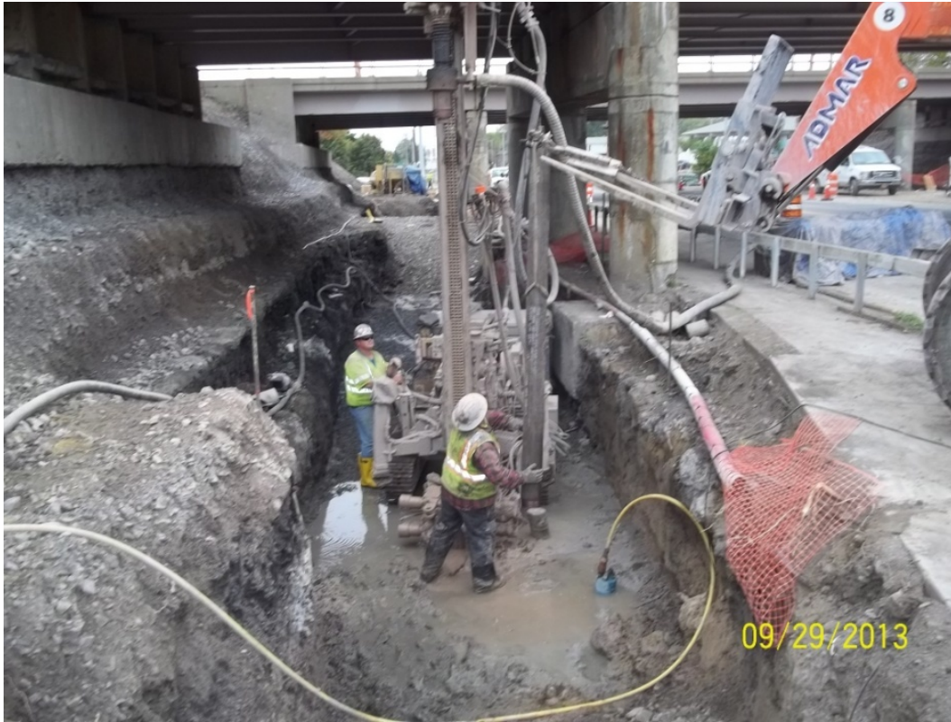
Figure 14. Photo. Installation of micropiles behind existing pier.
