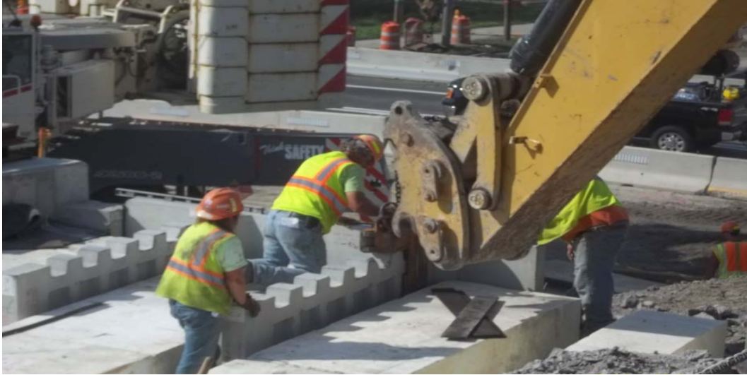
Figure 29. Photo. Modular T-wall construction and backfill installation.
