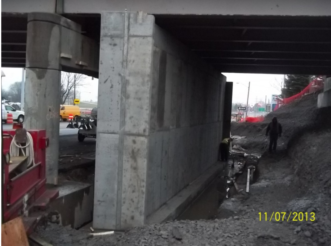
Figure 16. Photo. Completed abutment in place without backfill.
