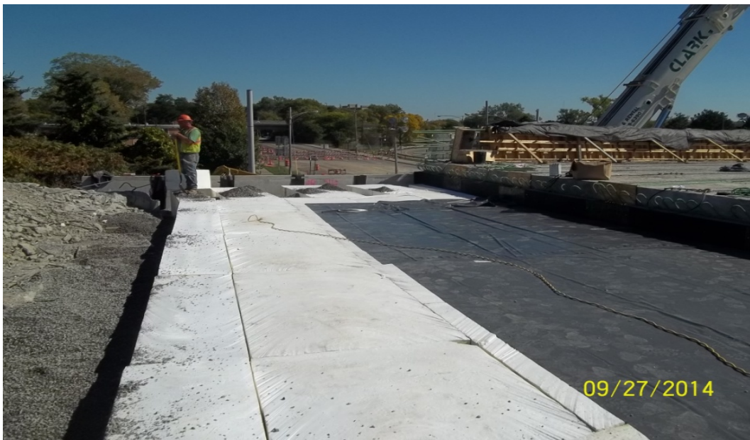
Figure 32. Photo. View of geo-membrane placed on top of abutment fill.
