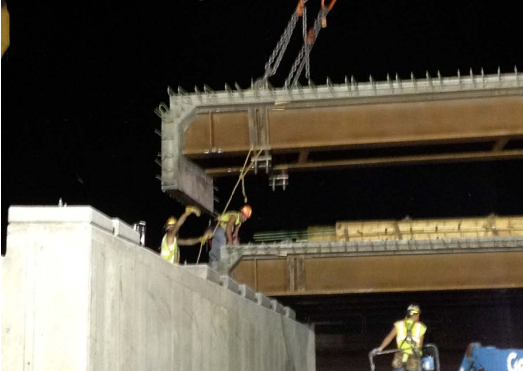
Figure 27. Photo. Modular deck units being installed.
