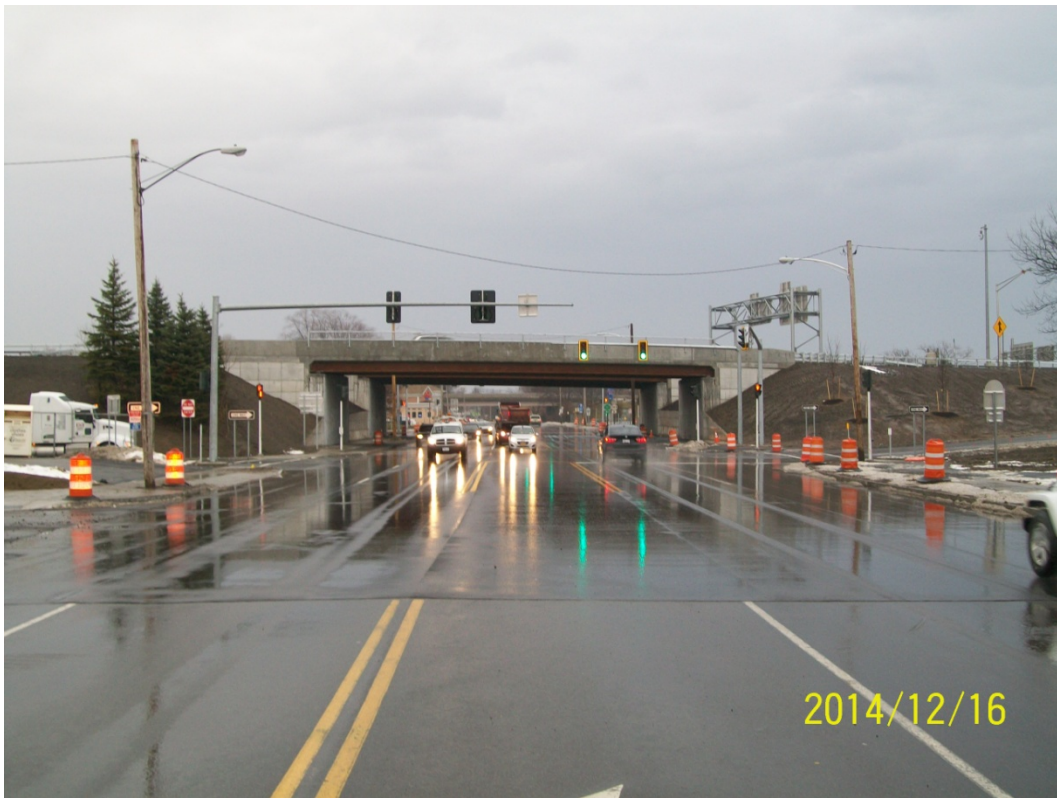
Figure 37. Photo. Completed Buffalo Avenue open to traffic.
