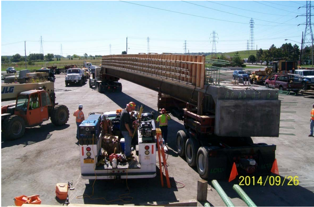
Figure 25. Photo. Loading of modular deck beam fascia unit.
