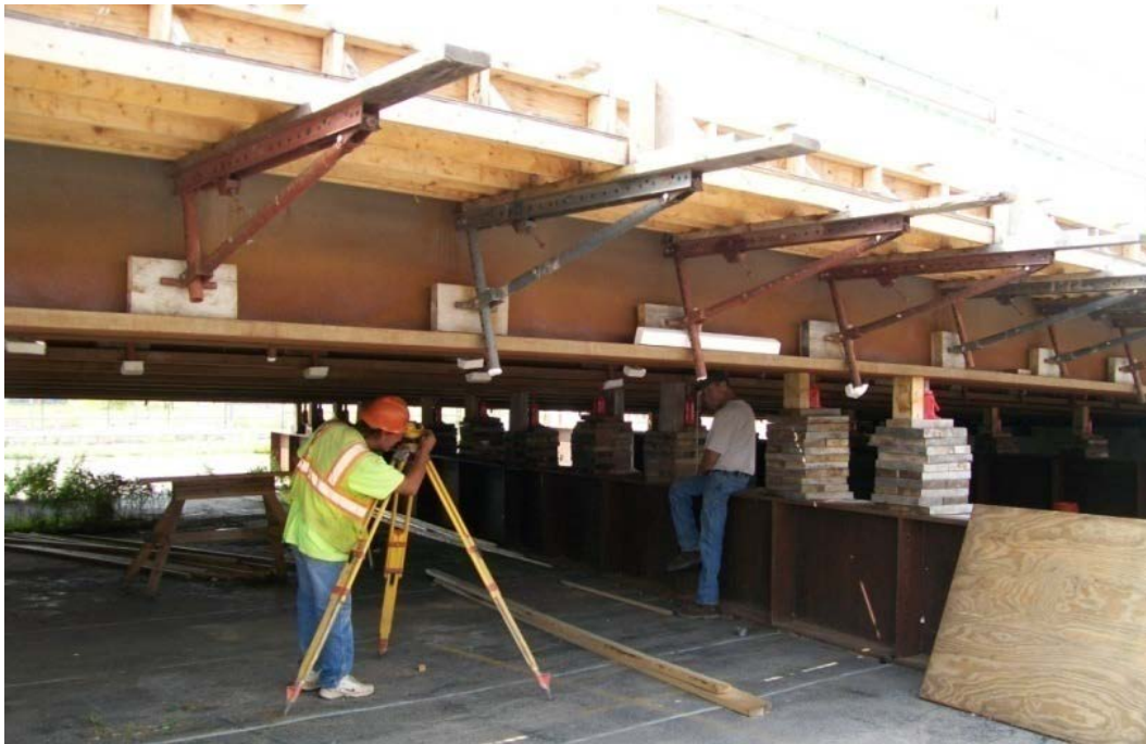
Figure 21. Photo. Making adjustments to cambers.
