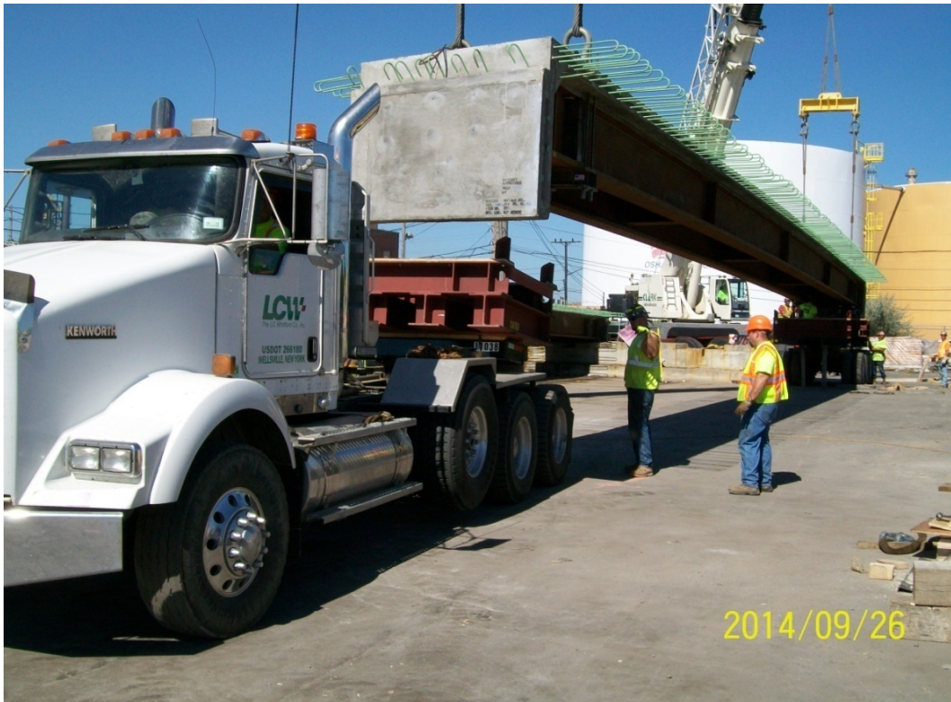
Figure 26. Photo. Loading of modular deck beam interior unit.
