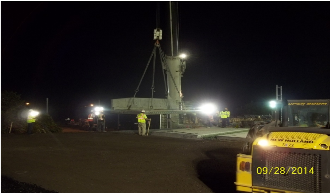
Figure 34. Photo. End approach slab unit installation.
