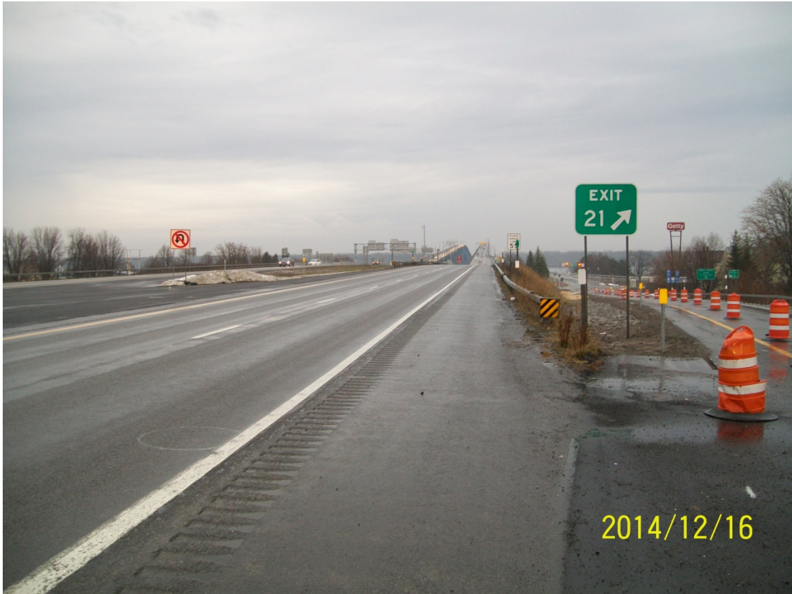
Figure 38. Photo. I-190 open to traffic
