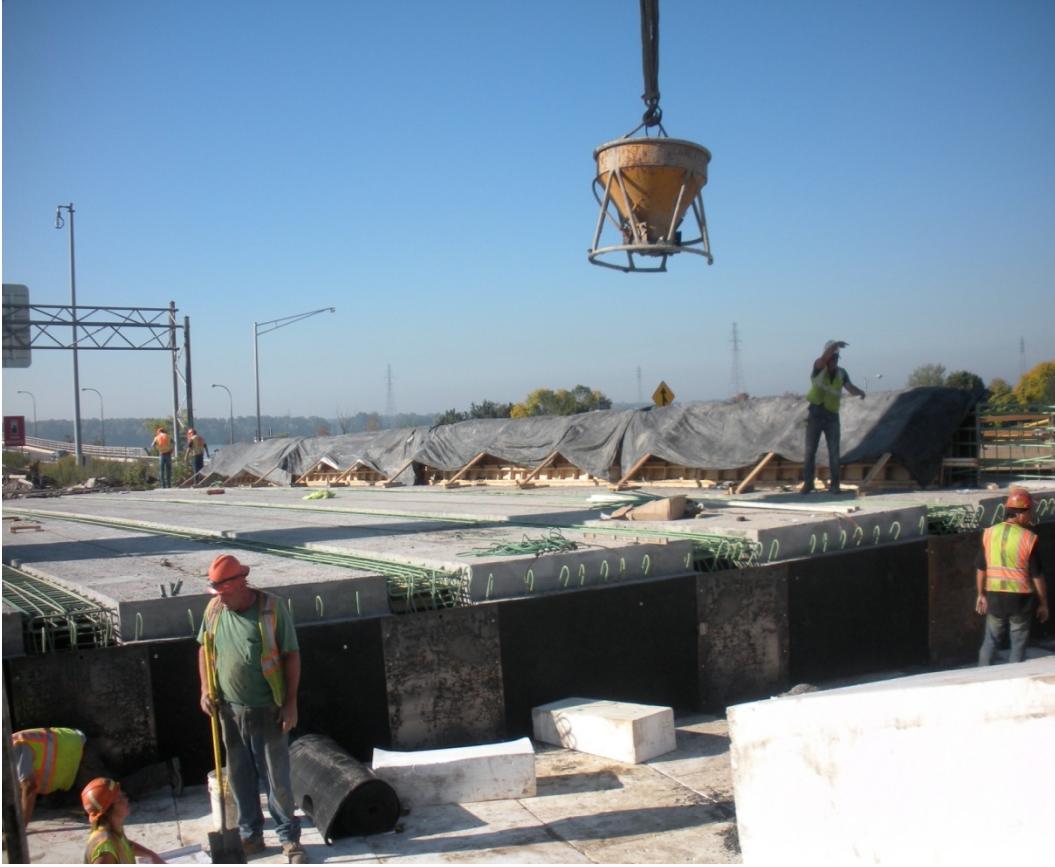
Figure 33. Photo. Deck closure pour in progress.
