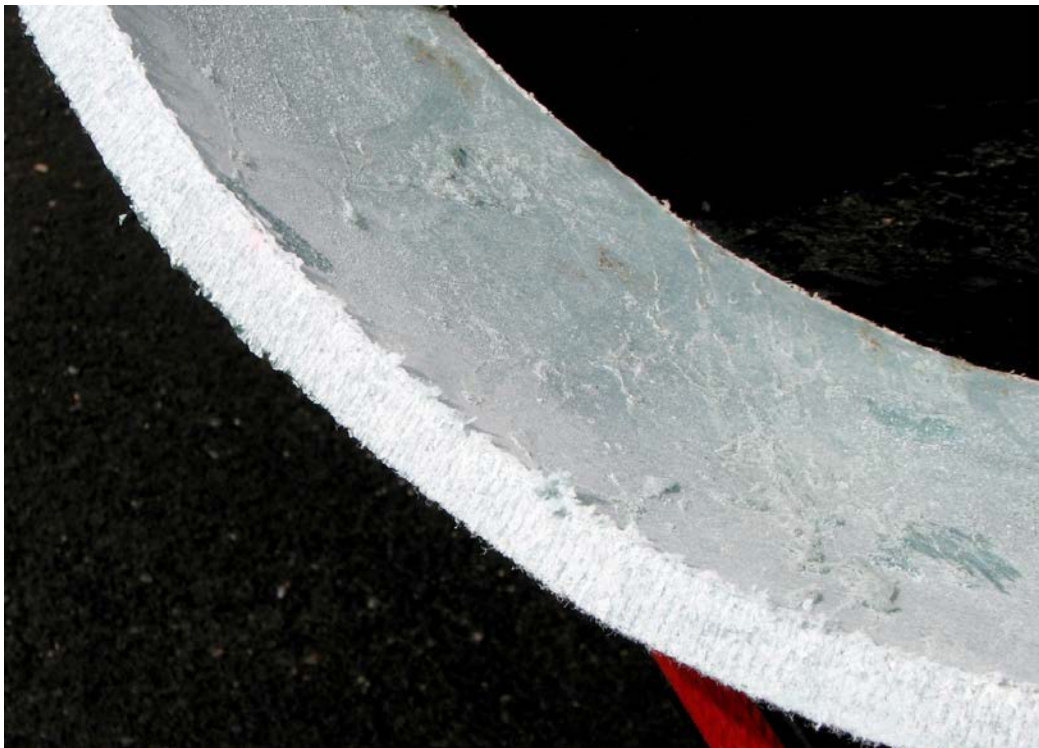
Figure 20. View of a fully cured CIPP.
