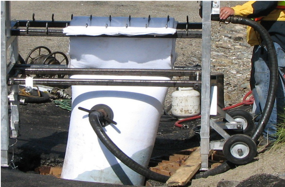
Figure 15. Closeup view of compressed air application and fully inverted liner.
