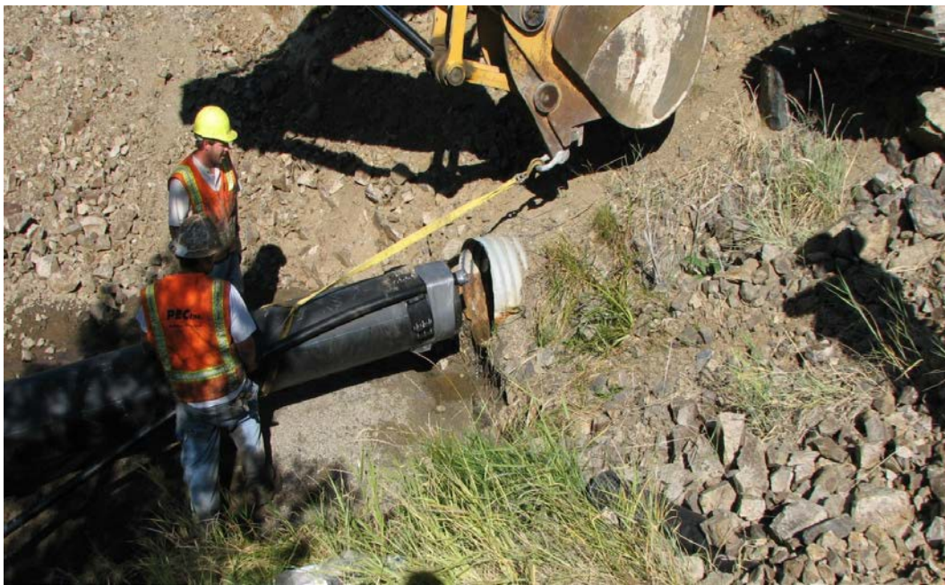
Figure 8. Pulling the liner and PVC tube into the existing pipe.
