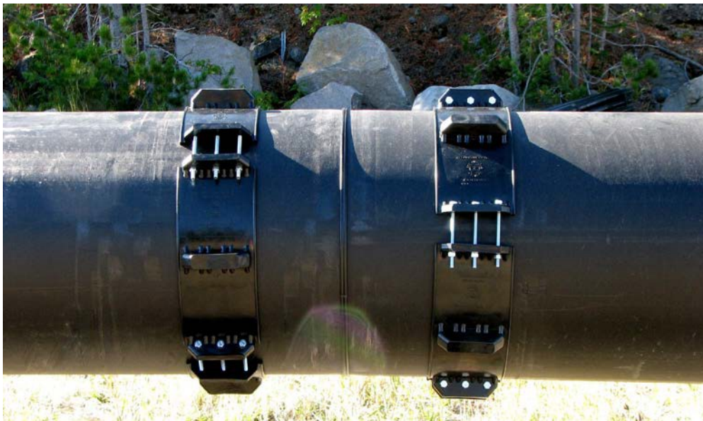
Figure 6. View of the welded pipes and spacers.
