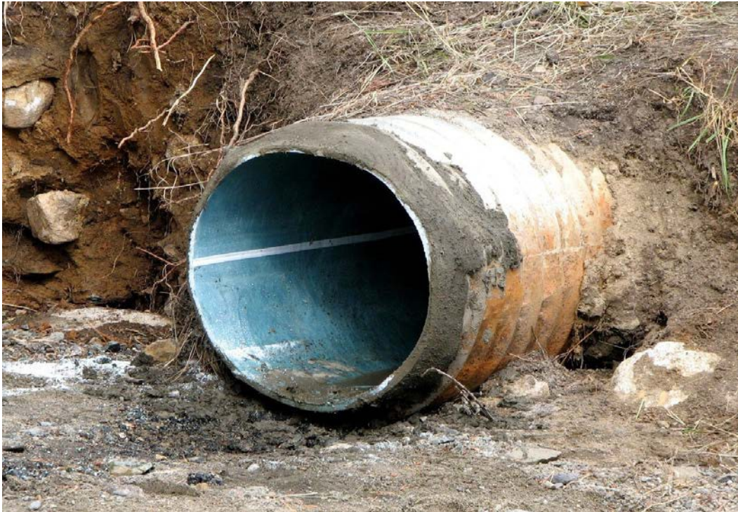
Figure 21. View of a fully installed CIPP liner ( Note intimate contact of the liner with the pipe).
