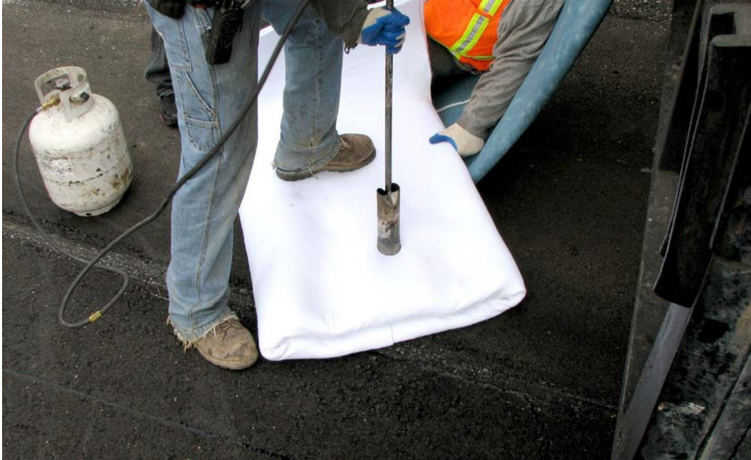
Figure 13. Inserting a circular hole into the liner using a heated core.
