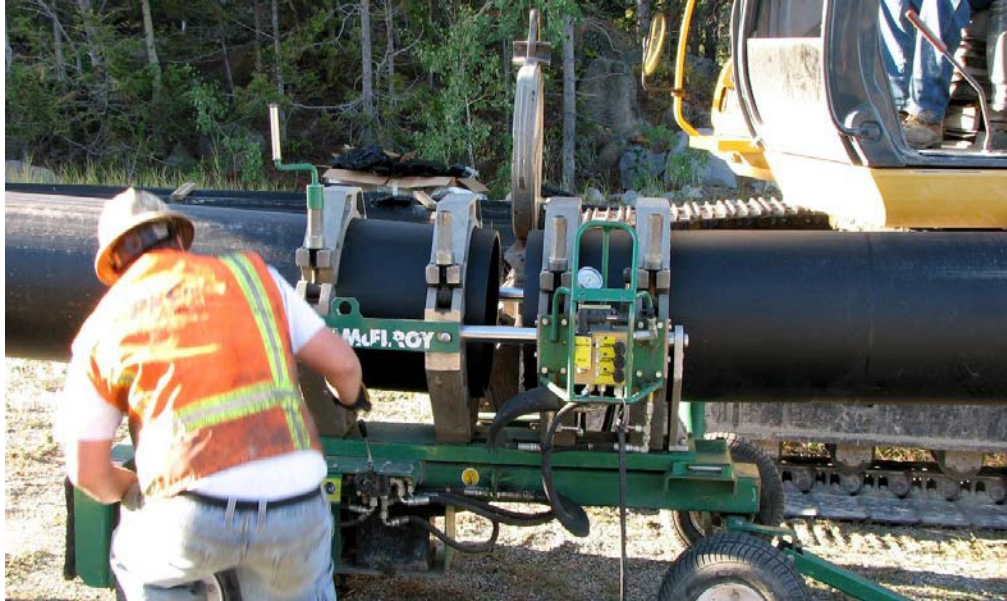
Figure 4. View of the pipe fuser apparatus.
