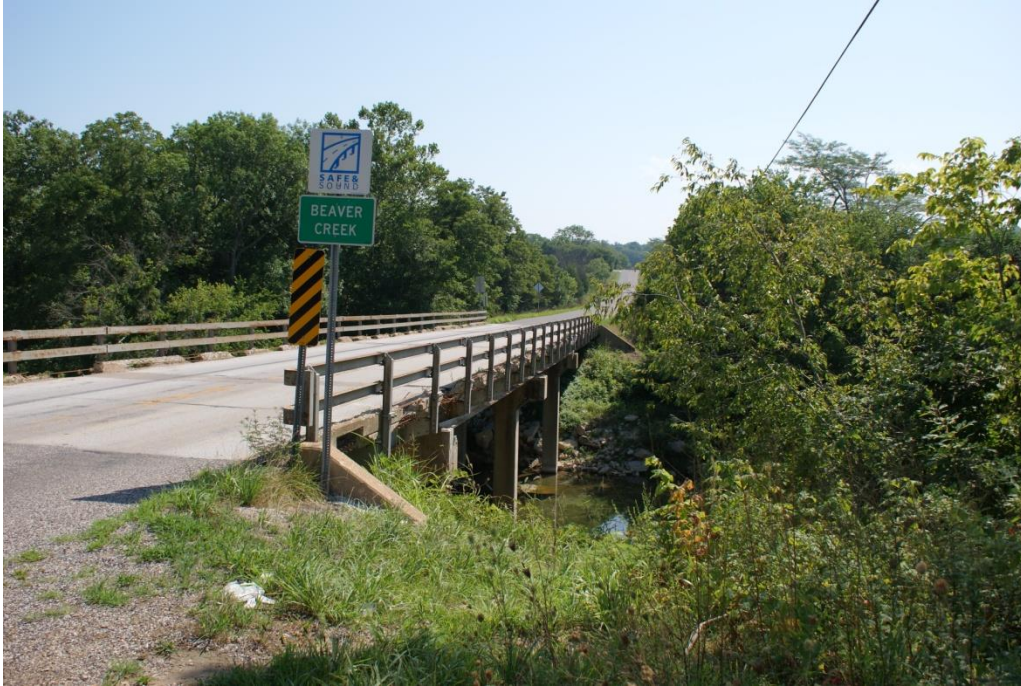
Figure 3. Old structure on MO 76 over Beaver Creek in Douglas County.
