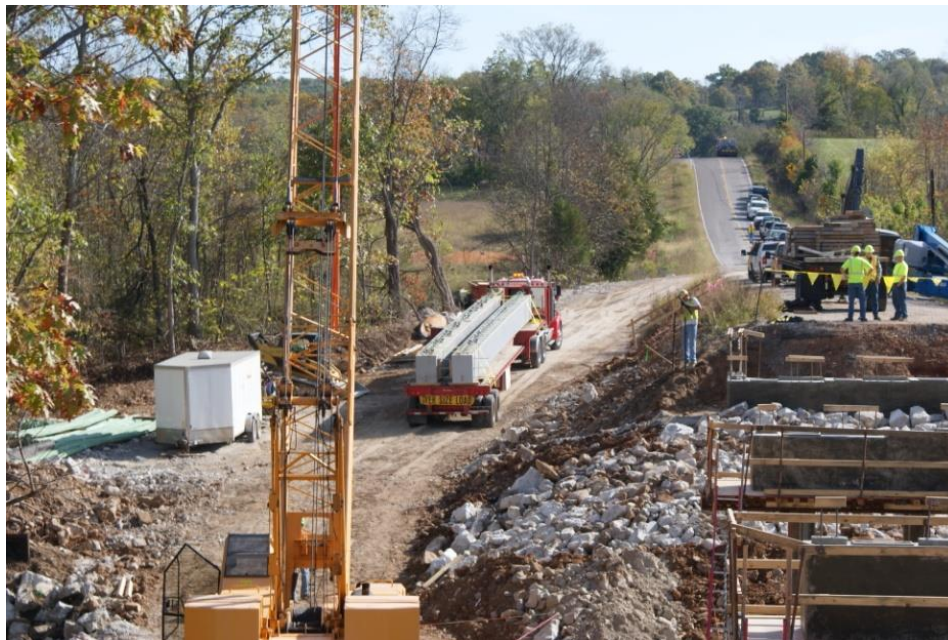
Figure 16. Delivery of beams to Douglas County project.
