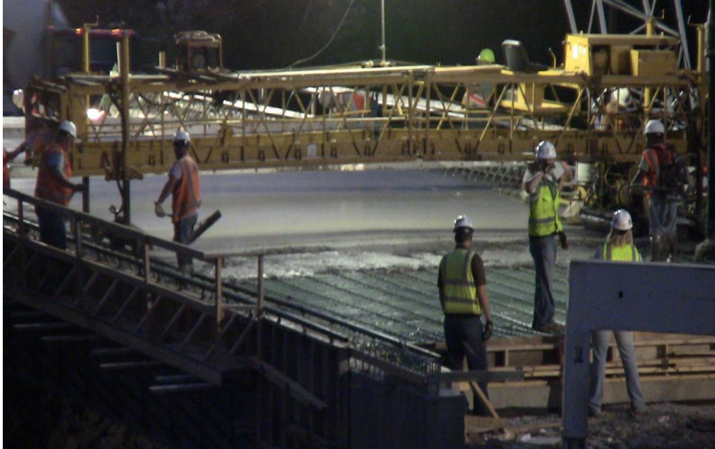
Figure 46. Deck placement on MO 97, Dade County.
