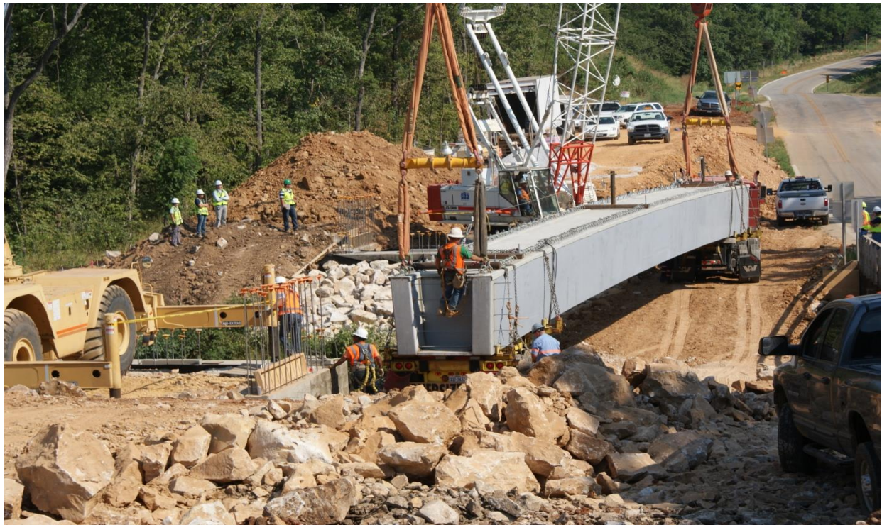
Figure 44. First beam attached to cranes for placement.
