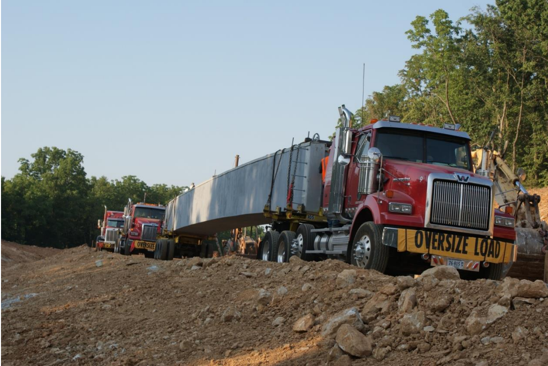
Figure 42. Beams lined up for installation.
