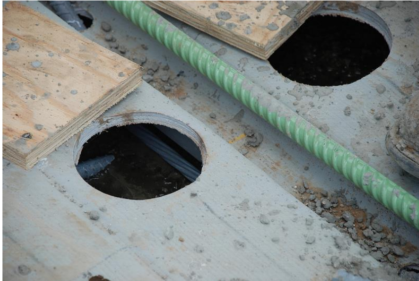
Figure 33. Original 4-in access holes for concrete introduction.
