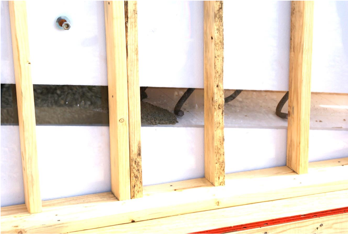
Figure 10. Self-consolidating concrete flowing through the beam arch around reinforcing steel.
