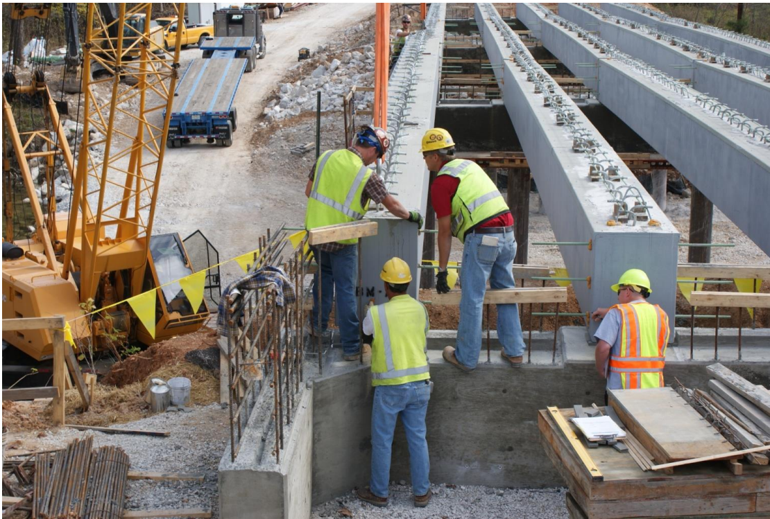
Figure 20. Final beam set in place.
