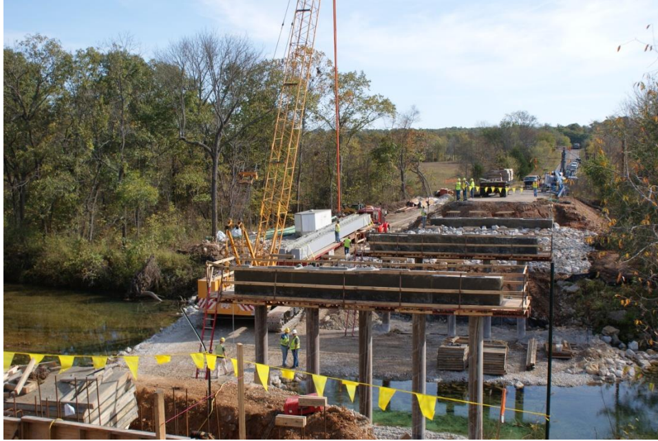
Figure 17. First beams arriving at the Douglas County site.
