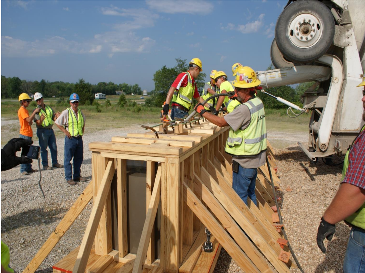
Figure 11. Vibrator being used to facilitate mix flow through beam arch.
