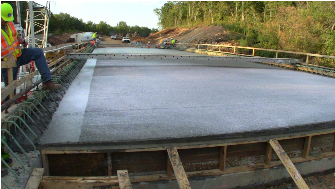
Figure 47. Completed deck on MO 97, Dade County.
