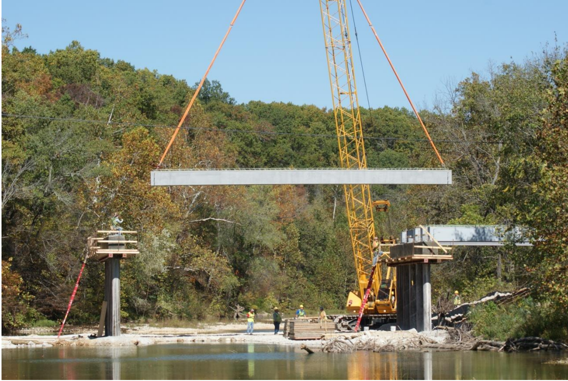
Figure 19. First center span beam lifted into position.
