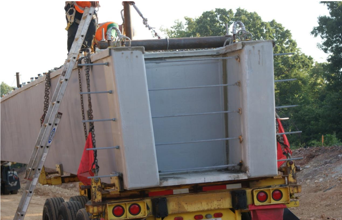
Figure 43. Beams are prepared for lifting into place. Note pipe bolted into place to accommodate lifting straps.
