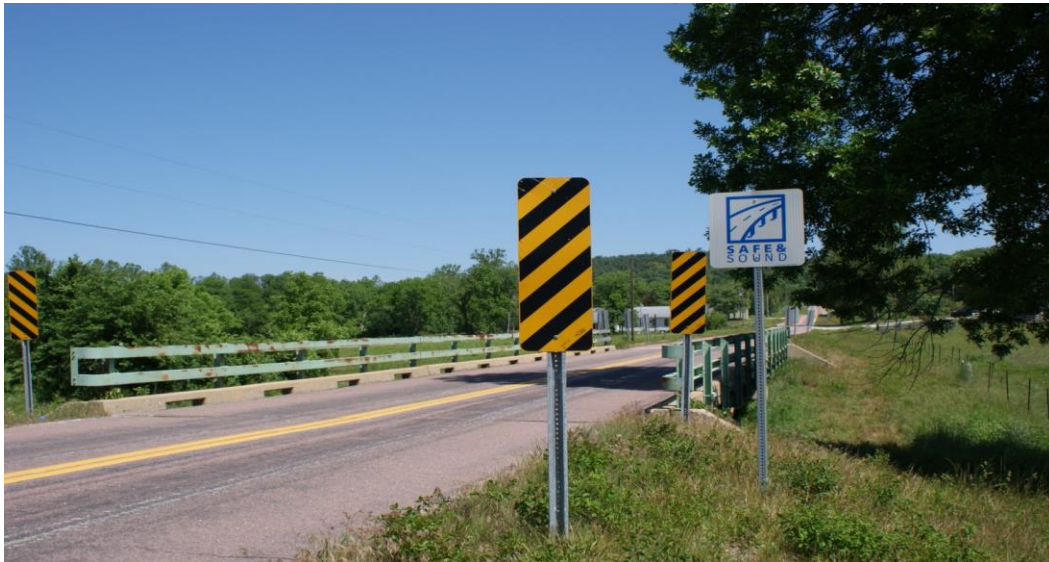
Figure 23. Existing structure on MO 49 over Ottery Creek Overflow in Reynolds County.
