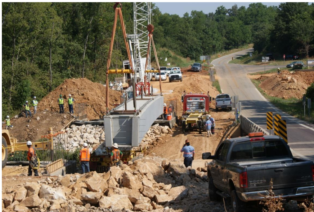
Figure 45. First beam moved into place.
