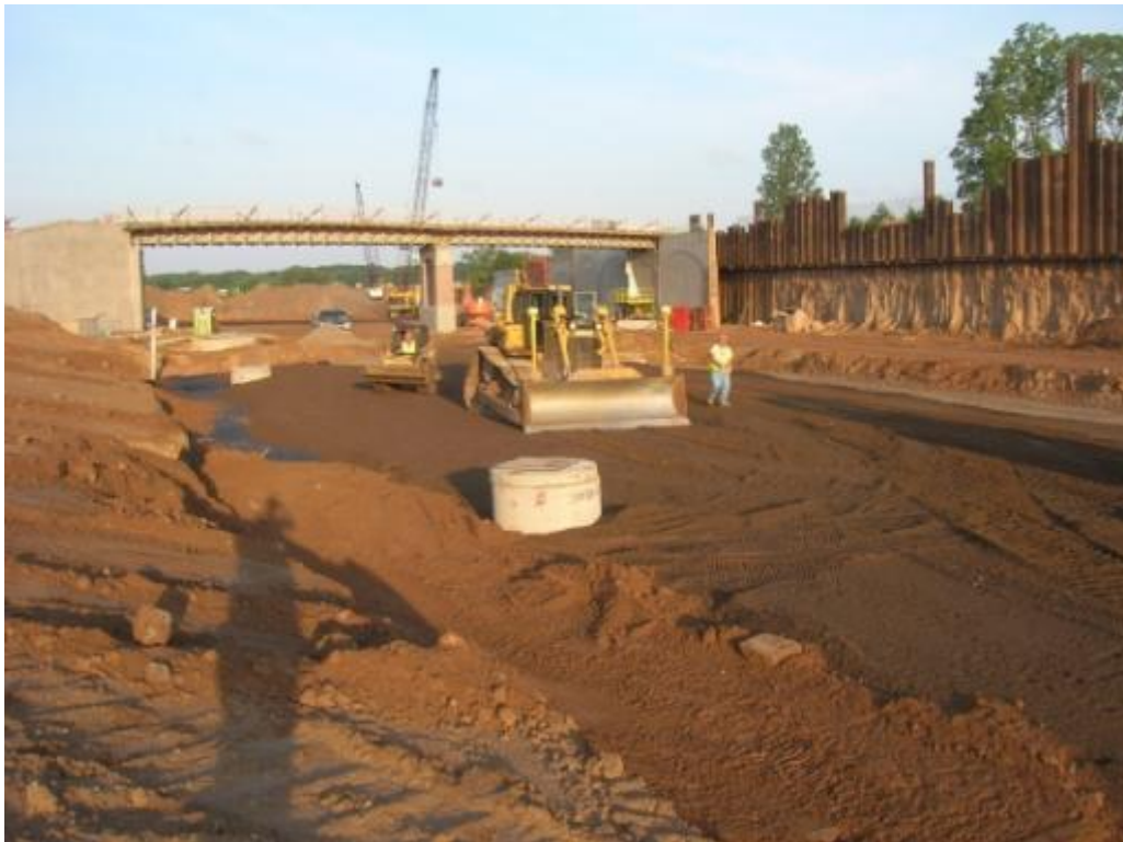
Figure 8. Pedestrian bridge under construction.
