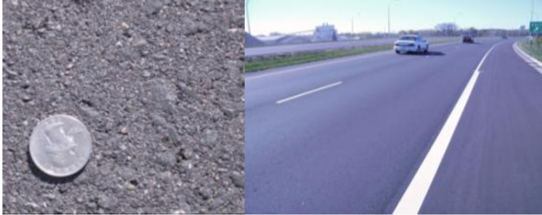
Figure 13. Newly constructed TH 36 HMA pavement.
