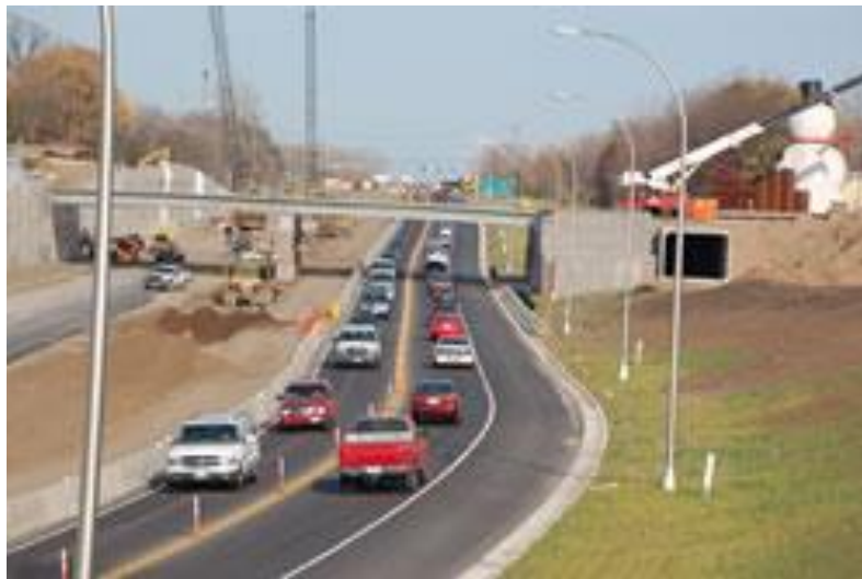
Figure 9. Eastbound lanes carrying head-to-head traffic. (Source: TERRA)
