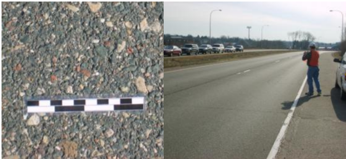
Figure 12. Existing TH 36 HMA pavement.
