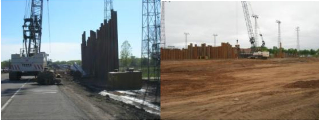
Figure 5. Shoring being placed along TH 36.
