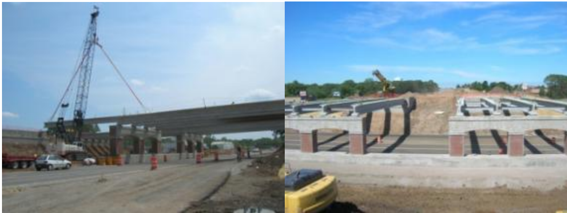
Figure 6. McKnight Road bridges under construction.
