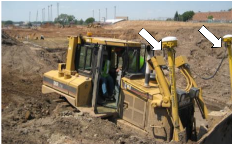
Figure 4. Bulldozer equipped with GPS receivers for grade control.
